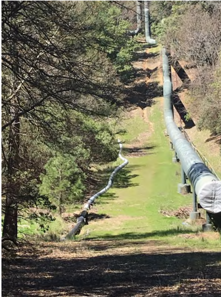
Injection Line Area
