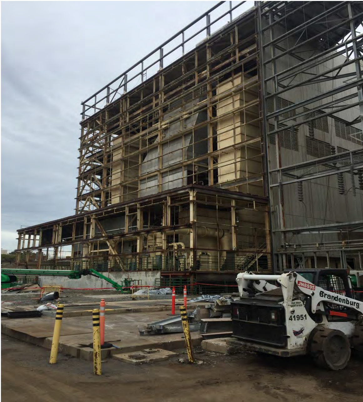
Photo #2: Encina East Wall transite panels removed, Transmission Bay structure on right.
