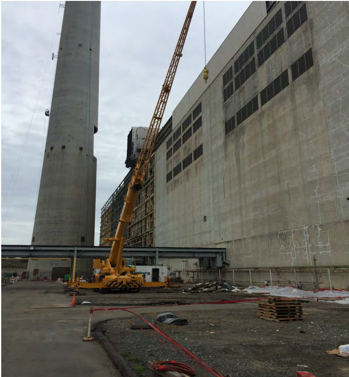
Photo #4: Encina East Wall Remaining Transite at North End Removal ongoing.
