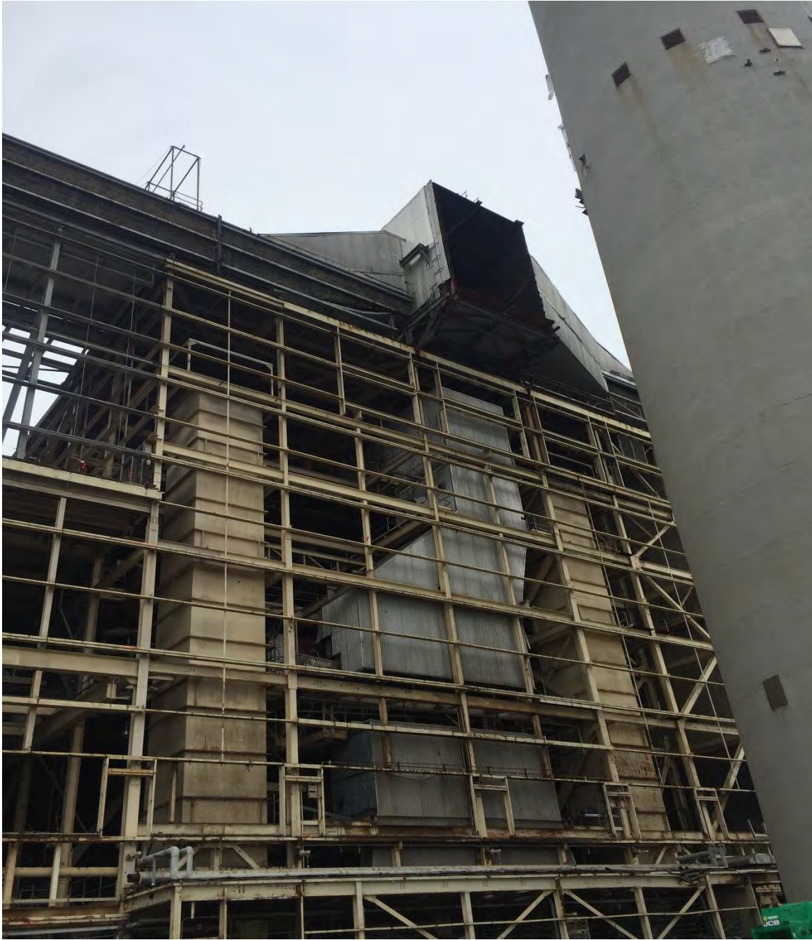
Photo #7: Encina East Wall Roof Demo “Peel Off” ongoing.
