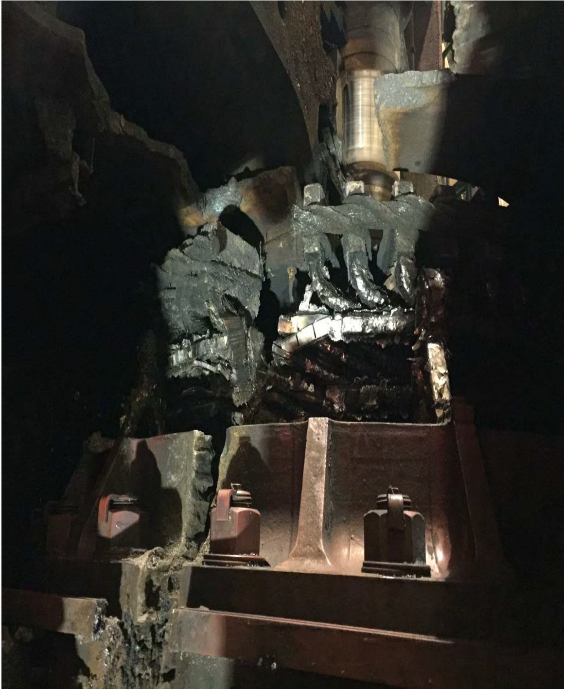
Photo #5: Encina Turbine #4 Mounting Feet remaining Turbine Structure Cut & Removed.
