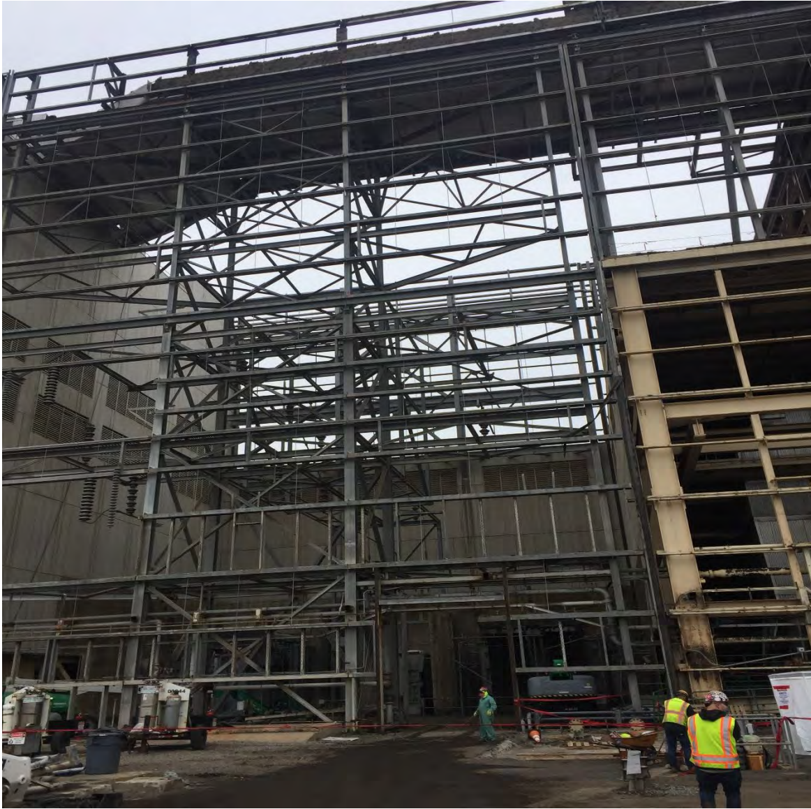
Photo #3: Encina East Transmission Bay Structural Steel Cut & Removed ongoing.
