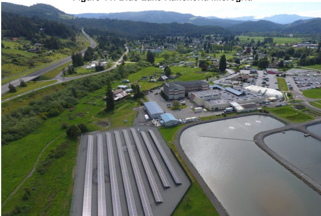
Figure 11: Blue Lake Rancheria Microgrid
