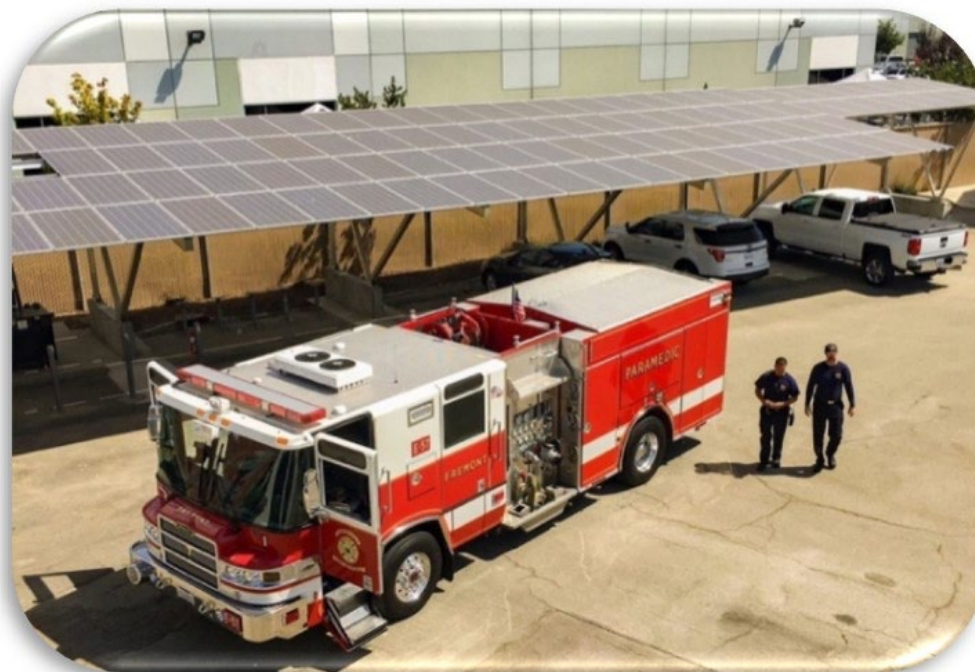
Figure 6: City of Fremont Fire Station Microgrid
