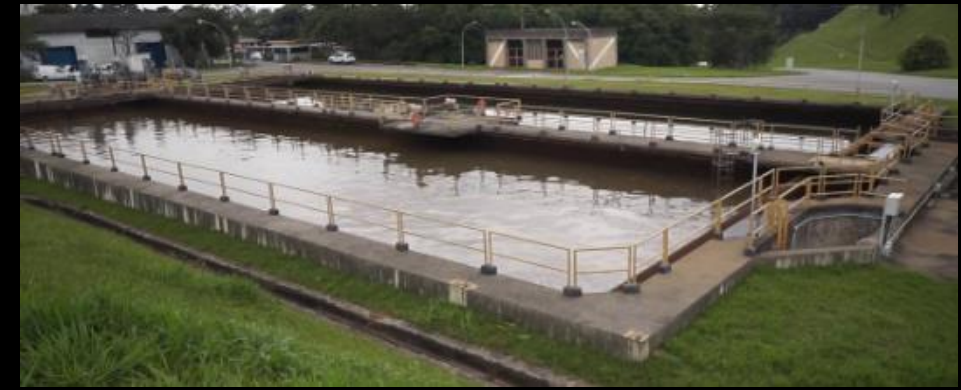
Equalization Tanks to Remove Smell
