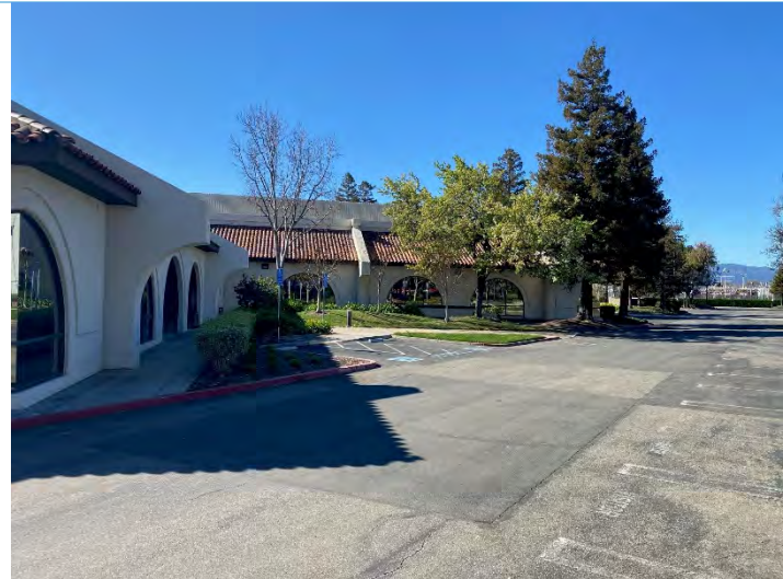
Photograph 8: Looking west along alley on north side of building (2/24/21).
