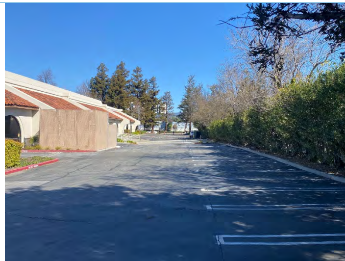
Photograph 16: Looking northeast along alley on southeast side of the building (2/24/21).
