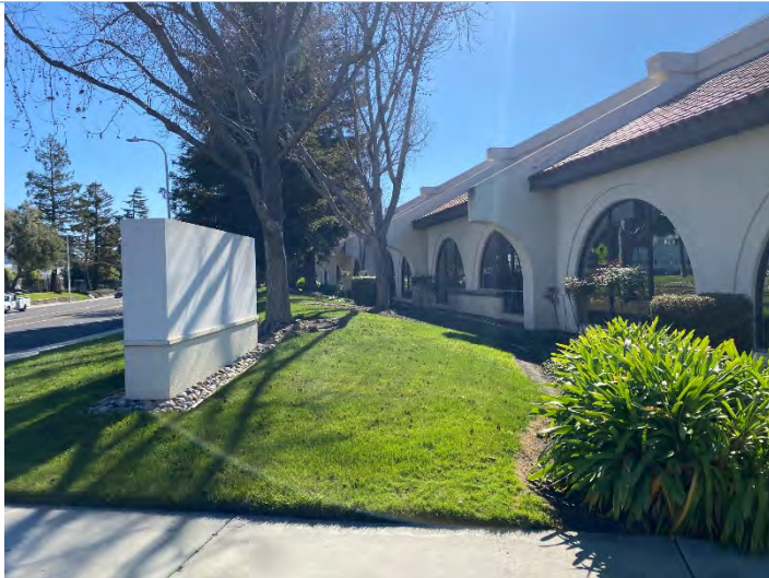
Photograph 7: Looking southeast along Walsh Avenue (2/24/21).
