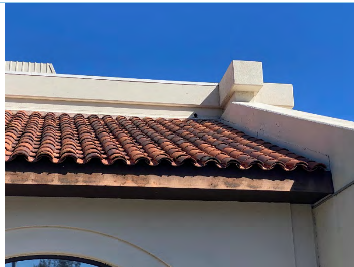
Photograph 14: Typical terra cotta type roof style (2/24/21).
