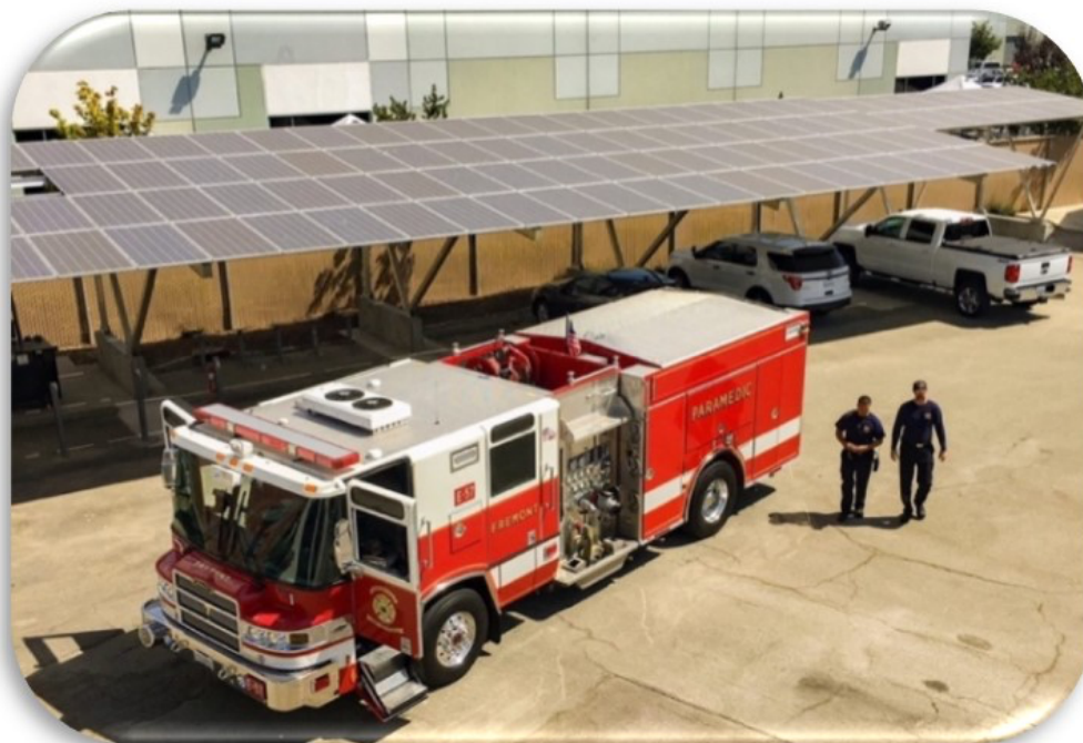
Figure 6: City of Fremont Fire Station Microgrid
