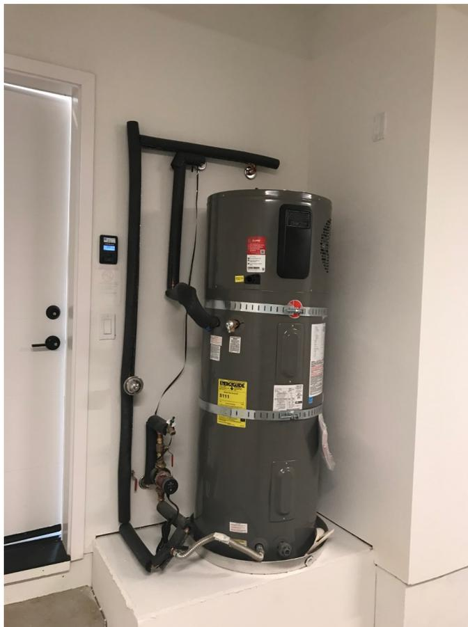
**Plan 1's tanked electric water heater element in the garage of a Round Barn townhouse model. The associated shared, heat pump, is mounted on the rooftop to minimize loss of 100-sqaure feet of garage space [3].**
