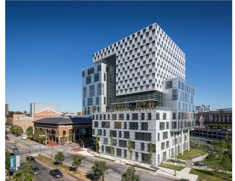
“The facade and atrium design led to passive and active strategies that typically aren't applied in this climate. The building's passive design strategies achieve very high performance and flexibility without the use of PV or solar thermal systems.”
