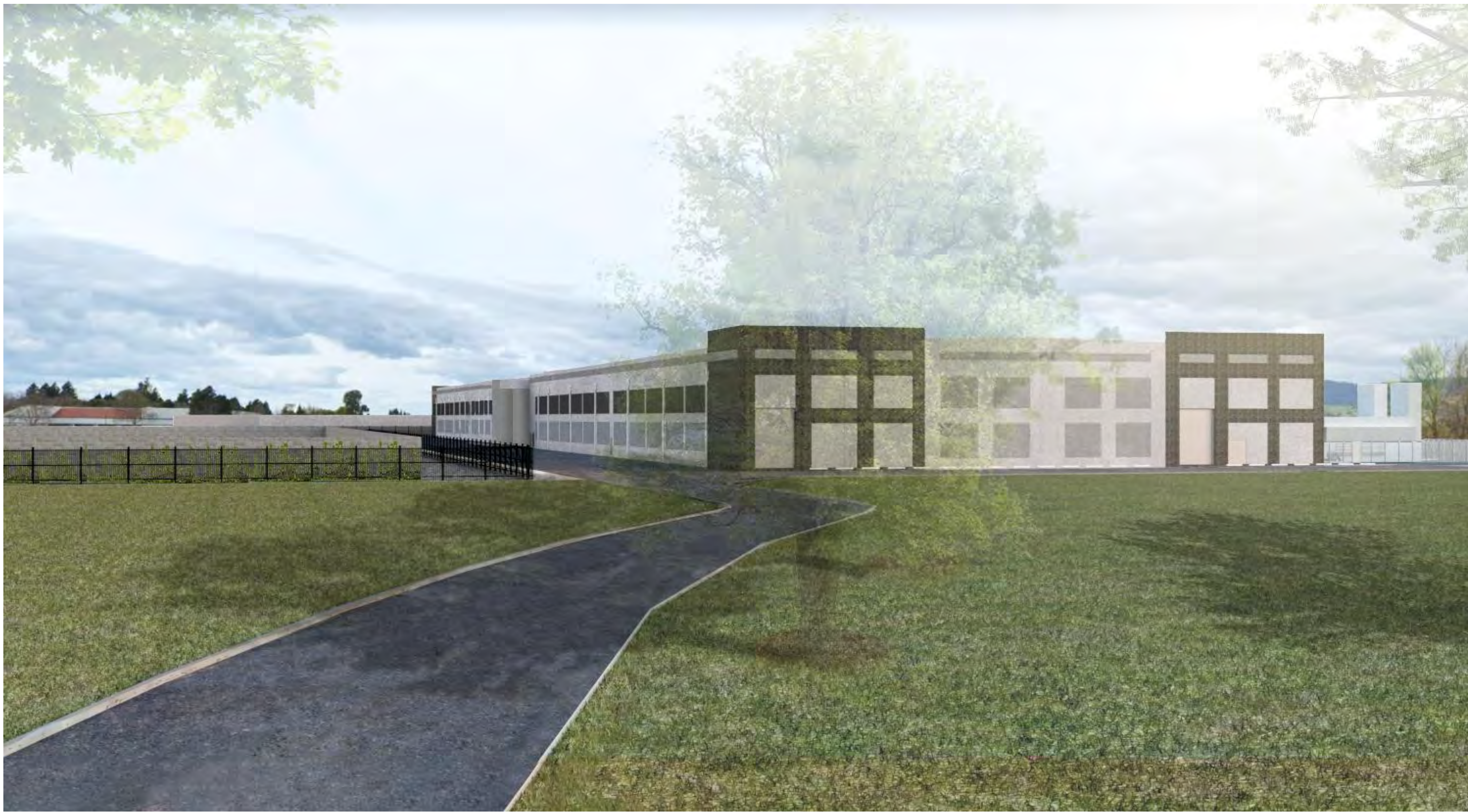
1. Southern Entry Roundabout View
