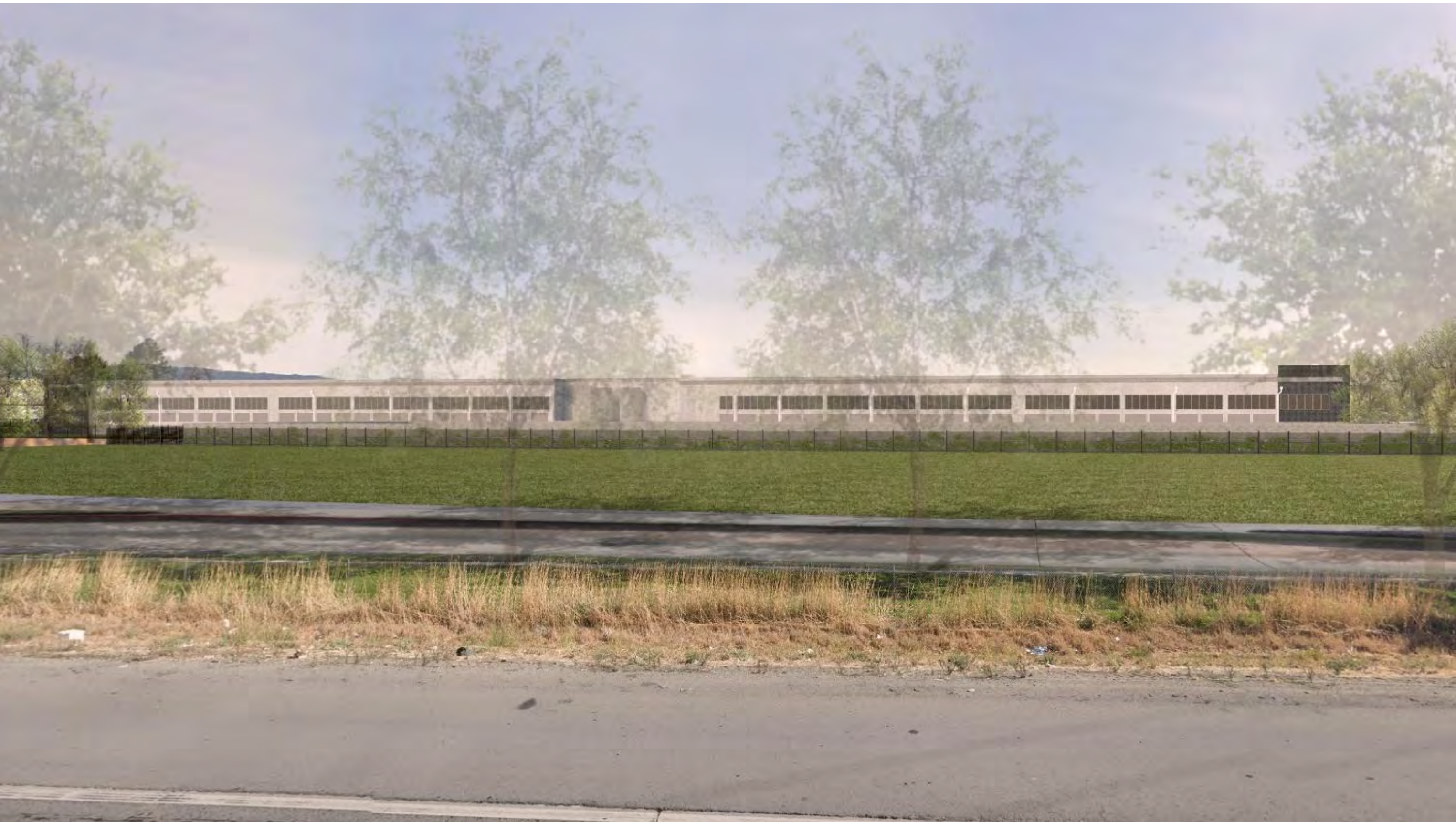
2. South Valley Freeway View
