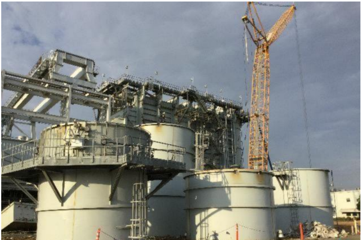
Cut parts of the stack from Unit 1.
