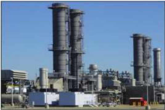
Two LMS100 Gas Turbine Generators with Encased Clutches at LADWP's Haynes Power Station, Long Beach, CA
