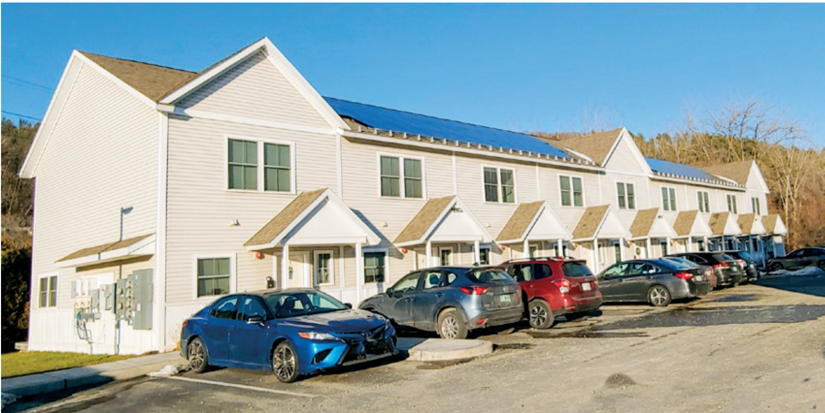
Multi-unit apartment building with solar panels in Vermont.
