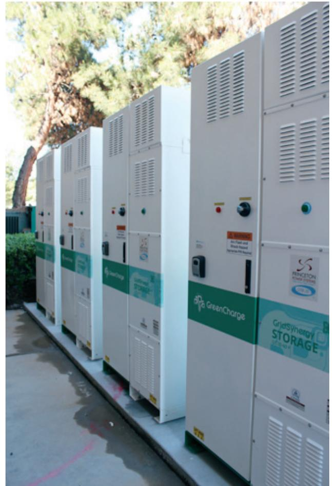
Battery systems in the 100 kilowatt-hour to 500 kilowatt-hour range, such as this system at a Safeway supermarket in San Jose, CA, typically cost less than smaller systems, around the \$600 to \$800 per kilowatt-hour range.
