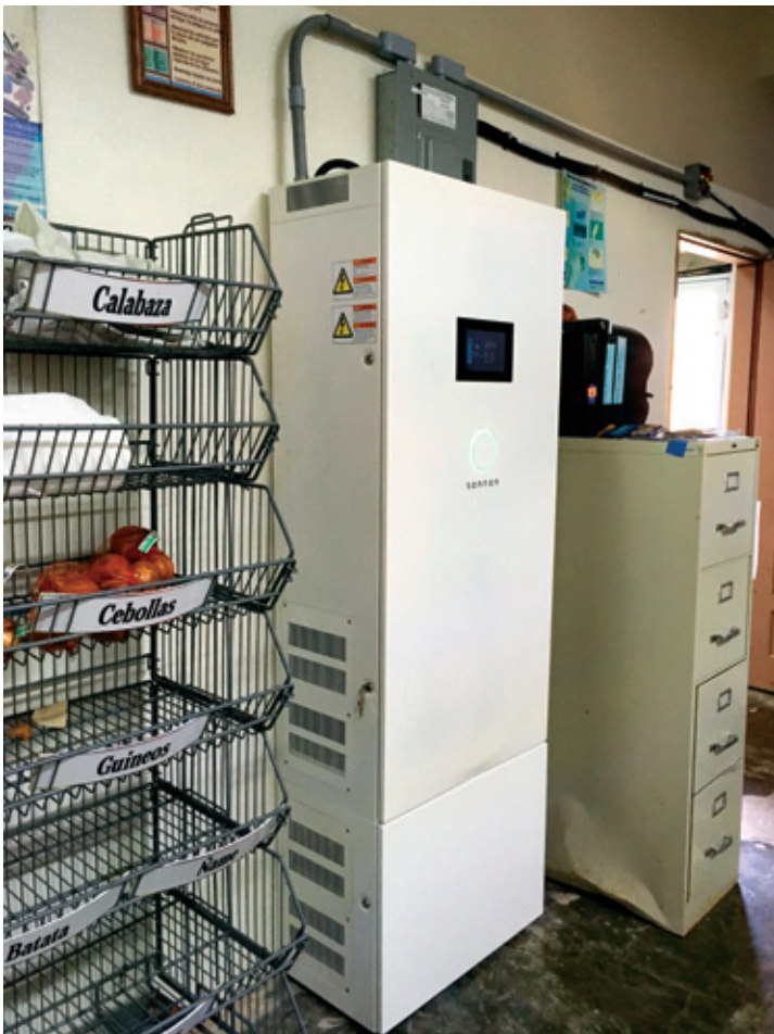
Residential and small commercial battery systems, like this 14-kilowatt-hour sonnen eco 14 battery at a remote school in Orcovis, Puerto Rico, tend to have an average installed cost between $800 to $1,000 per kilowatt-hour.
