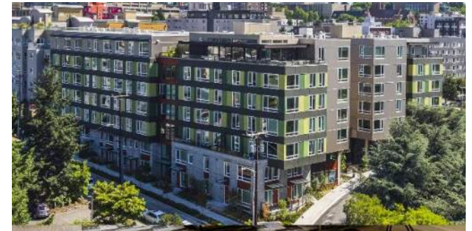
August Apartments, Seattle
