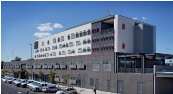
SMUD Office & Operations Building, Sacramento
