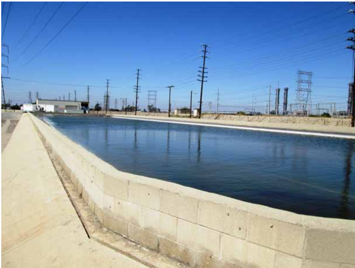
South Retention Basin, view looking northeast
