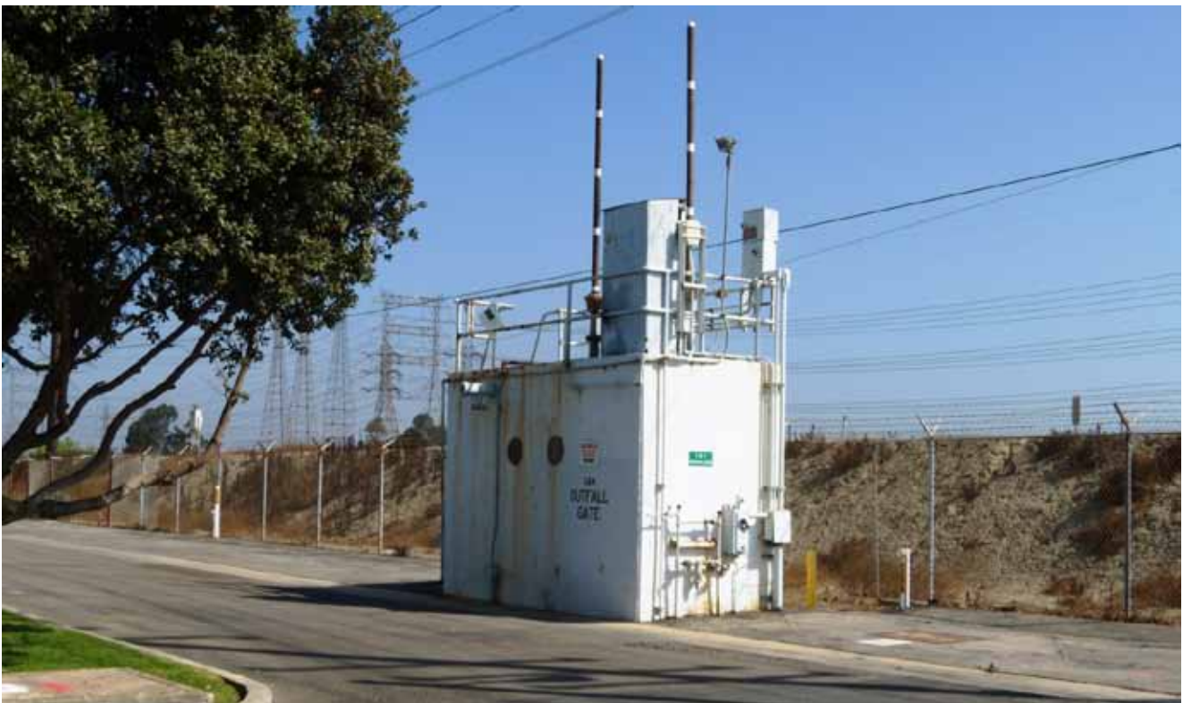
Units 3 and 4 Outfall Gate, view looking northeast.
