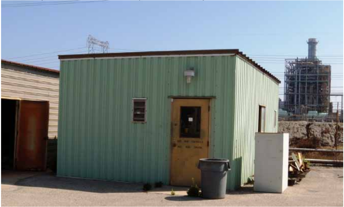
Mud Controls Building for Units 5 and 6, view looking northeast
