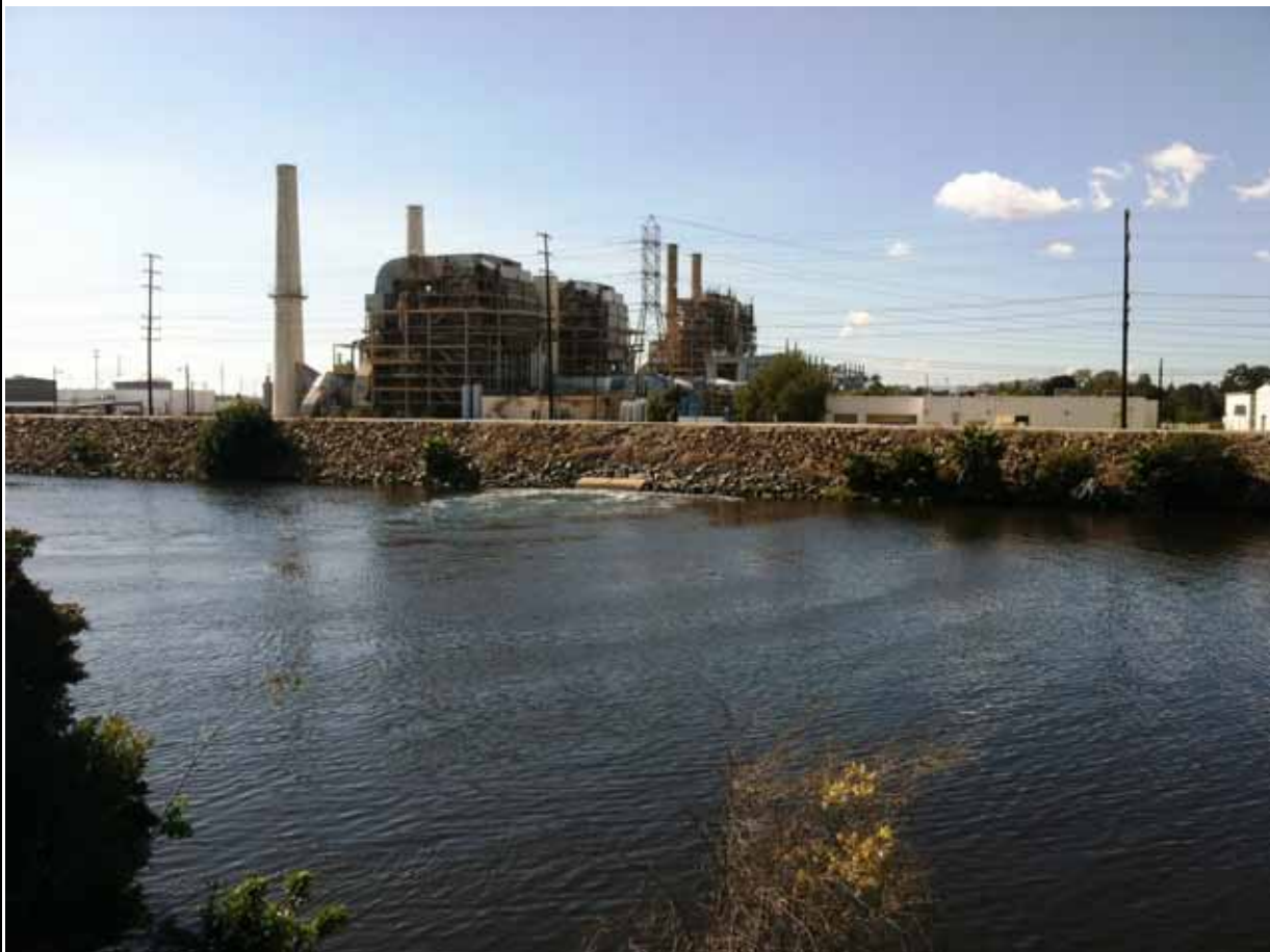
View looking southwest at AES Alamitos outfall for units 1 & 2 and east side of west bank levee. February 2014.
