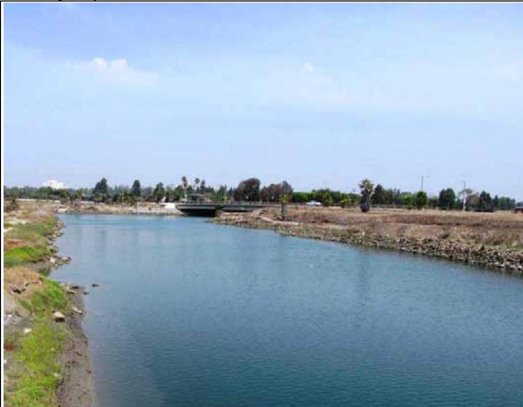
Los Cerritos Channel, view looking northeast towards Loynes Drive bridge. July 2013.
