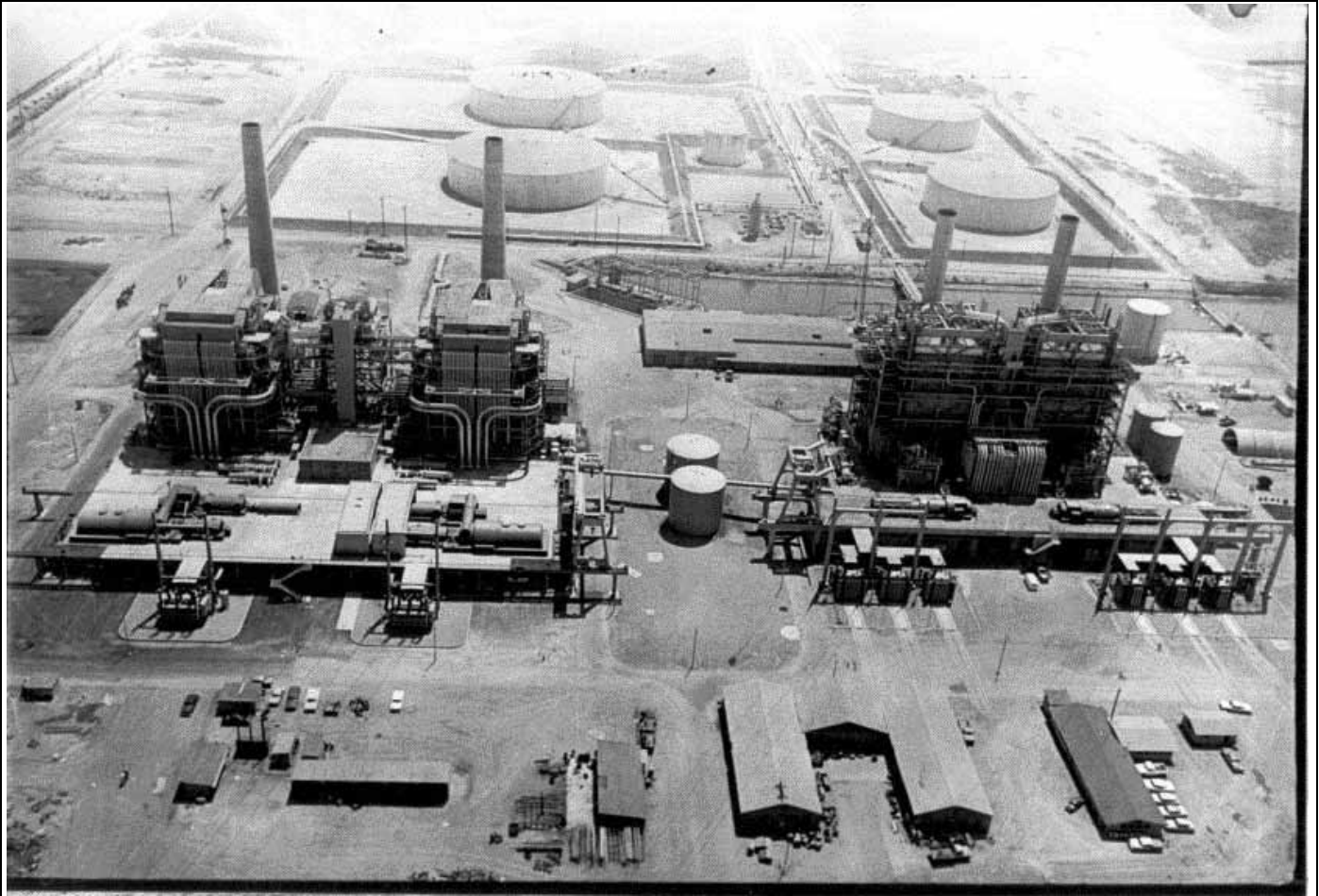
Unit pairs 1 and 2 (on the right) and 3 and 4 (on the left), aerial view looking south, October 1962. Photo from Long Beach Press-Telegram archive files. Construction facilities (no longer extant) are visible along the bottom of the photo.
