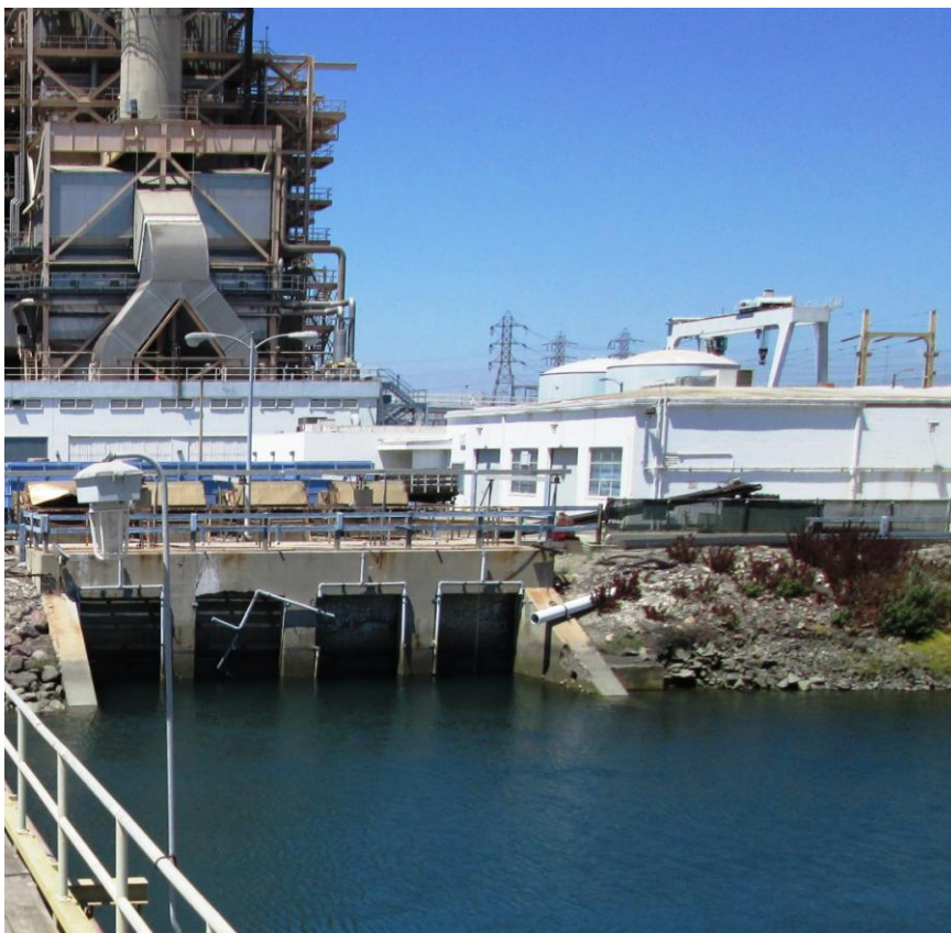
North Intake Channel, view looking north at intake structure for Units 1 and 2
