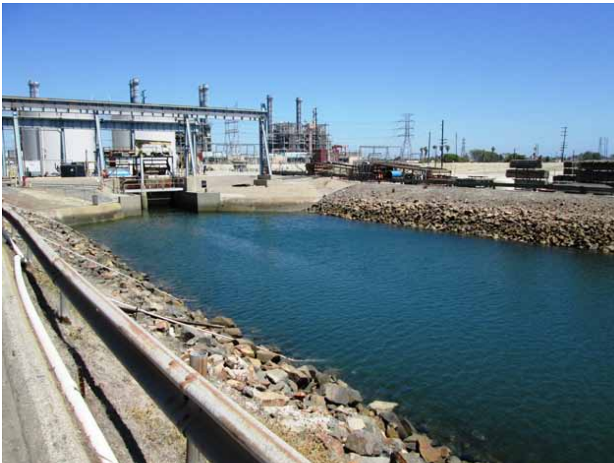
Intake Channel, view looking southeast at intake structure for Unit 6
