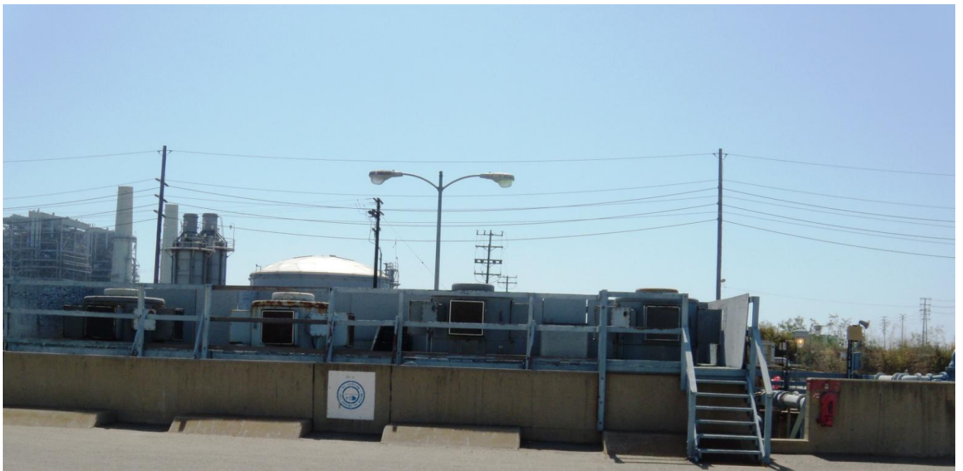
Units 1 and 2 recirculating water intake – north intake channel is immediately south (not visible), view looking south. Units 5 and 6 are visible in the distance at left.
