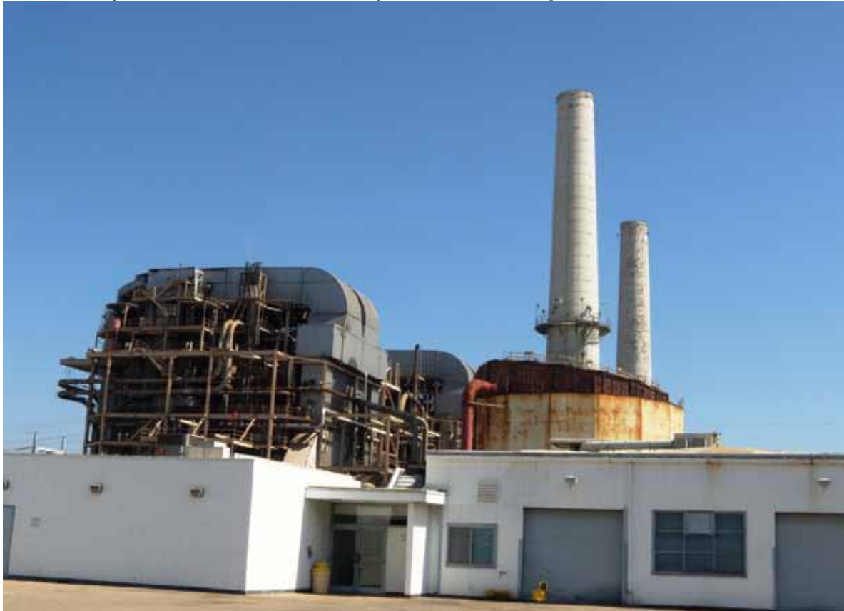
Units 3 and 4 with maintenance/locker room in the foreground, view looking northeast.
