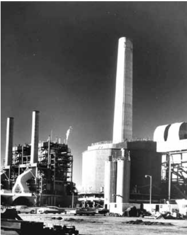
Unit 3 with bag house, view looking northwest. Units 1 and 2 are visible at the far left. 1960s photo. (Photo by Doug White. From the Edison Archive. Courtesy of The Huntington Library, San Marino, CA)
