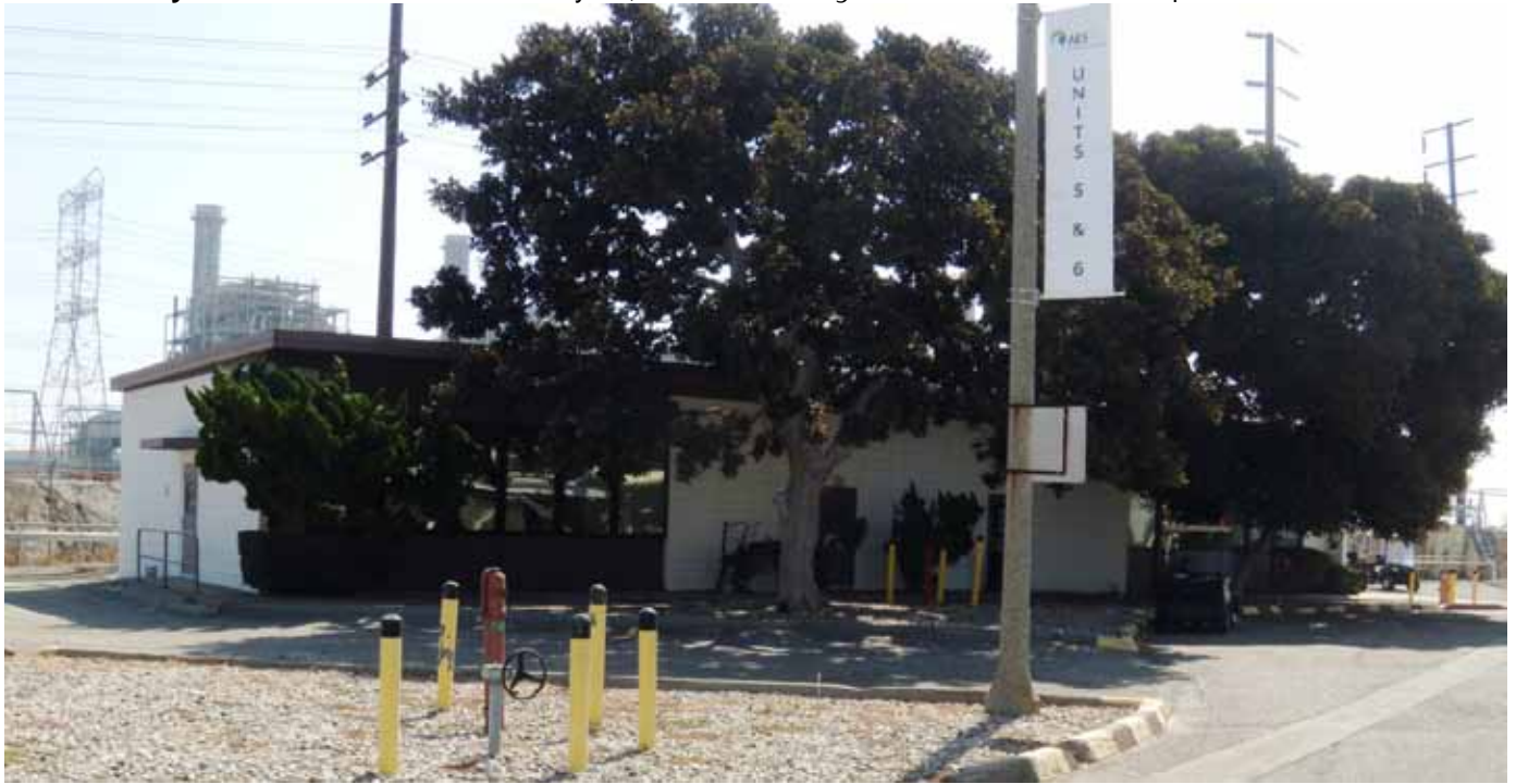
Units 5 and 6 Administration Building, view looking southeast
