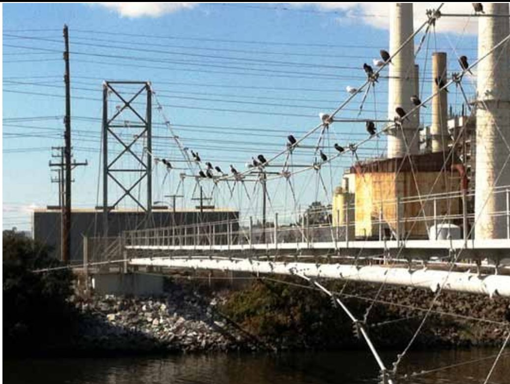
View looking northwest at pipeline suspended across San Gabriel River. February 2014.
