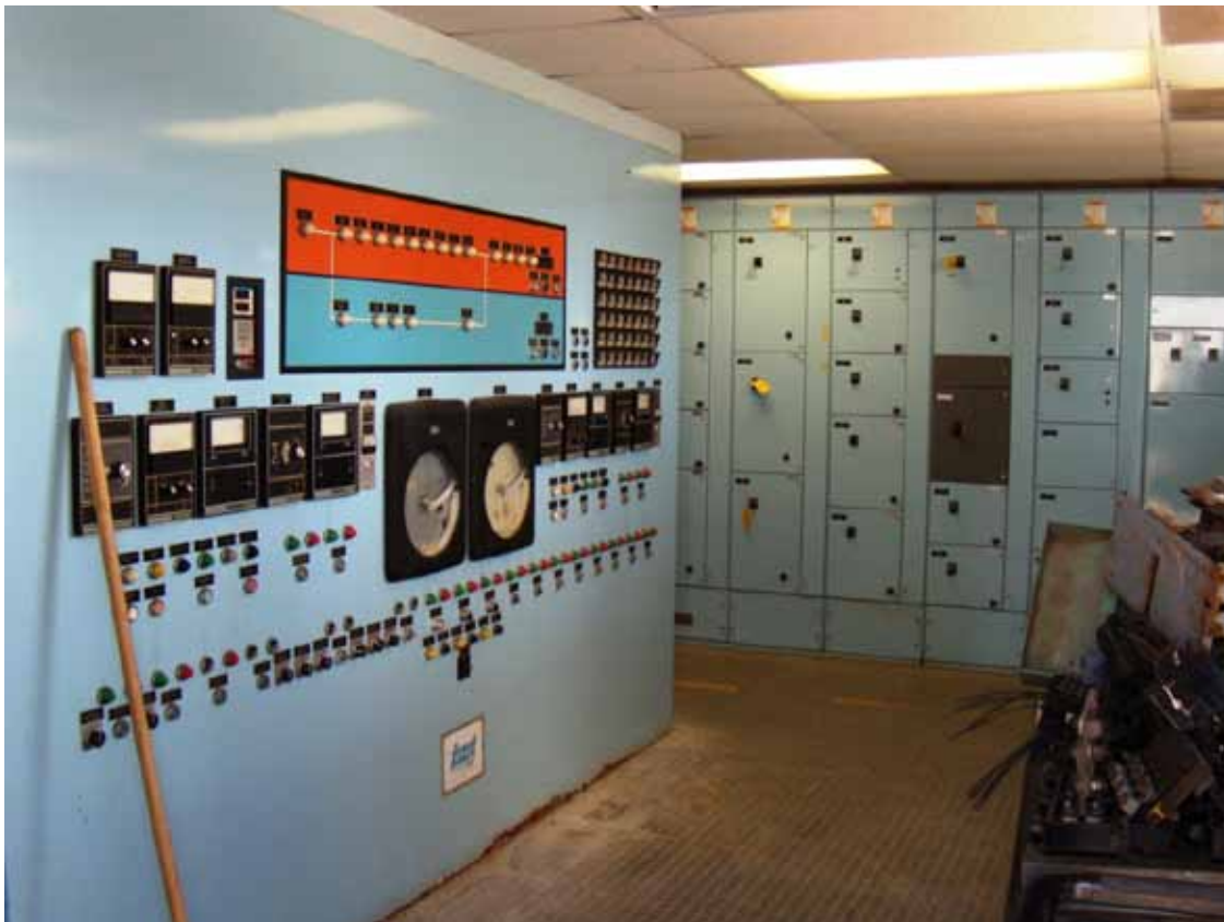
Interior view – Mud Controls Building for Units 5 and 6.
