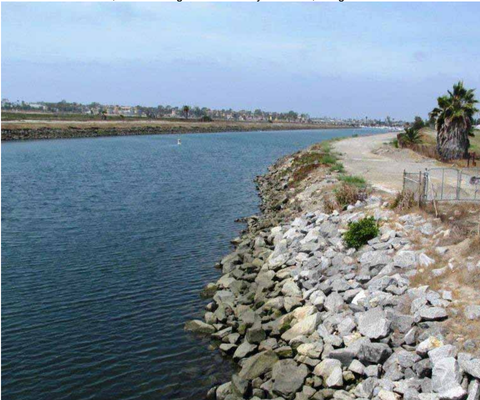
Los Cerritos Channel, view looking southwest from Loynes Drive. July 2013.
