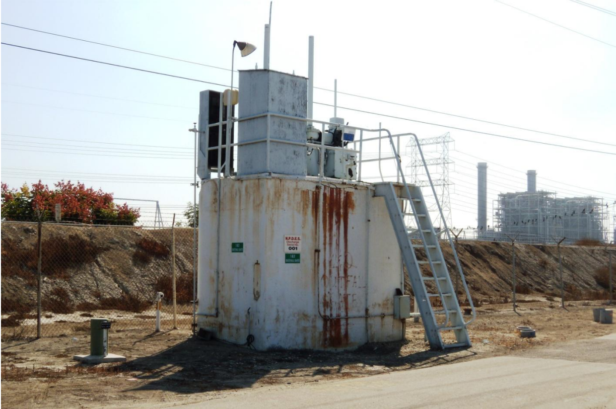
Units 1 and 2 Outfall Gates, view looking southeast.
