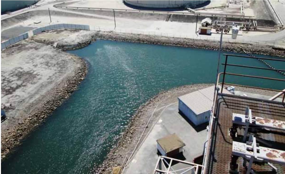
Intake Channel, view looking southwest at southwest corner of channel
