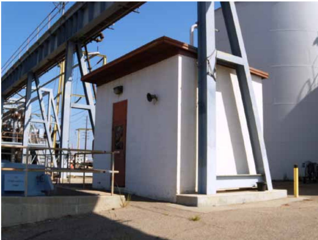
Unit 6 Screen Wash Controls House, view looking northeast
