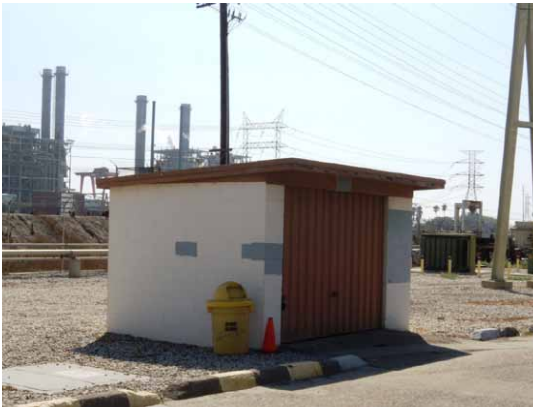
Units 5 and 6 east side hose house, view looking southeast
