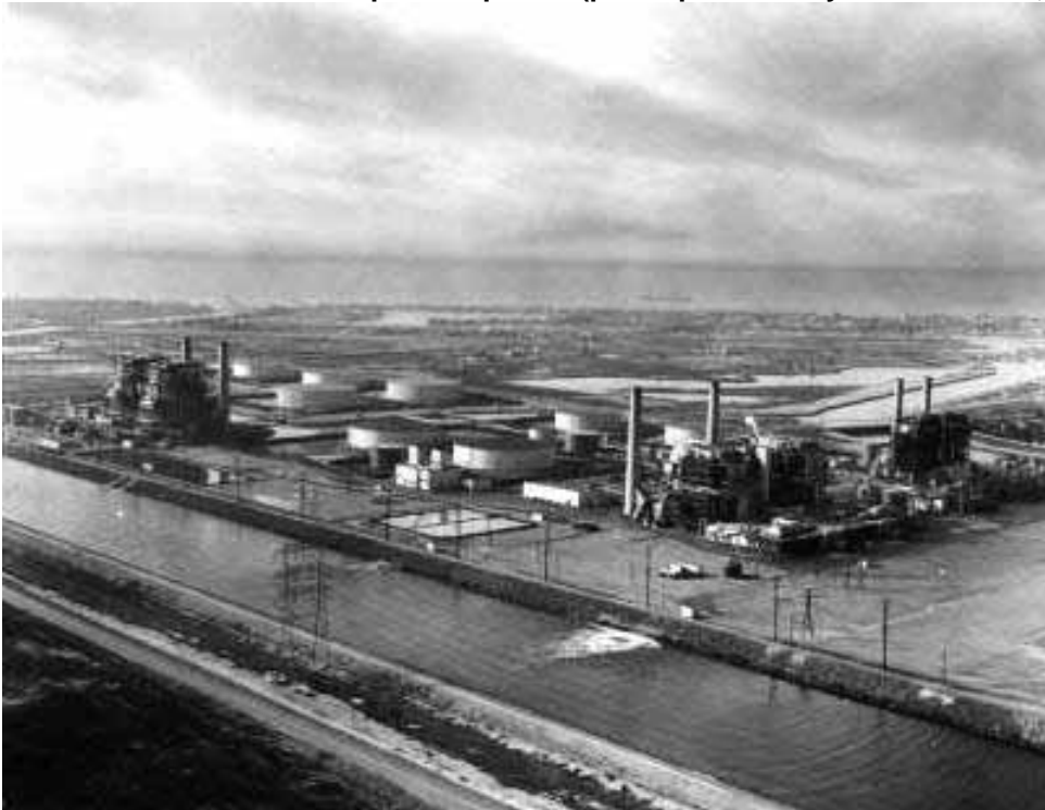
Aerial view of Alamitos Generating Station, view looking southwest, taken August 26, 1972. (photo by Joseph Fadler, from the Edison Archive. Courtesy of The Huntington Library, San Marino, CA)
