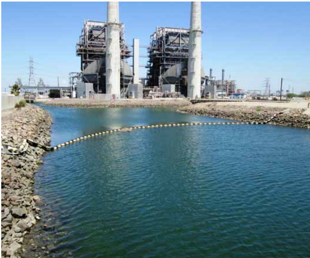
Intake Channel, view looking east, Units 5 and 6 in background
