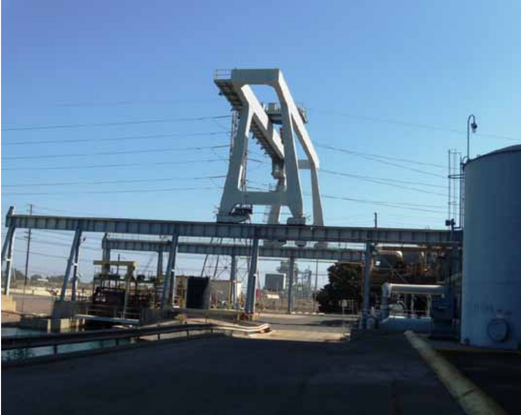
Gantry crane for Units 5 and 6, view looking east.
