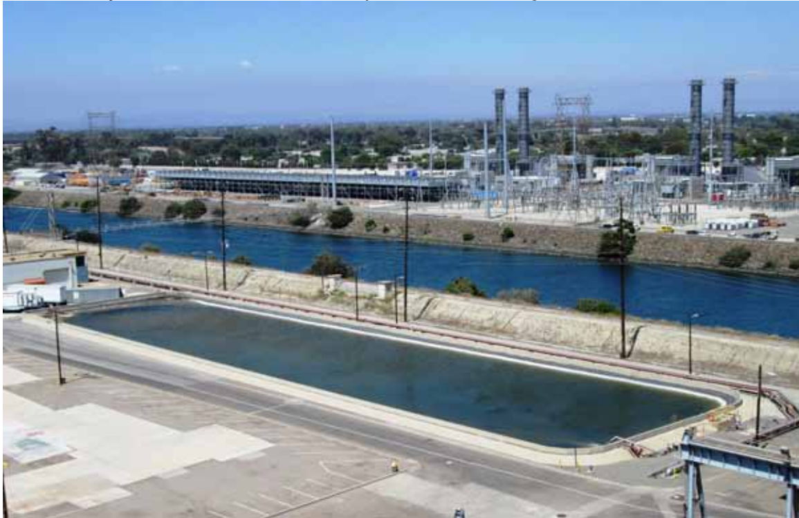
South Retention Basin, view looking northeast; San Gabriel River in the background
