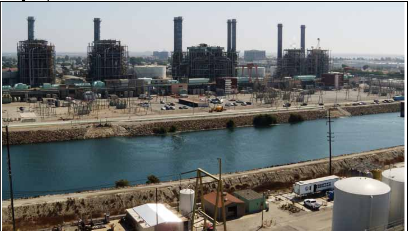
View looking east from AES Alamitos. West bank levee is near bottom of photo with San Gabriel River in center of photo. Haynes Generating Station outfalls are visible in east bank levee. September 2011.
