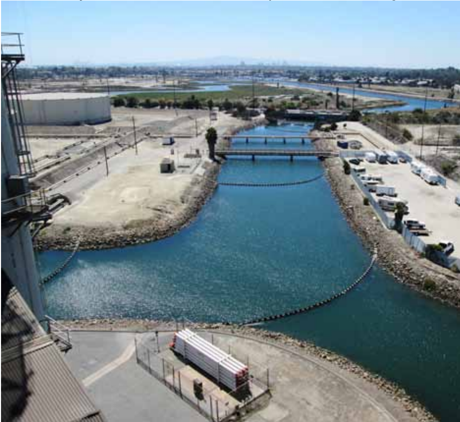
Intake Channel, view looking west
