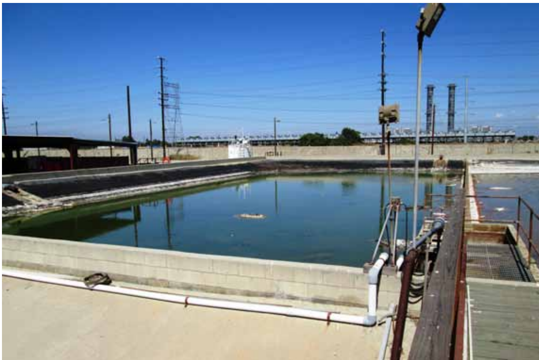
North end of Central Retention Basin – view to east
