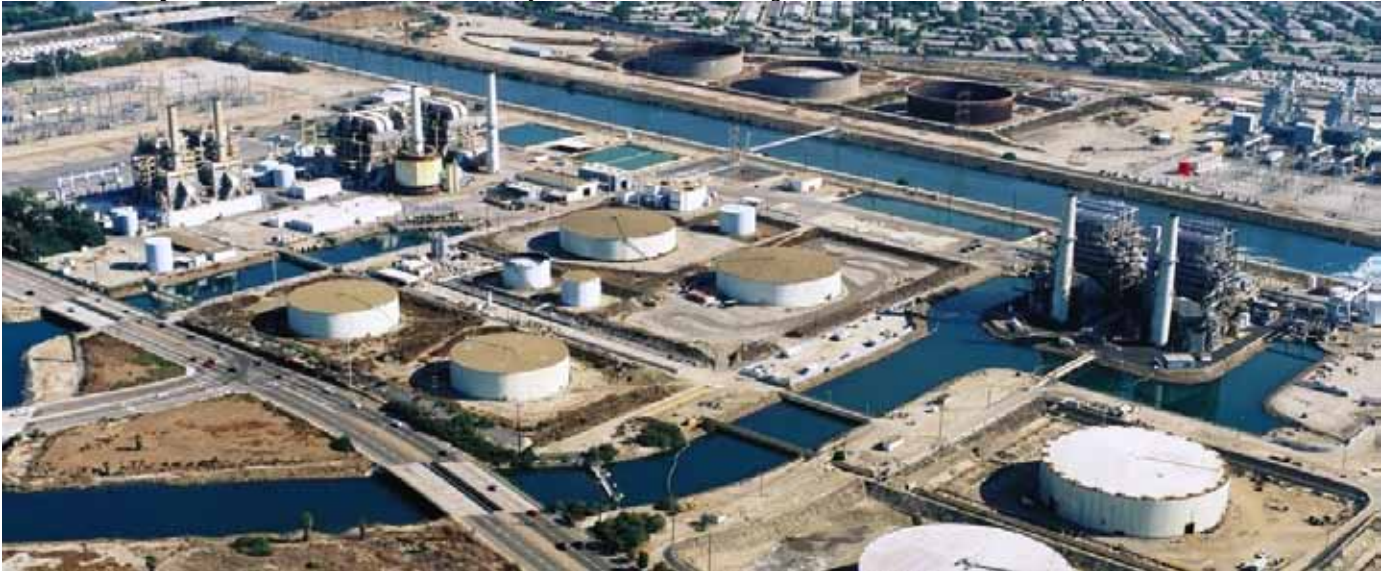
Aerial view of Alamitos Generating Station, view looking northwest, taken in 2006 before the fuel tanks in the center parcel were removed. Units 1 through 4 are at the upper left, Units 5 and 6 are on the far right. The San Gabriel River is near the top of the photo. (photo provided by AES Alamitos, LLC)
