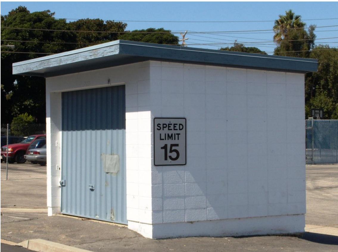
Units 1 and 2 Hose House (typical of all hose houses on the facility), view looking northwest.
