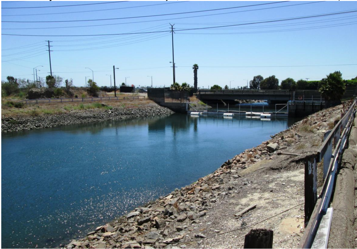
North Intake Channel, view looking southwest
