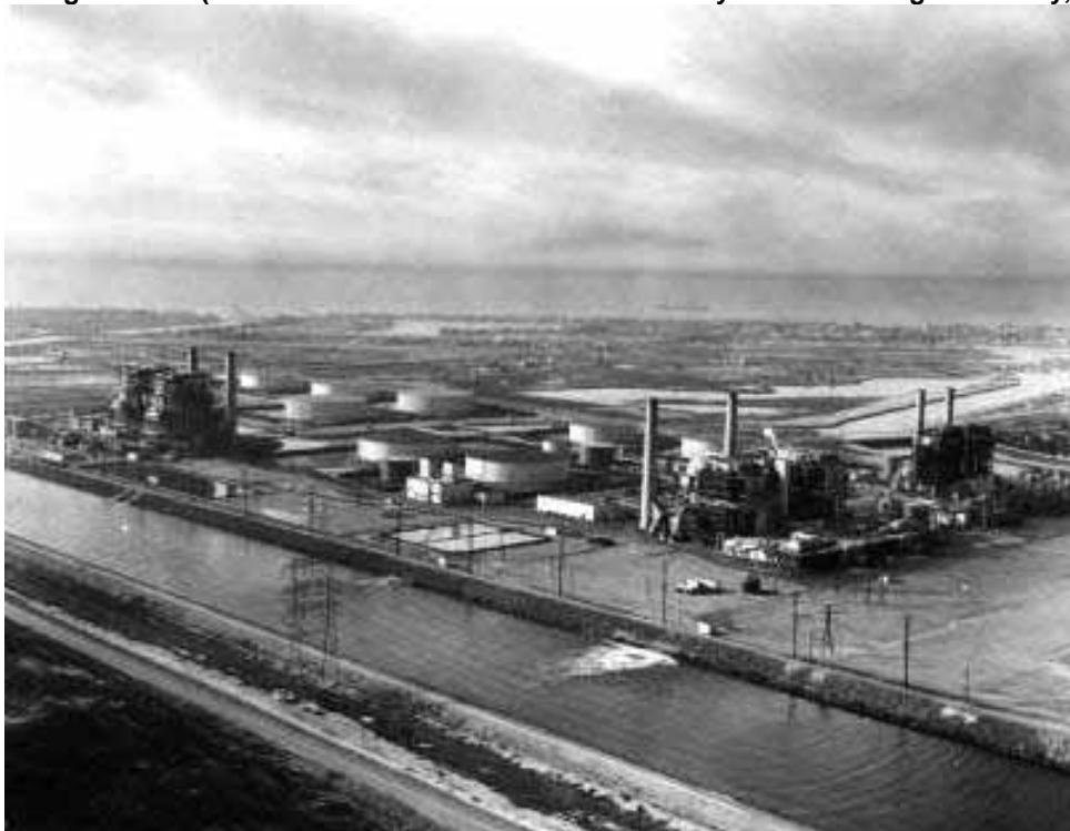
Aerial view of Alamitos Generating Station, view looking southwest, taken August 26, 1972. Armored levees and outfalls are in place. (Photo by Joseph Fadler, from the Edison Archive. Courtesy of The Huntington Library, San Marino, CA)
