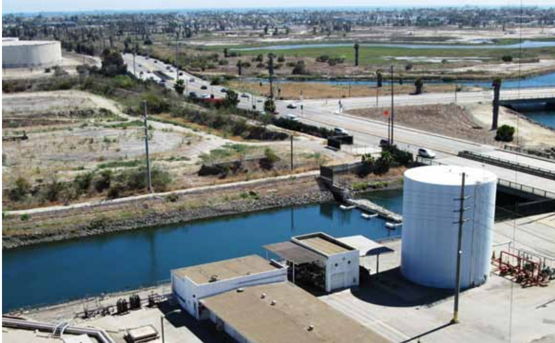
North intake channel – aerial view to southwest
