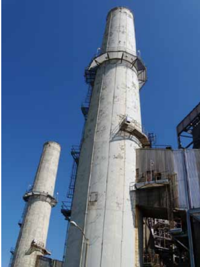
Units 5 and 6 Stacks, view looking north.
