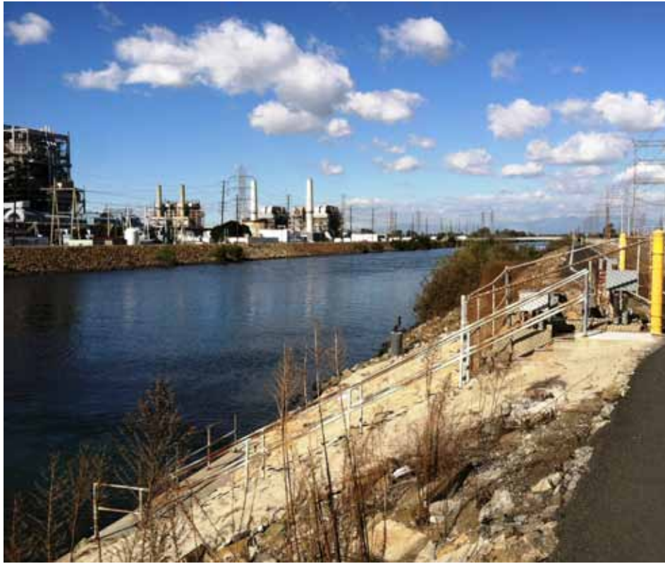
View looking northwest with outfall for Haynes Generating Station and east bank levee in foreground. February 2014.
