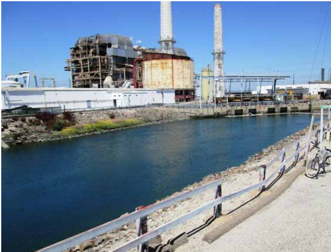
North intake channel – view to northeast looking towards intake structure for Units 3 and 4
