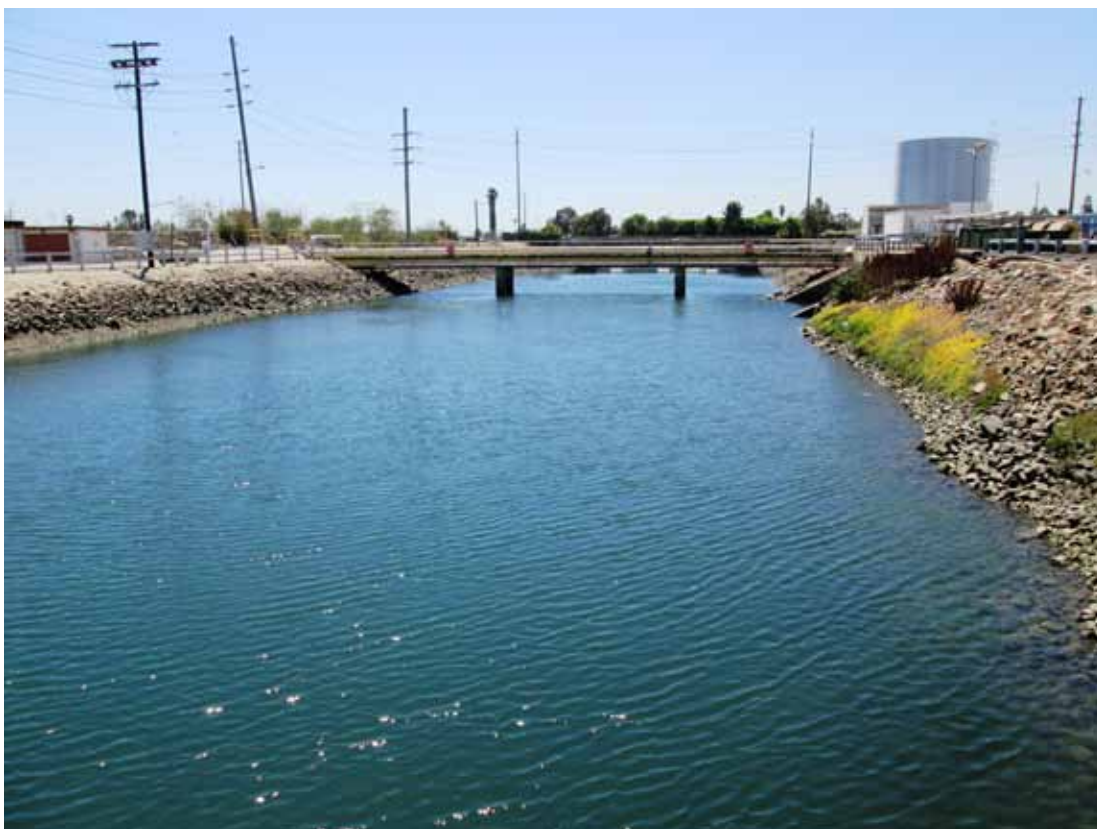
North intake channel – view to north
