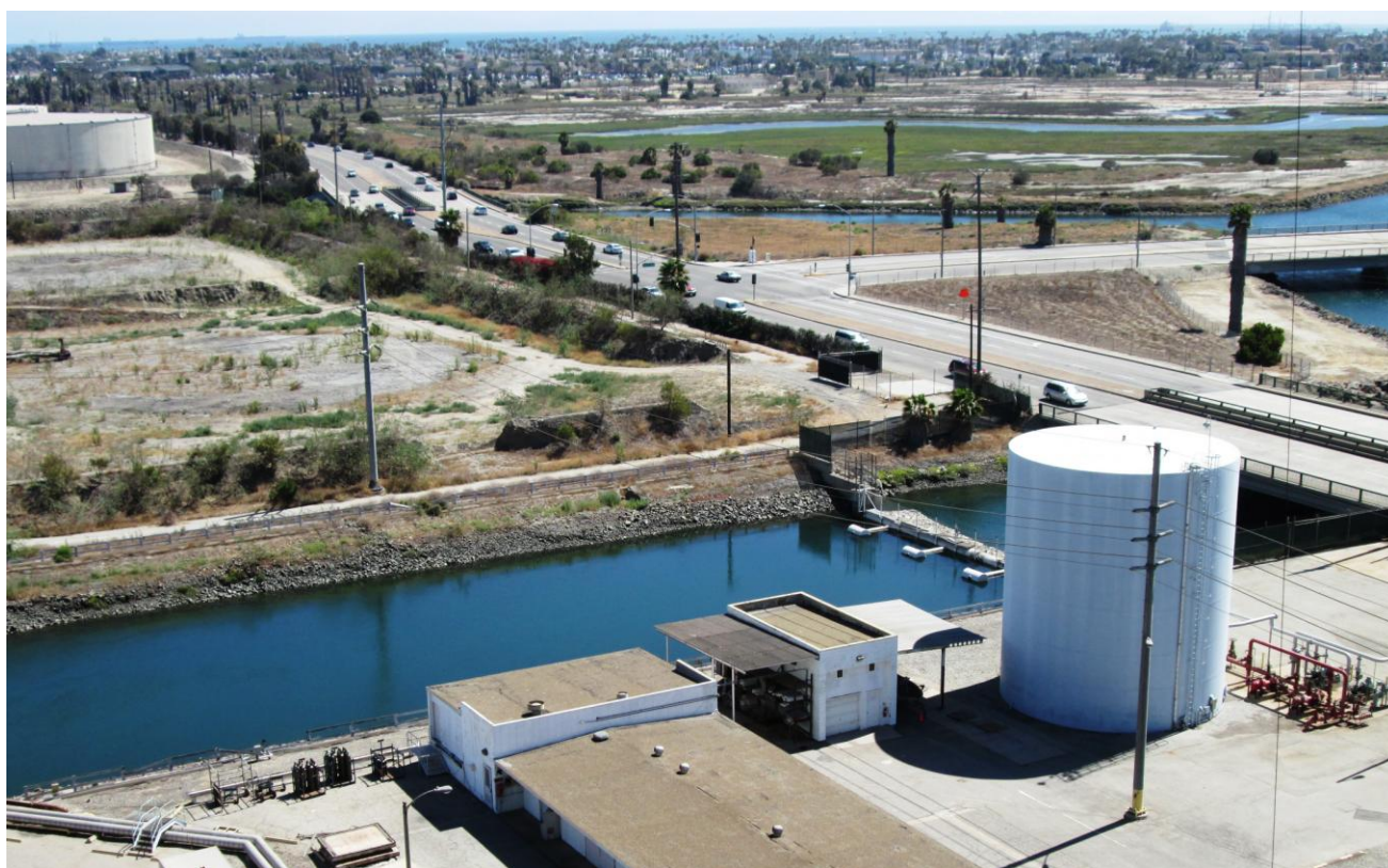
North Intake Channel, aerial view looking southwest
