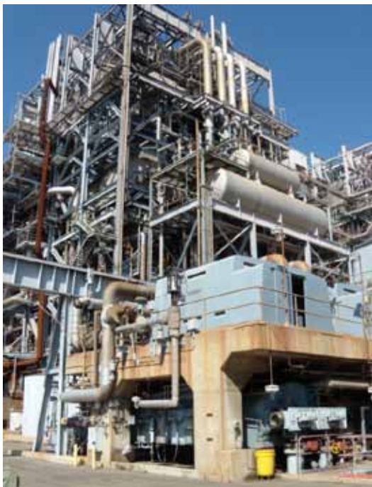
Unit 6, view looking northwest.
