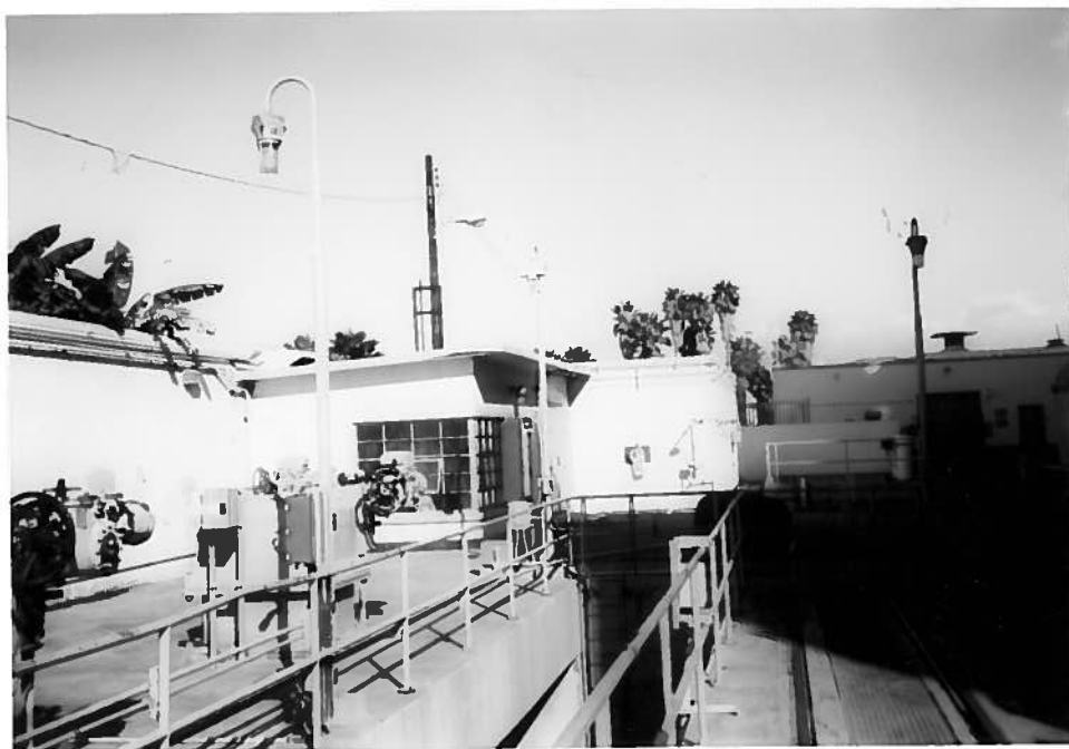
Photo 6. Screenwell structure of seawater intake system for Units No. 1 and 2 in foreground. Screenwell control house just left of center, with seawall visible to rear.
