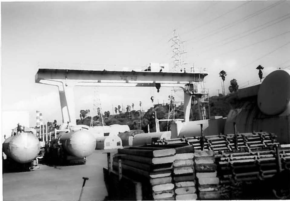
Photo 11. Gantry crane, Units No. 3 and 4.
