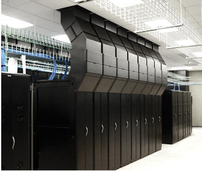
Figure 5. Example return air chimney and enclosed server rack product.
