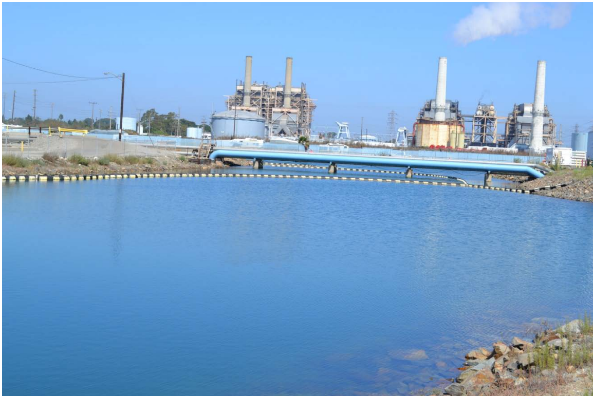
Alamos Energy Center. Photo of existing channel and facilities, view facing north.
