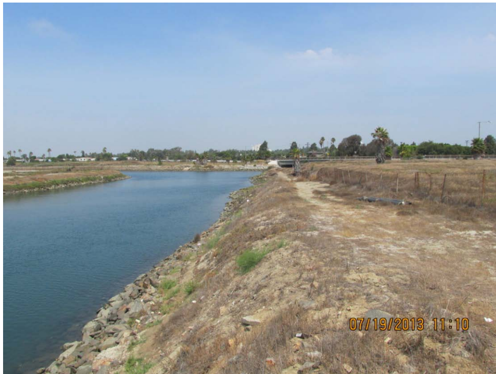
Alamitos Energy Center. Photo from the channel from the AES site and south of Loynes Drive, view facing northwest.
