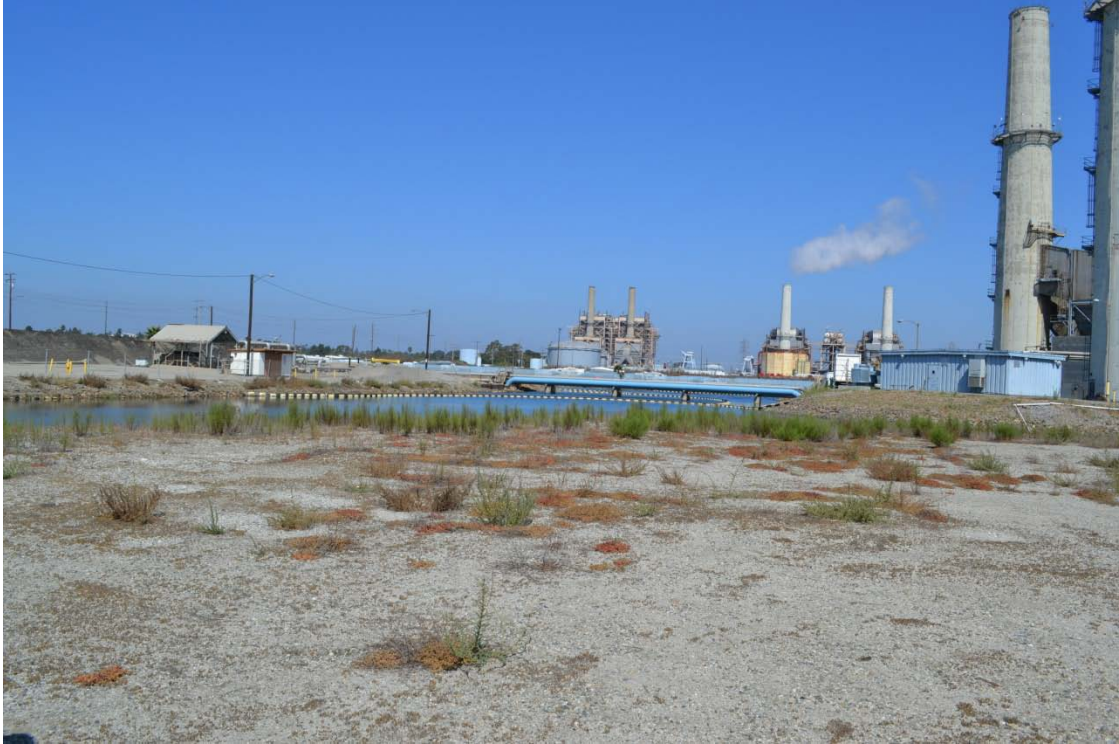
Alamos Energy Center. Photo of existing channel and facilities, view facing north northwest.
