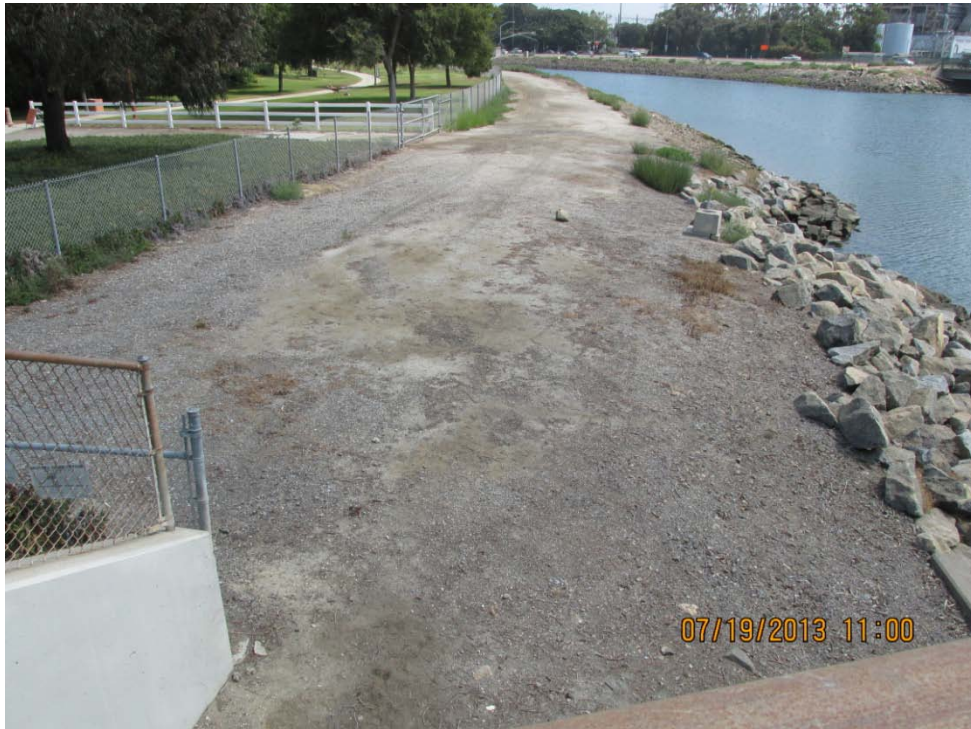
Alamitos Energy Center. Photo from the northwest corner of the existing bridge over Loynes Drive, view facing northeast.
