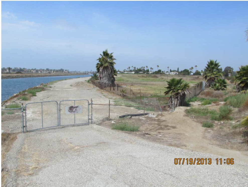
Alamitos Energy Center. Photo from the southwest corner of the existing bridge over Loynes Drive, view facing southwest.
