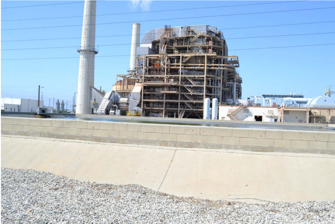
Alamos Energy Center. Photo of existing facilities, view facing west southwest.
