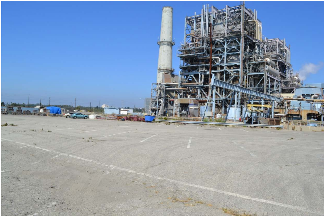
Alamos Energy Center. Photo of existing facilities, view facing northwest.
