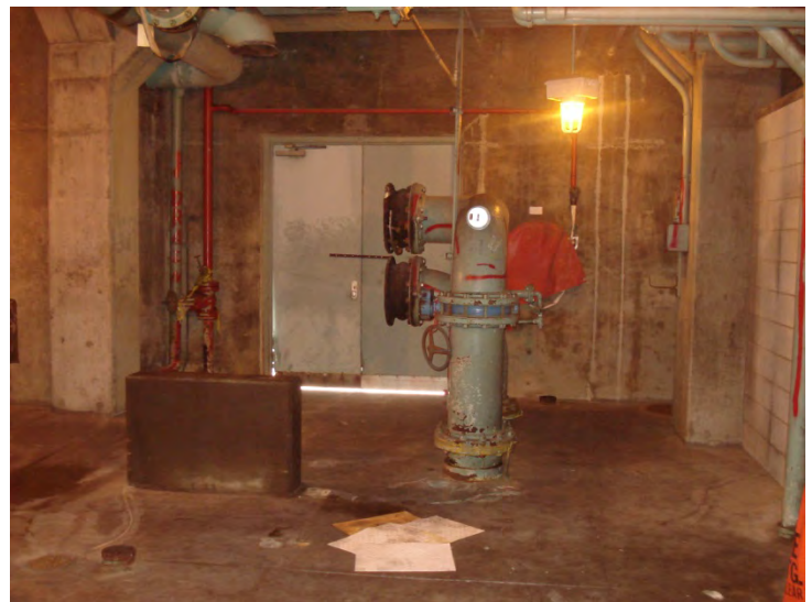
Photograph 32: Interior of former Unit 7 peaker building.
