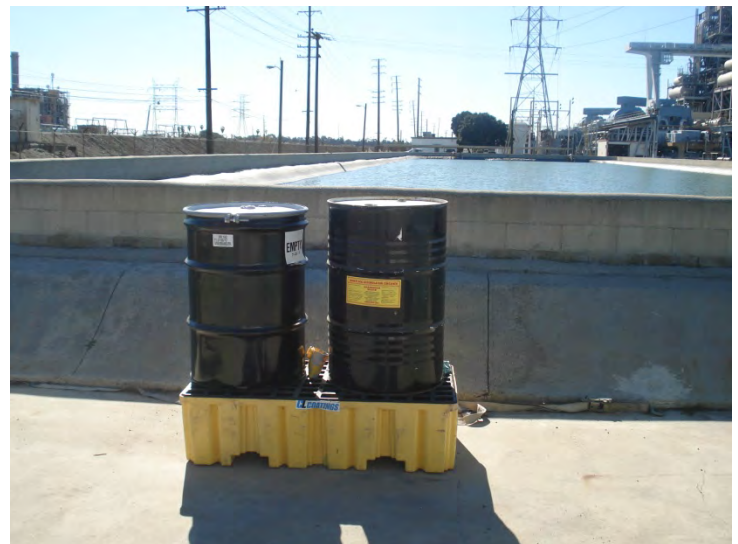
Photograph 30: Two 55-gallon drums located on secondary containment.
