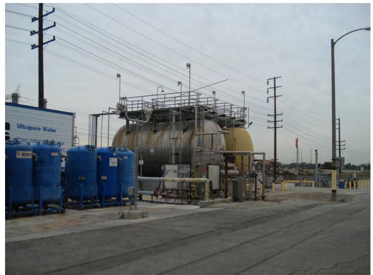
Photograph 18: Out-of-service acid and caustics tanks.
