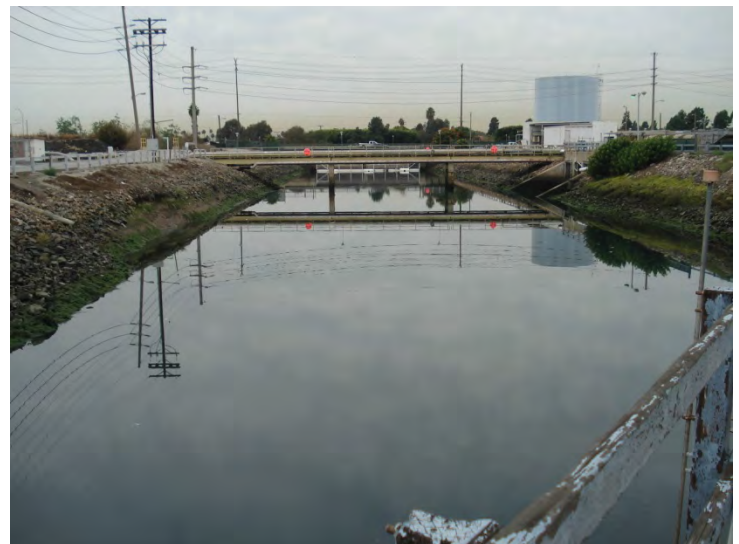
Photograph 21: Intake channel to Units 5 and 6.
