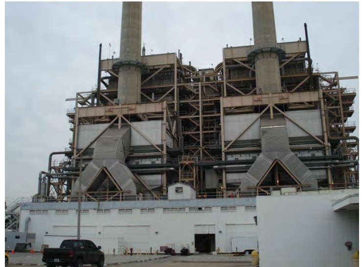
Photograph 1: Twin power plant Units 5 and 6.
