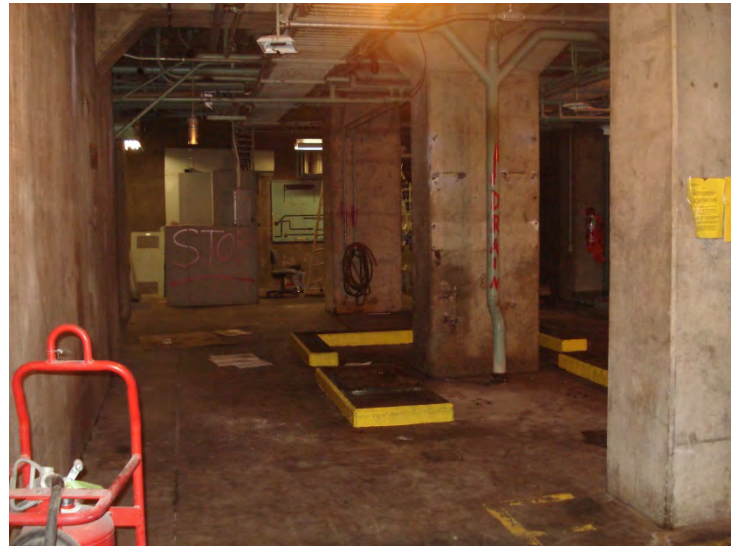
Photograph 31: Interior of former Unit 7 peaker building.
