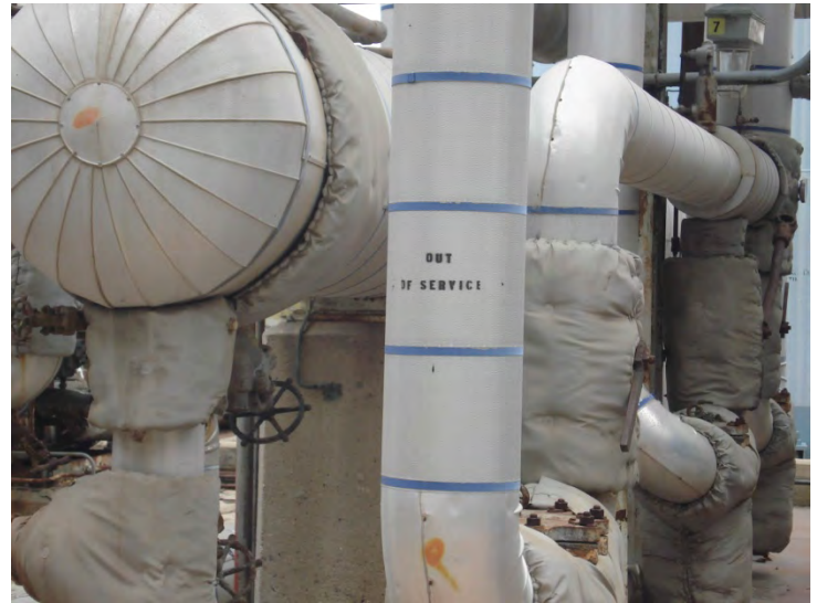
Photograph 19: Out-of-service fuel oil handling facility.
