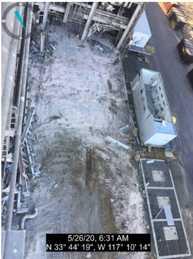
Demo on the west side of Unit 2
