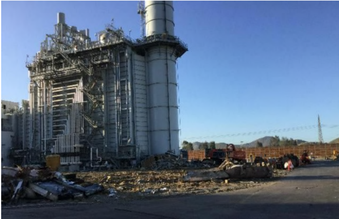
2020/05/04 Looking at Unit 2, facing southeast.
