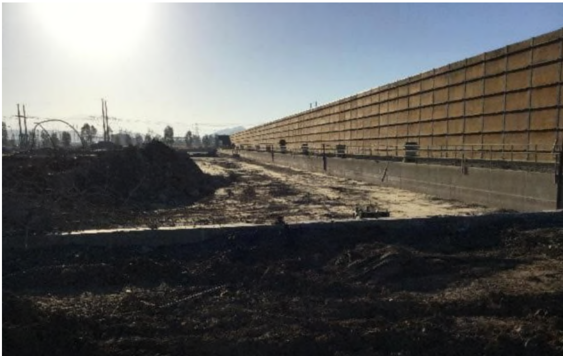
2020/05/04 Cooling tower area, looking east.
