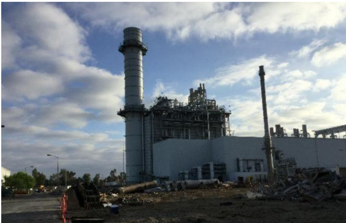
2020/05/11, 06:56:31 Unit 1 looking north.
