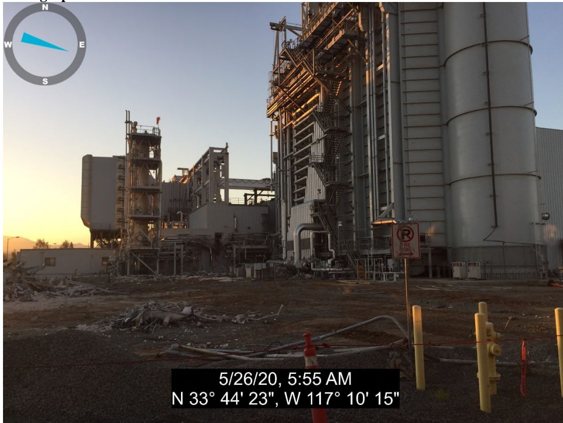
North side of Unit 1, facing east.
