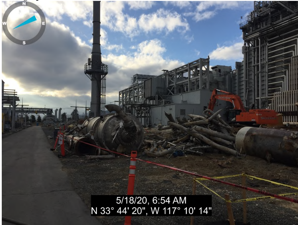
North side of Unit 2 and courtyard, facing east.
