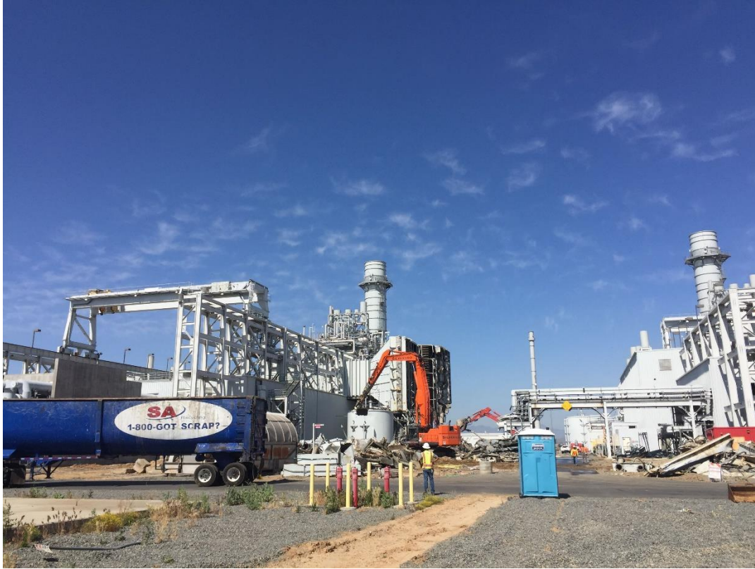
Silverado crews working to demo air intake on Unit 2/courtyard.
