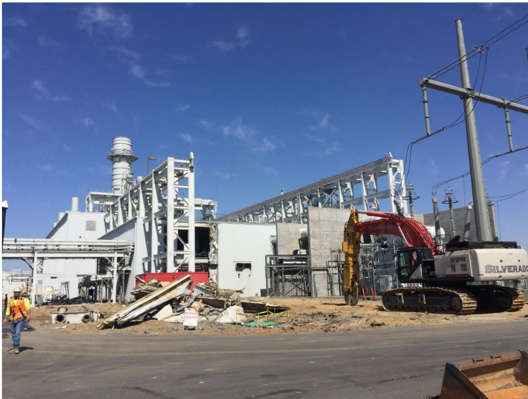
Other crews still working on turbine deck of Unit 1.
