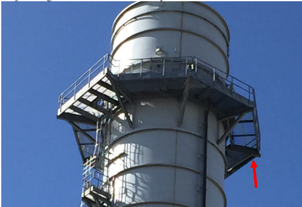
Arrow showing location of Kingbird nest construction.
