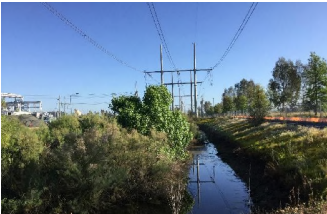
2020/05/04 East retention basin looking north.
