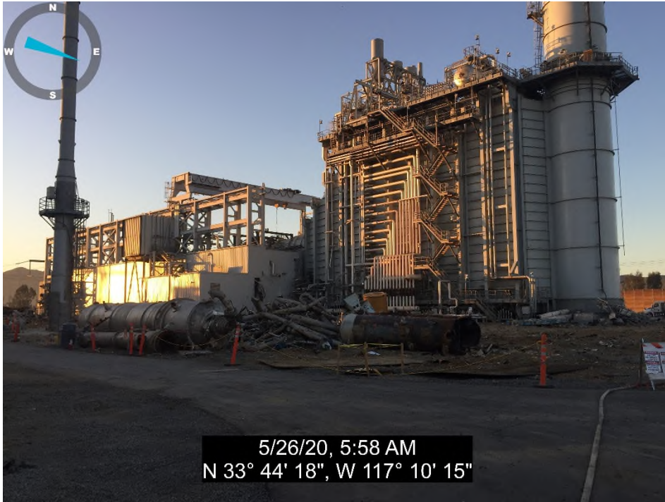
Courtyard and Unit, looking southeast.
