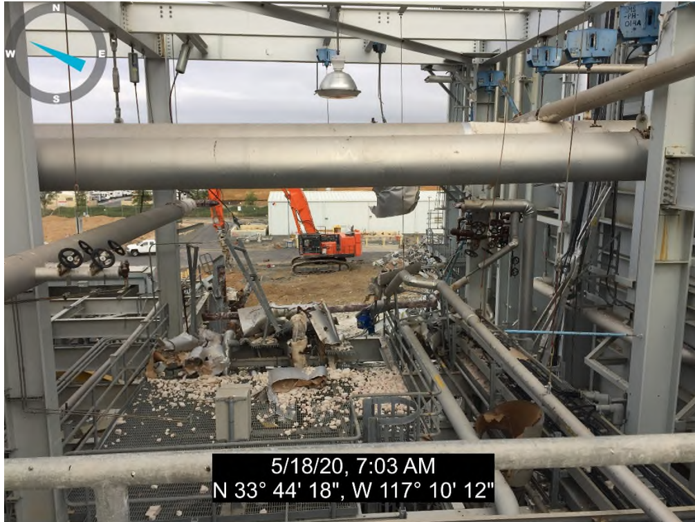
Demo on the west side of Unit 2, from the Turbine deck.
