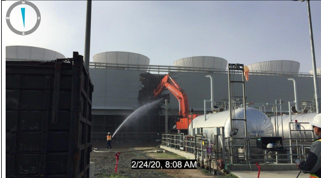
Crews starting demolition of cooling tower
