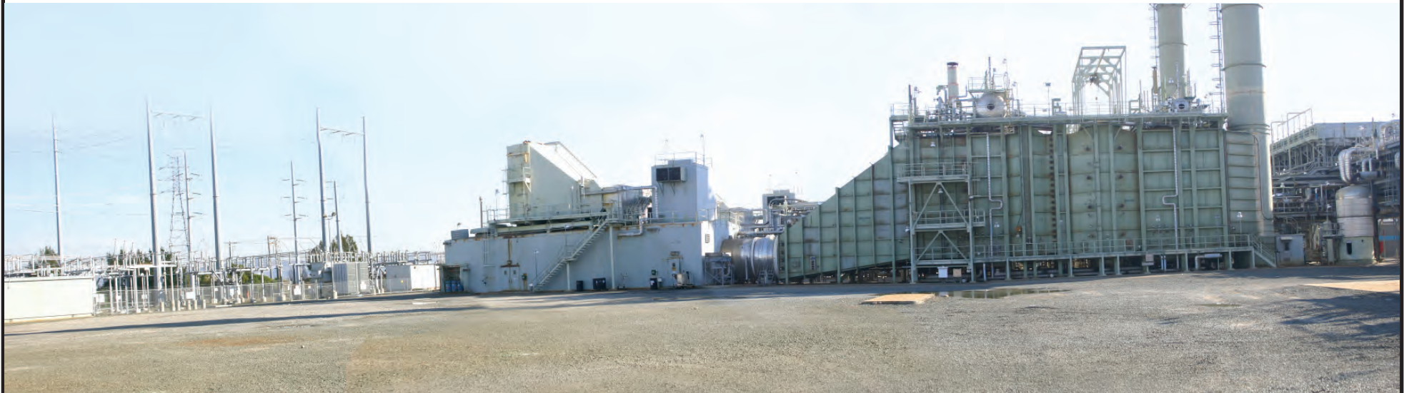
Photo 2: Existing view looking southeastward across the site of the proposed cogeneration facility.
