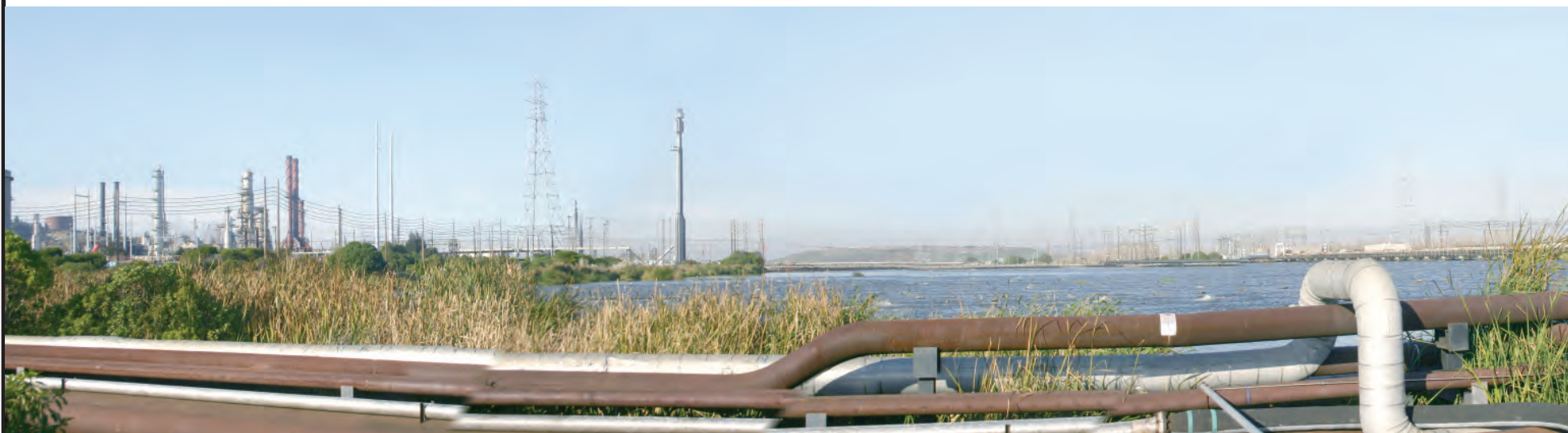
Photo 3: Existing view looking toward the transmission line that will be reconducted as a part of the proposed Project.
