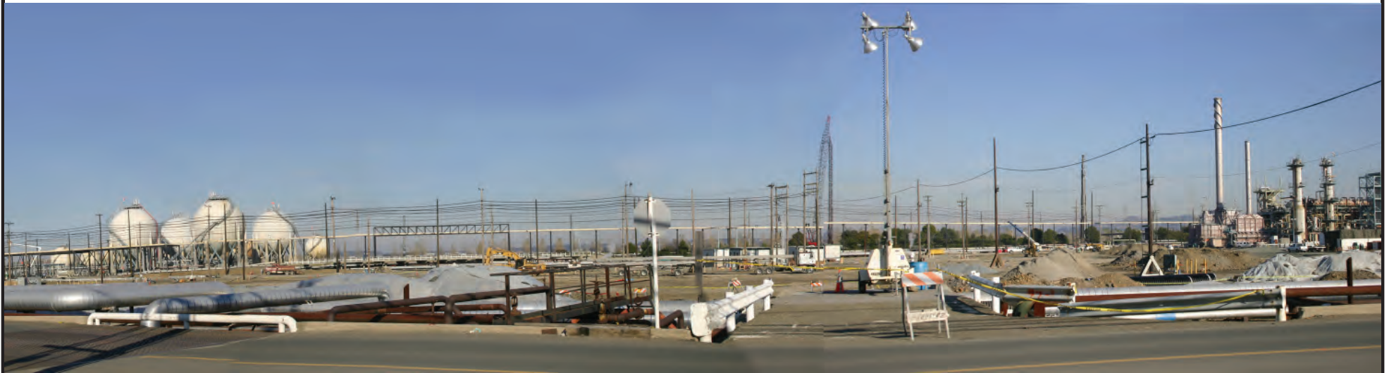
Photo 1: Existing view looking eastward across the site of the proposed hydrogen plant where the steam turbine generator, cooling tower, and switchgear that are part of the PPRP will be located.
