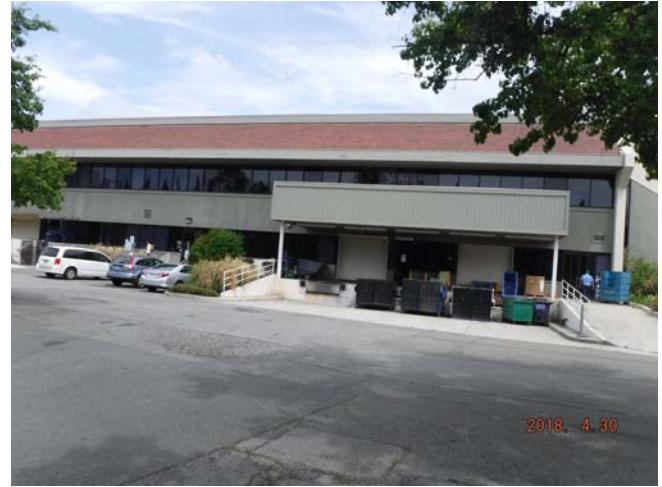
Photo 2: View of the south side of 2825 Lafayette Street, looking north.
