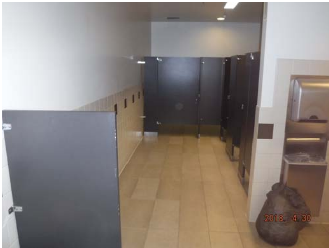
Photo 9: View of an example restroom facility.
