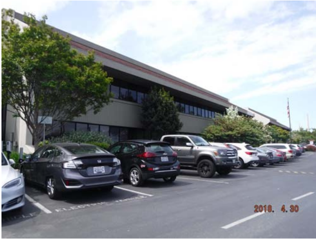
Photo 1: View of the north side of 2825 and 2845 Lafayette Street, looking southwest.
