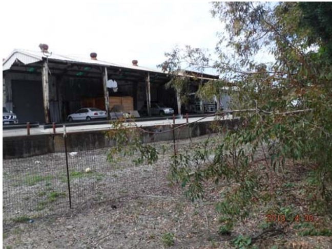
Photo 27: View of the south adjacent site, looking south.
