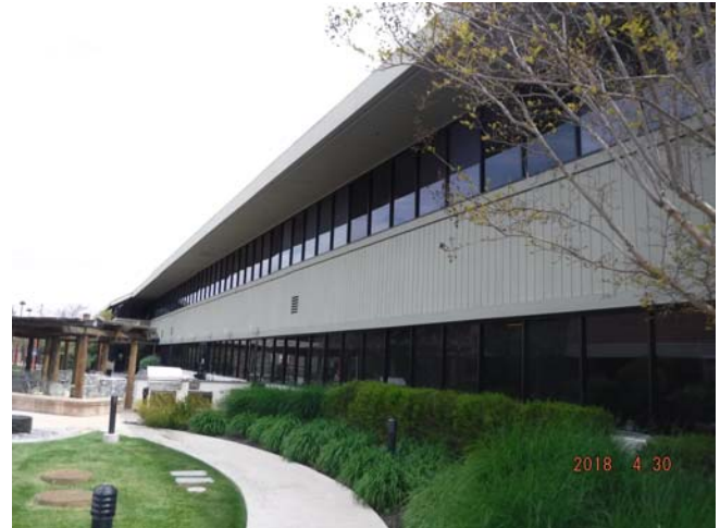
Photo 4: View of the west side of 2825 Lafayette Street, looking north.
