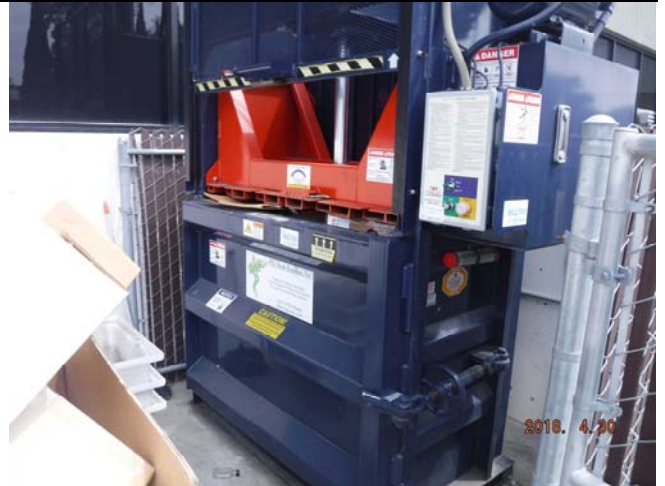
Photo 20: View of a hydraulic compactor.
