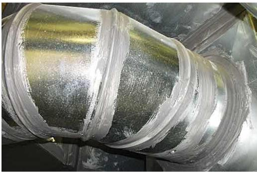
**Figure 21: Duct with mastic applied.**
