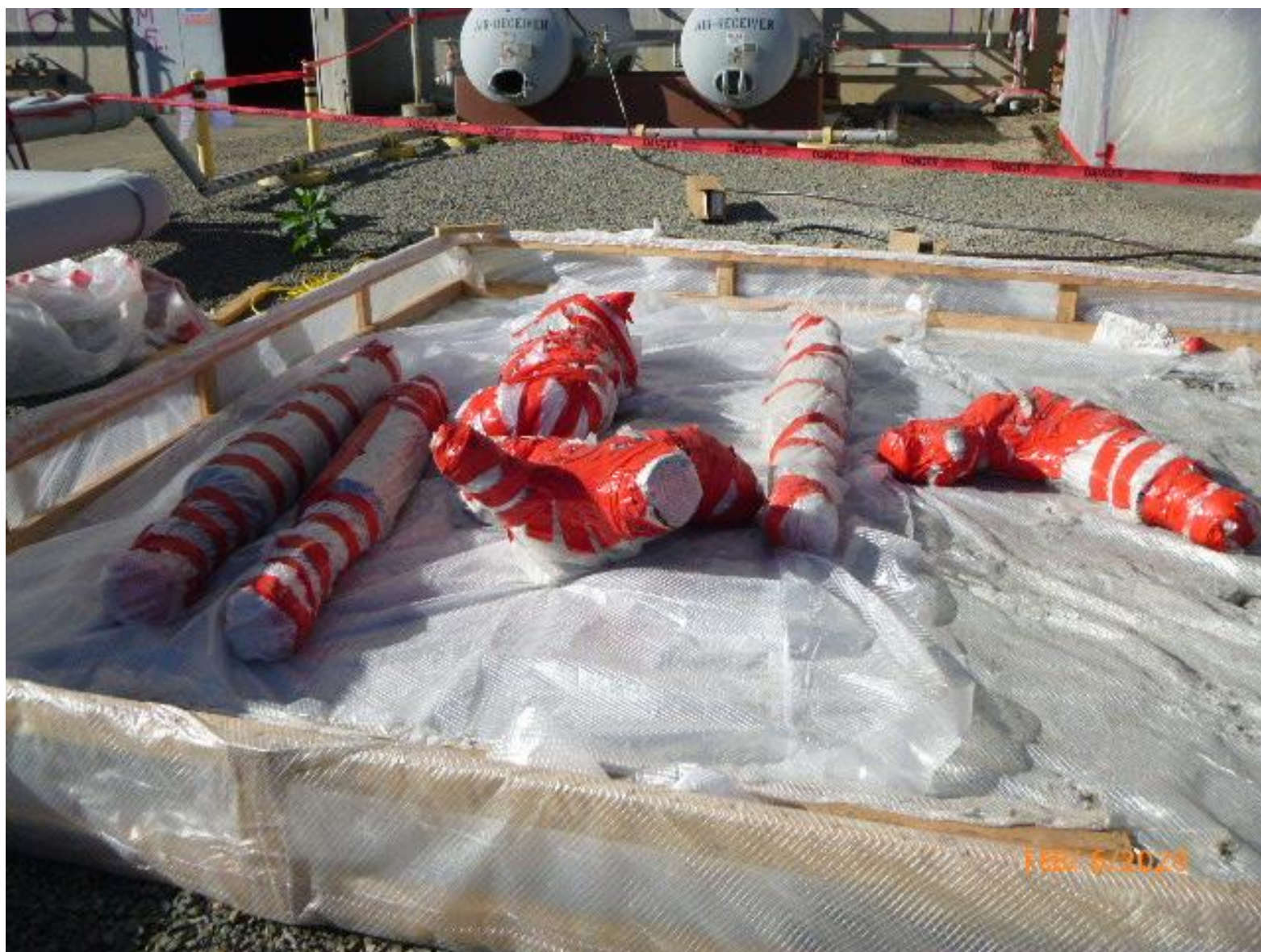
Photo #5: Removed sections of oil piping wrapped and taped in containment area prior to loading and removal.
