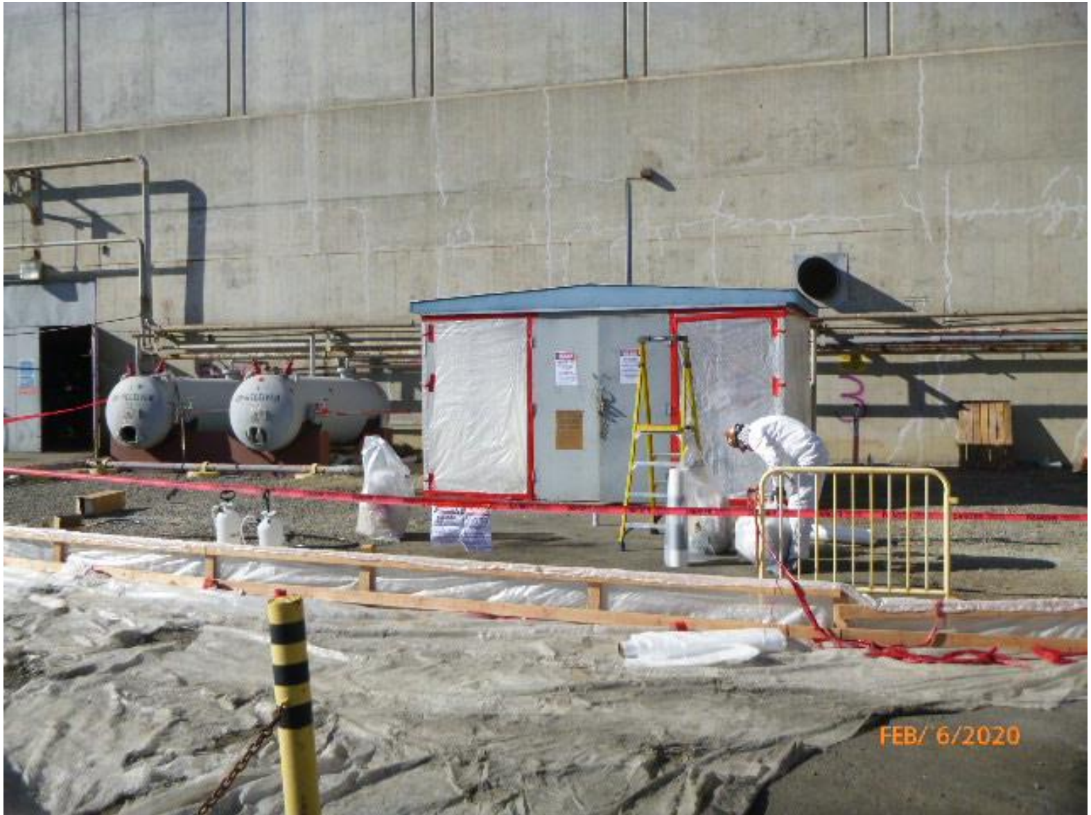
Photo #6: Modular building siding taped, and poly wrapped for containment prior to removal and disposal.
