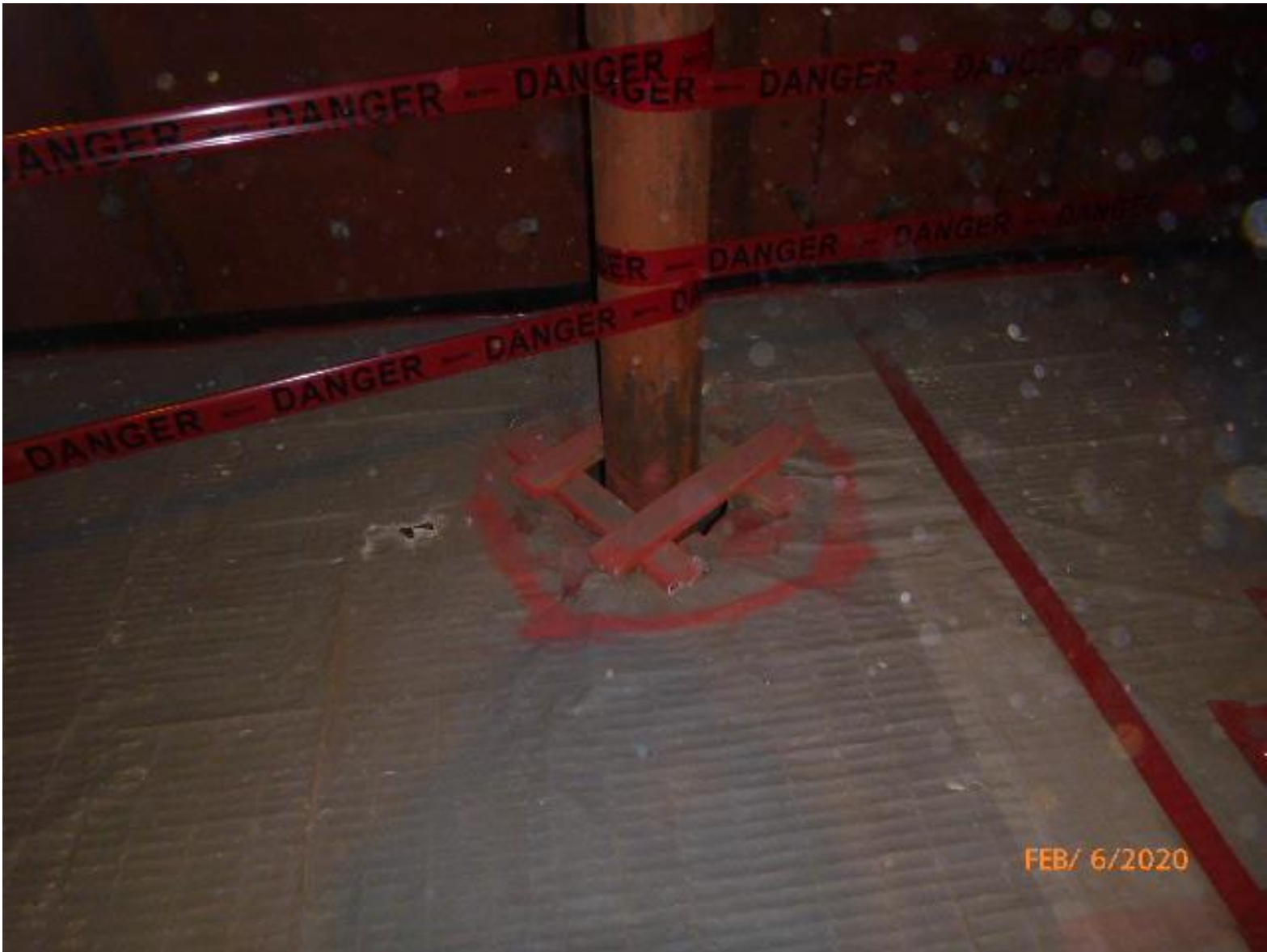
Photo #4: Floor opening protection closed after removal of jacket insulation from pipe penetration.
