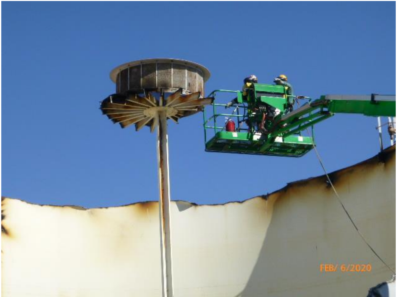
Photo #2: Craft Workers in aerial bucket cutting steel sections of water tank walls and center support column.
