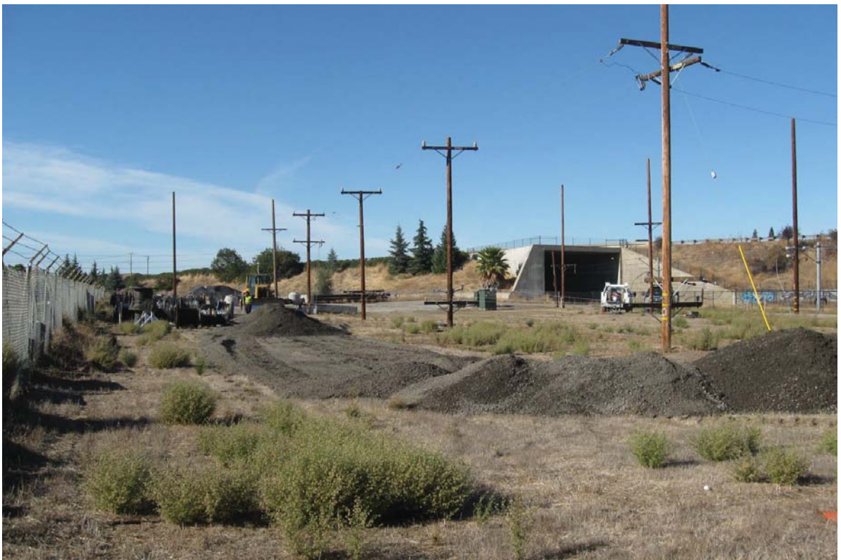
PHOTO 6: Existing view of the PG&E Edenvale Service Center from the southeastern corner of the site looking northwest.
