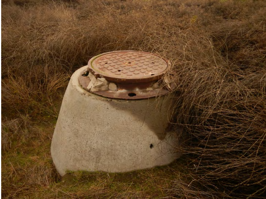
Photograph 9. View of a storm drain vault that indicates an underground pipe running along the northern boundary of the proposed storage area.
