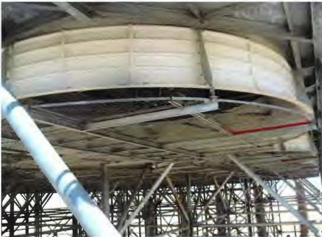
**Photo 3. An overview of the ACC underside showing cells with fans inside housing (plenum) above grates, and infrastructure.**
