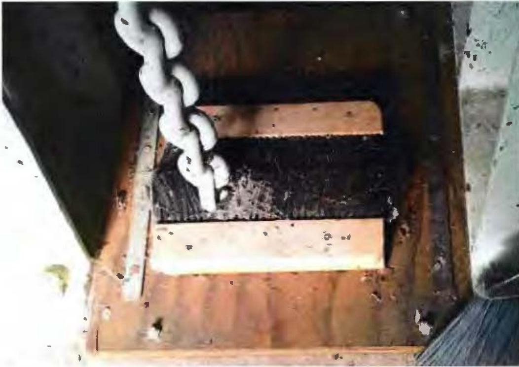
**Photo 6. Brush heads block the space around a chain passing through a concrete deck in a PG&E dam.**
