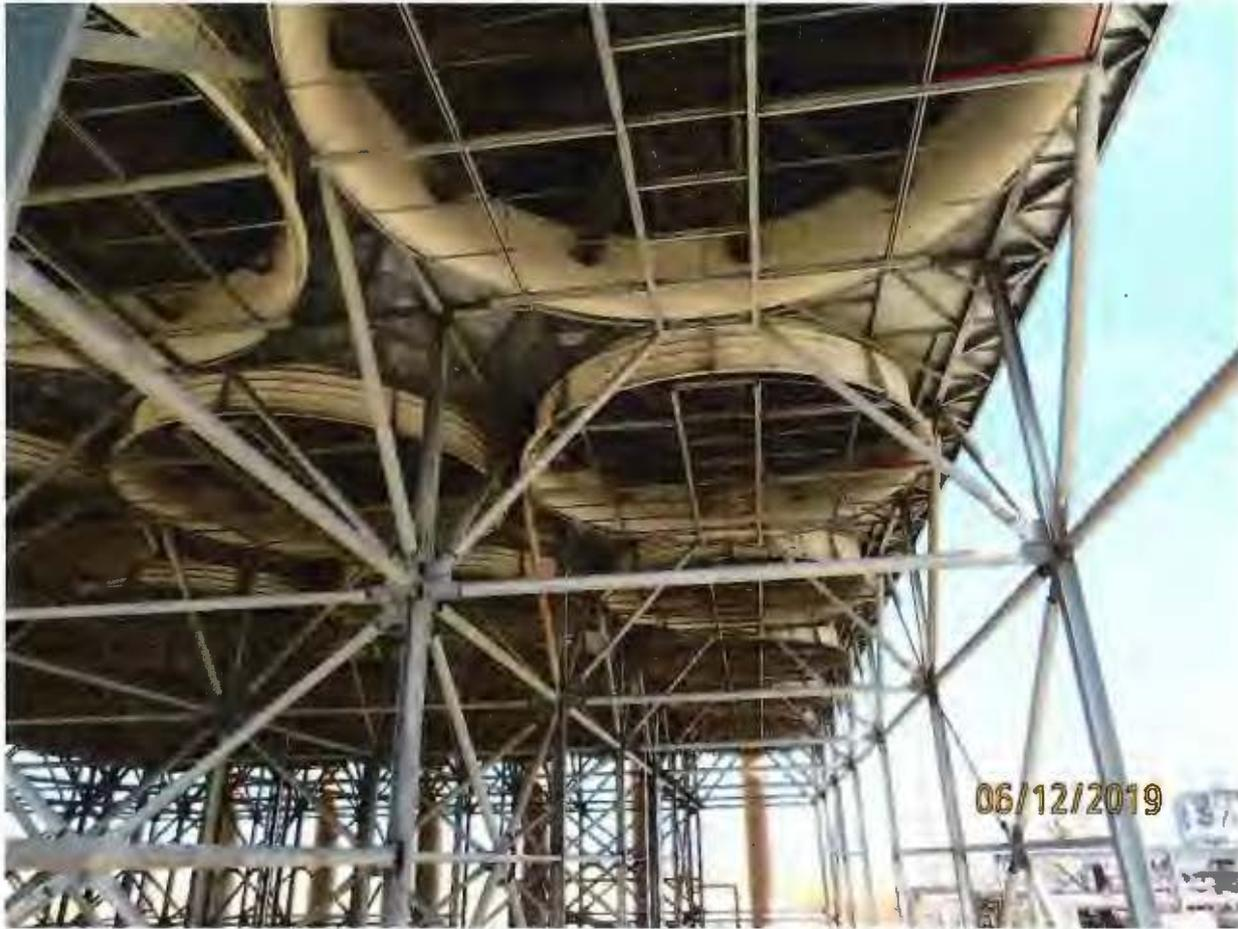
**Photograph 3: Closer view of fan and grate. Note gap between fan housing and grate**
