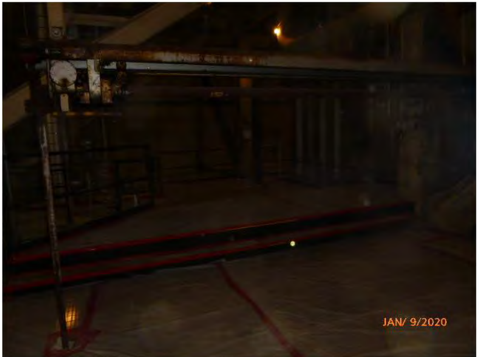
6. Flooring covered with poly reinforced sheeting adhesive taped joints & adhesive to floor.
