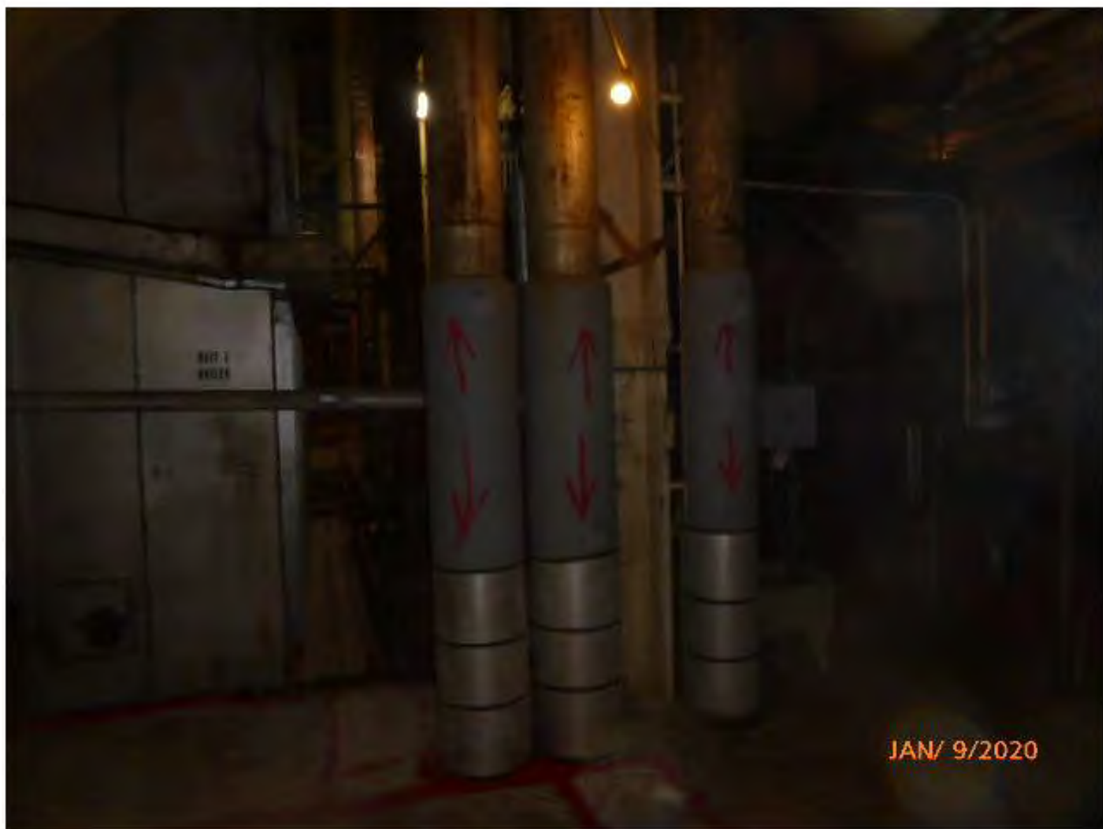
4. Identification of ACM (asbestos contained material) marking with Red Paint
