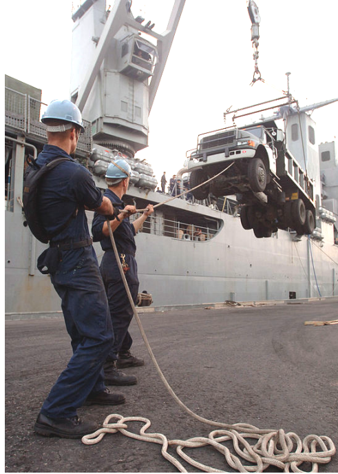
Figure 11: workers using tag-lines to guide the load during a lifting operation
