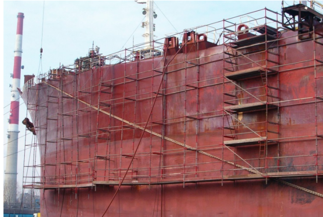
Figure 22: Cantilevered scaffold on a ship. Picture by Brosen, CC BY-SA 3.0
