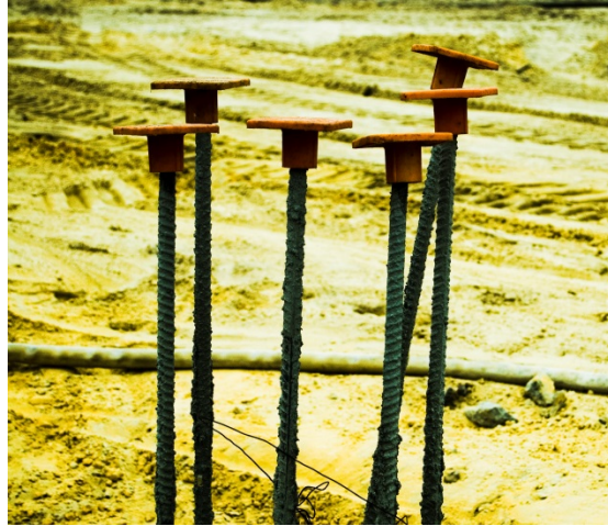
Figure 2: Protruding reinforcement steel with protective endcaps. Picture by Paul Goyette, CC-BY-SA-2.0
