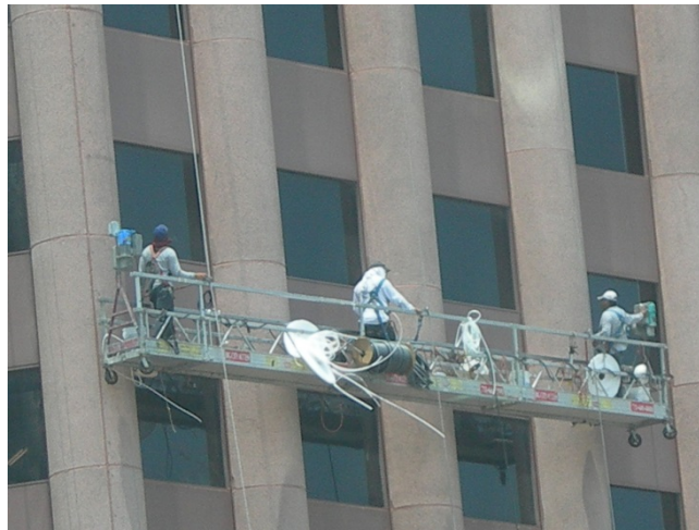
Figure 23: workers on a suspended scaffold. Picture by Hourick at en.wikipedia.org, CC BY-SA 3.0
