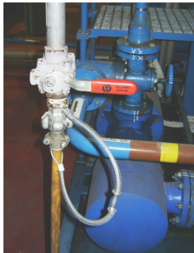
Figure 20: "Whip arrestor" fitted on a quick-release hydraulic piping coupling
