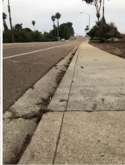
South Egress Sidewalk, Curb and Plants facing West along Cannon Road
