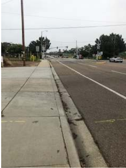
South Ingress/Egress Sidewalk, Curb, Driveway and Plants facing East along Cannon Road
