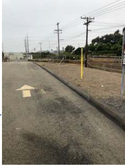
South Ingress/Egress facing Northeast, Curb, Gravel and Roadway
