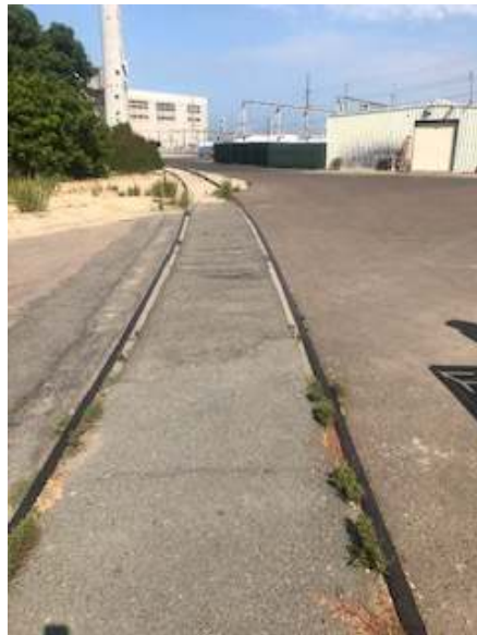
Railroad Tracks at Encina Gate Ingress/Egress facing West
