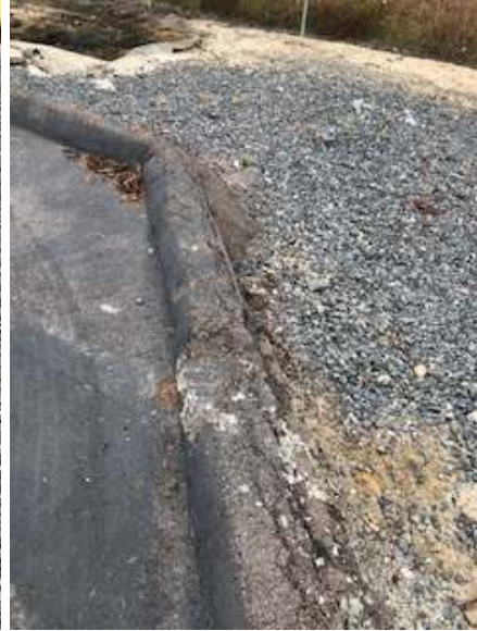
South Ingress Curbs, Gravel, Berm and Driveway facing Northeast
