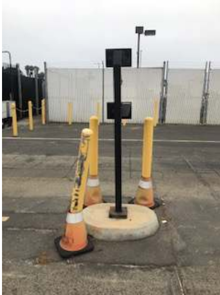
South Egress Card Reader facing West
