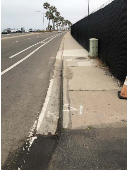
Berm, Curb, Sidewalk and Roadway Northeast Ingress facing North
