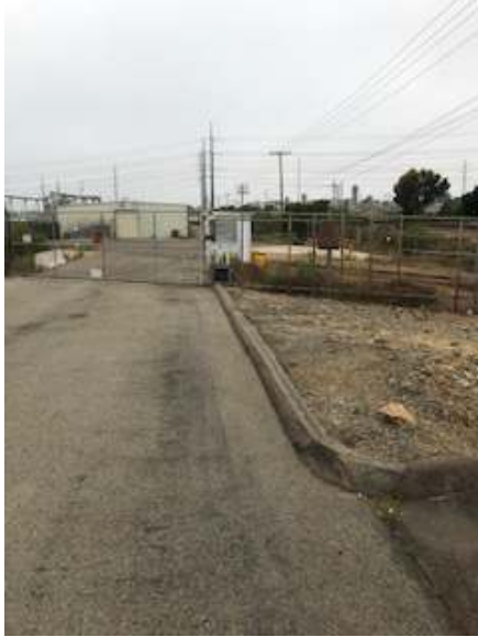
South Ingress/Egress facing North, Curb, Fencing/Gate and Roadway
