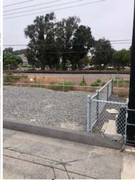
South Ingress Fencing, Curb, Driveway and Gravel
