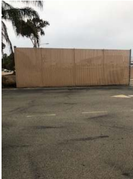
South Egress Fencing and Driveway facing West
