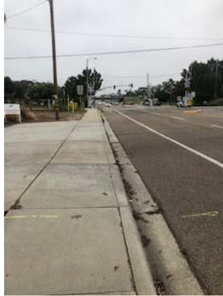
South Ingress/Egress Driveway, Sidewalk, Curb, facing East along Cannon Road
