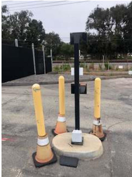
South Ingress Card Reader facing East
