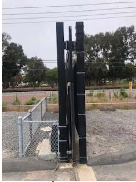
South Ingress Fencing, Curbs, Driveway and Gravel
