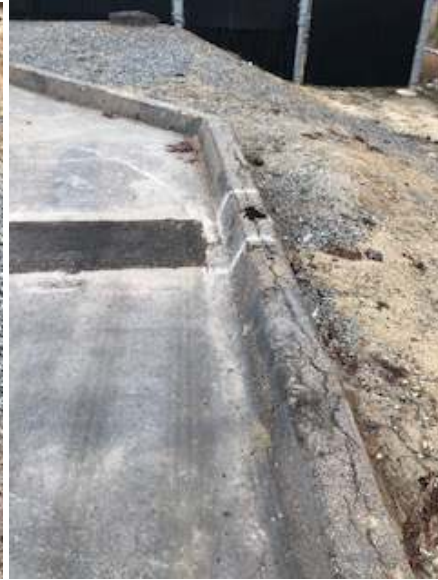
South Ingress Curb, Berm, Gravel and Driveway facing North
