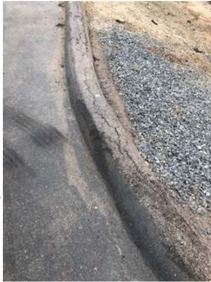
South Ingress Curb, Gravel, Berm and Driveway facing North
