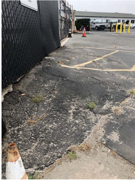
Northeast Berm at Ingress
