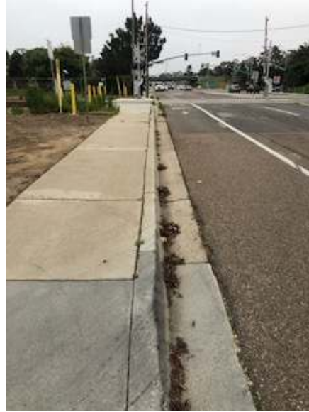
South Ingress/Egress Sidewalk, Curb, Plants and Sign facing East along Cannon Road
