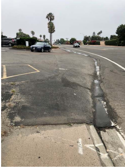
Sidewalk, Curb, Berm and Driveway at Northeast Ingress facing South
