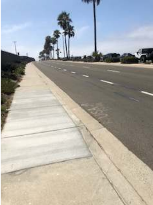
South Facing Ingress Driveway with Curb
