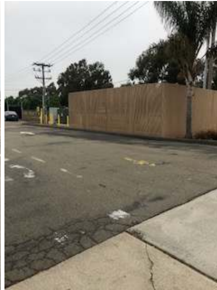
South Egress facing Northeast, Fencing, Bollards and Driveway
