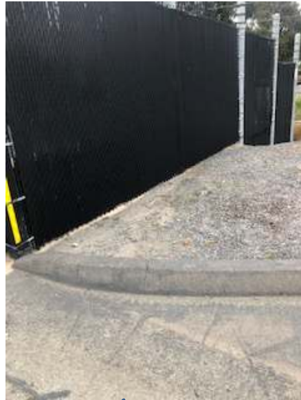
South Ingress Fencing, Curb, Driveway and Gravel
