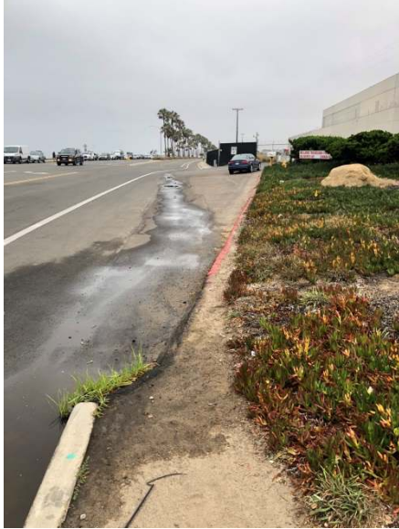
Curb, Roadway and Plants Northeast Ingress
