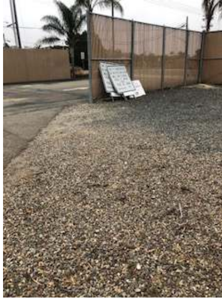
South Egress Fencing and Gravel facing Southeast
