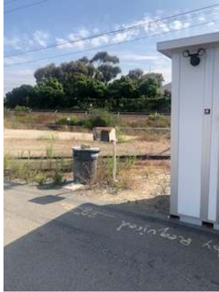
Encina Guard Shack, Card Reader and Roadway facing Northeast
