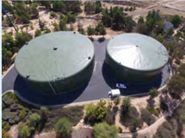
6 Million Gallons of Water Storage at RCWD. Source: RCWD
