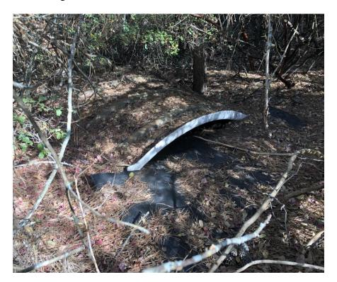
• The sedimentation pond outlet is dry and appears to be plugged.
