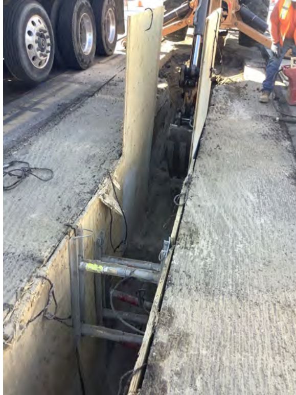
South, installing bracers after continuing trenching at 39+50
