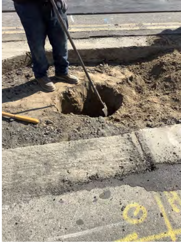
East, start of digging potholing at 48+30. Looking for sewer gas and water.
