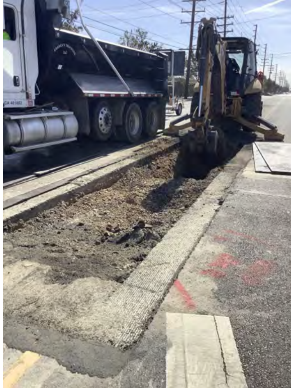
South. Start of excavation for exit of HDD at plant
