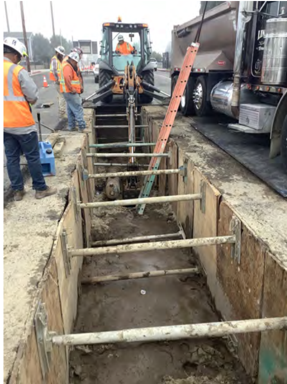
North, start of day cleaning out the HDD southern trench with the backhoe.
