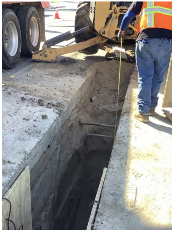
South, 46+40 2 inch gas and water lines crossing at 1 and 3 ft depth.
