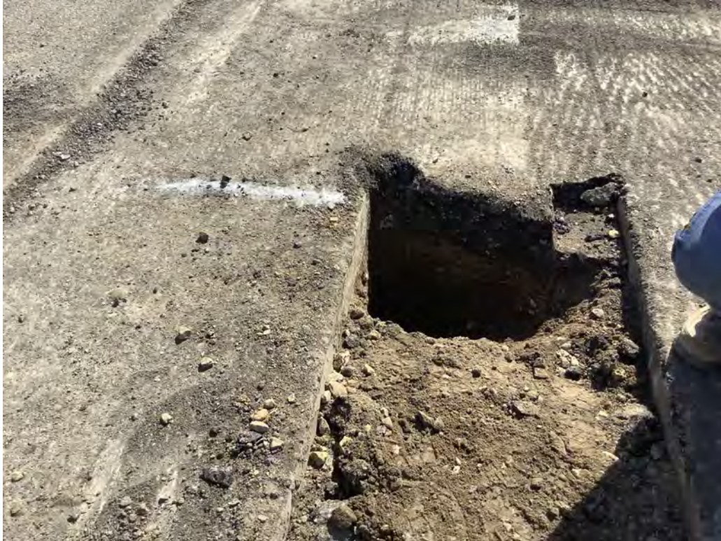
South, pothole (2 ft deep) at 64+75 where they were looking for signal electrical lines,
