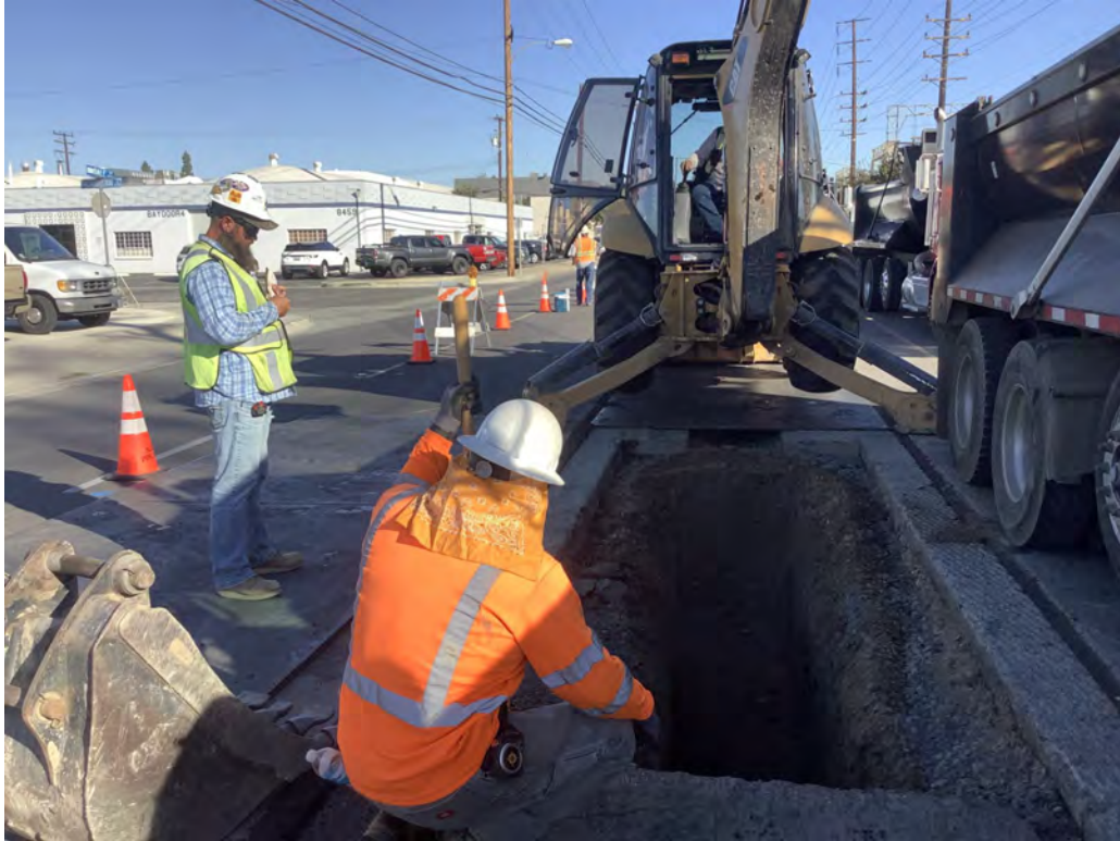
North, start of excavation for starting point to HDD under storm drain at Dale and STANDUSTRIAL ST.
