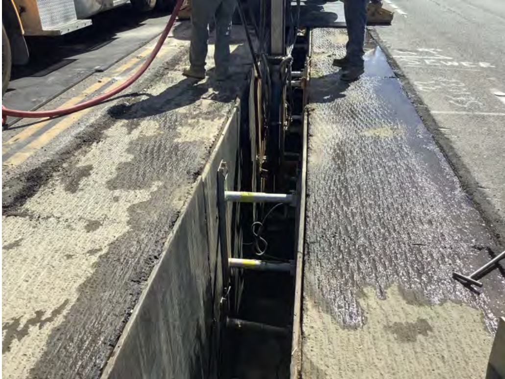
South, Steve 2 crew excavating around a Sewer pipe. Collapsing sand required wetting with water while digging (38+00).
