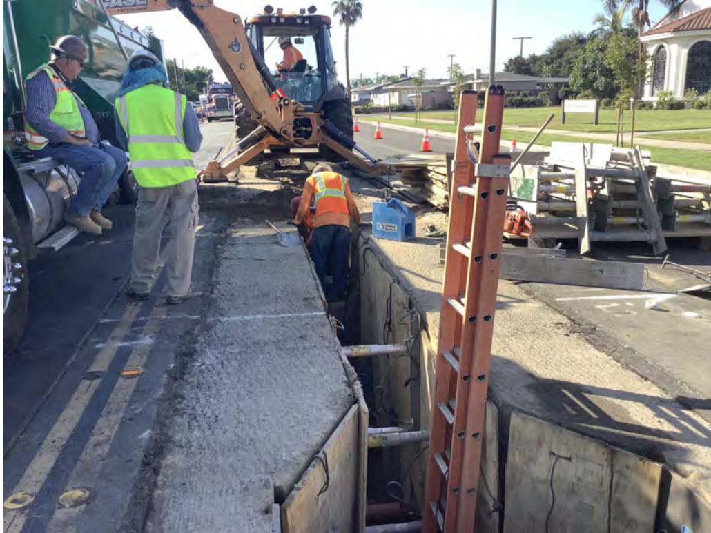
South, start of excavation process at 37+70. Laborers were hand digging around some electrical and wate pipes
