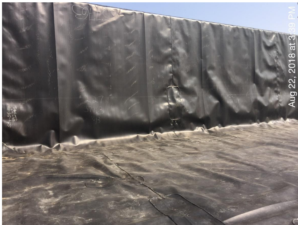
Detail of the secondary liner draped on the concrete wall
