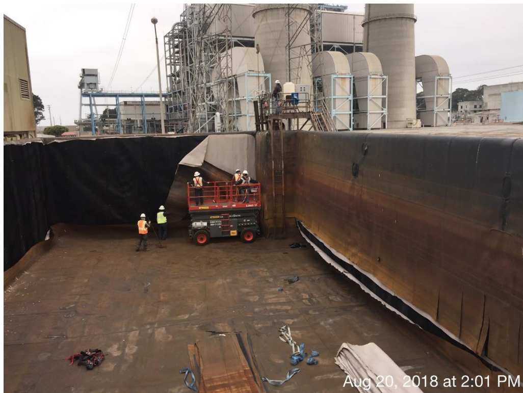
Larger piece of primary liner in the corner removed, it will be cut into smaller strip to be hauled out of the impoundment with the crane
