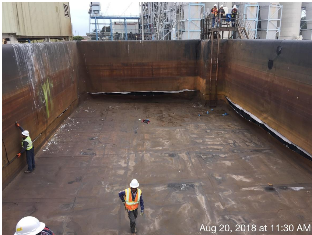
Bottom of the vertical primary liner was cut with hook blades and the liner crew gradually made vertical cuts to delineate what could be done from the bottom of MCWP No. 3
