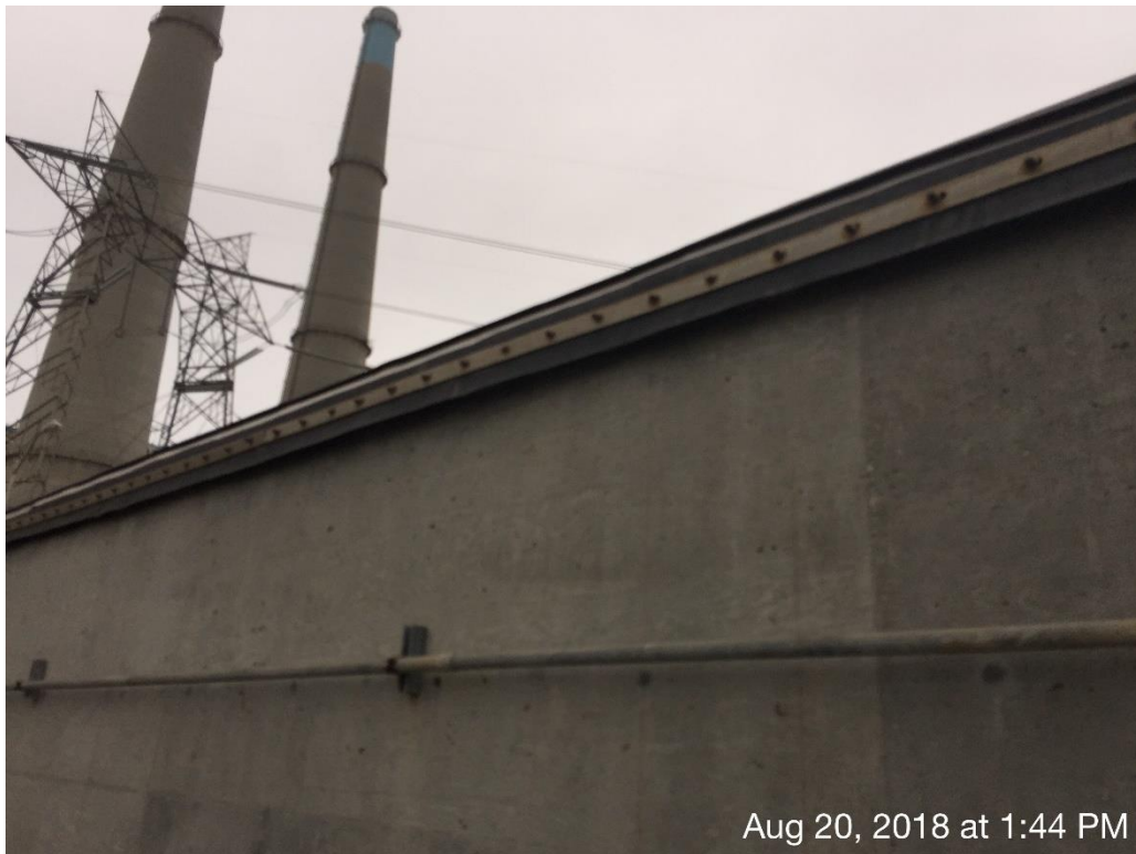
Detail of the batten strip, it was determined most optimal to leave the small little portion of primary liner in place and was used as a “washer” to hold the liner sandwich in place; otherwise the entire batten strip assembly would needed to be redone
