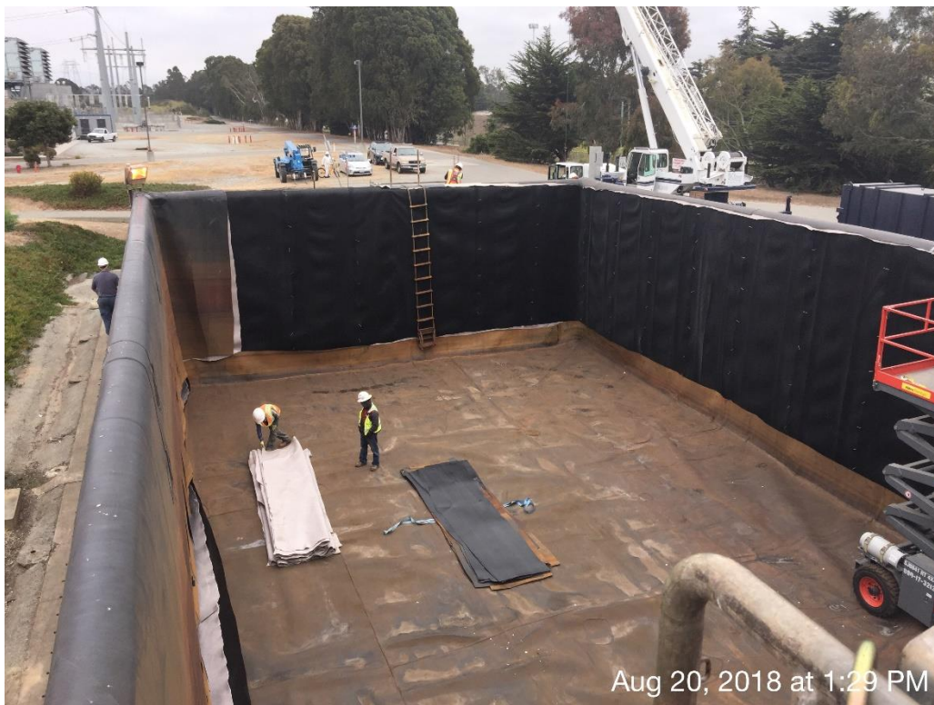
Liner crew making nice progress with the primary liner about ½ removed and the upper geotextile overlying the geonet as well
