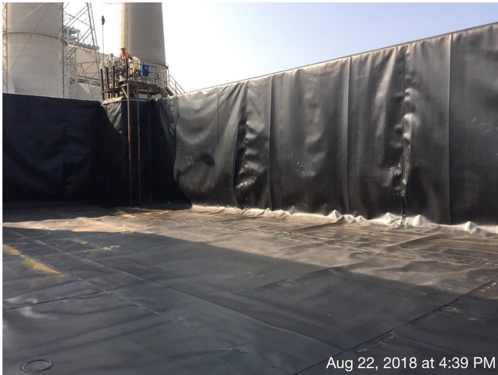
Detail of the MCWP No. 3 detailing the “secondary liner”, the original lining detail are still visible on the panels.
