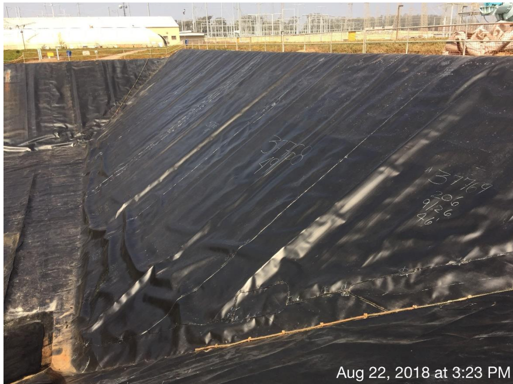
Different view into MCWP No. 2, original geomembrane roll listed, together with the length of the “panel”.
