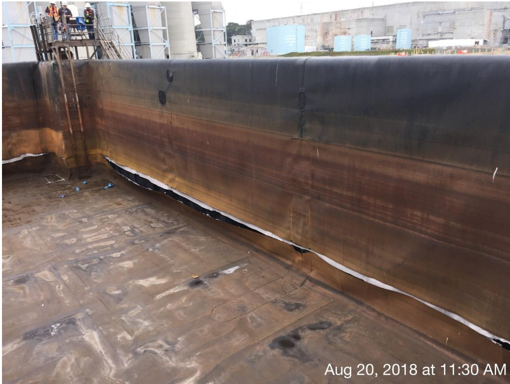
View towards the west, bottom cut made alongside the vertical walls
