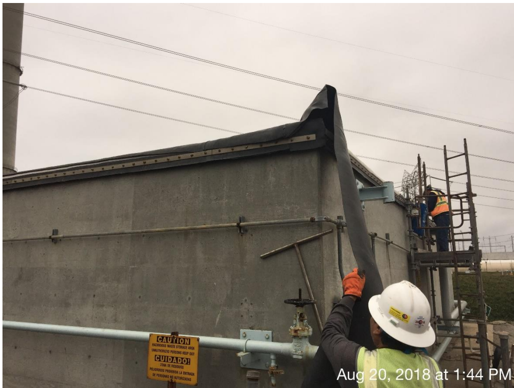
Removal of the primary liner from the top of the concrete walls
