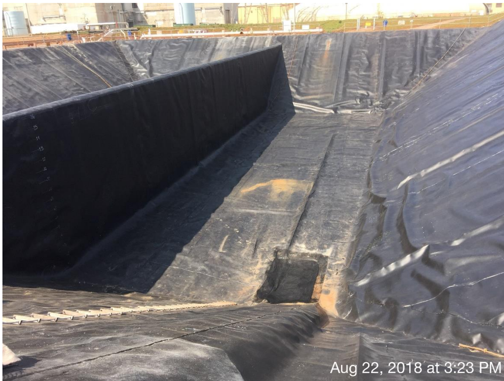
View into MCWP No.2, inspection of the “secondary liner (geomembrane). Since the primary liner was removed, this liner system now becomes a double lined system
