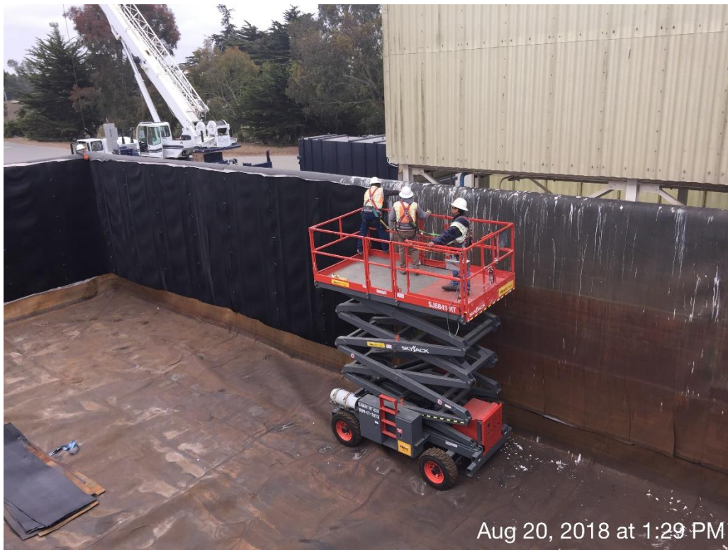
Boom lift used to make the vertical cuts in the primary liner
