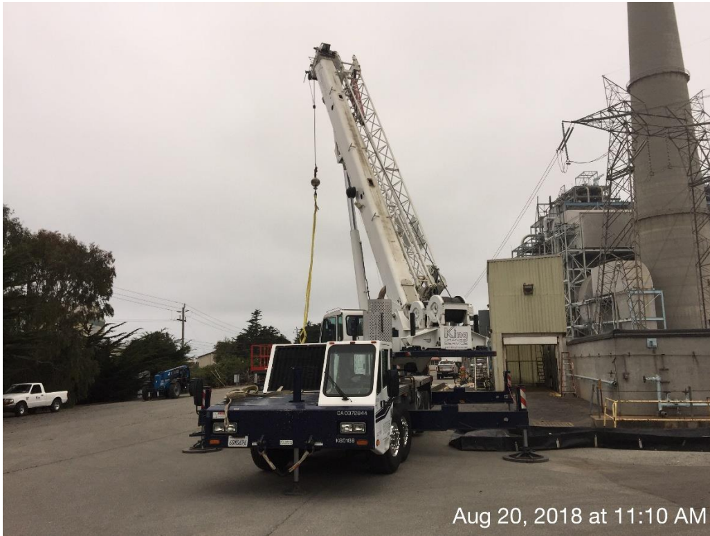
Crane is ready after weight checks to lift boom lift into the MCWP No.3
