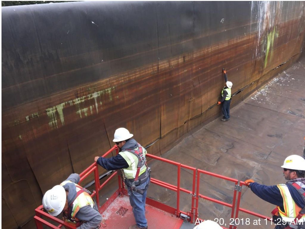
Liner crew from International Lining Technology started cutting “strips” with a hooked blade in the upper primary liner (geomembrane) as of not to damage the underlying secondary liner.
