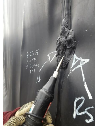
Photo showing the single repair made on the liner by placing a bead on it, the repair was checked by spark testing. The repair was successful
