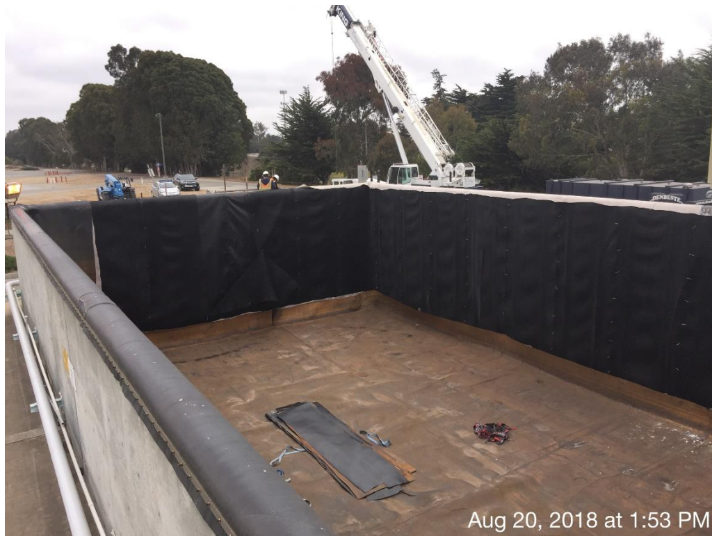
The geonet just started to be de-constructed as well on the eastern wall of the impoundment
