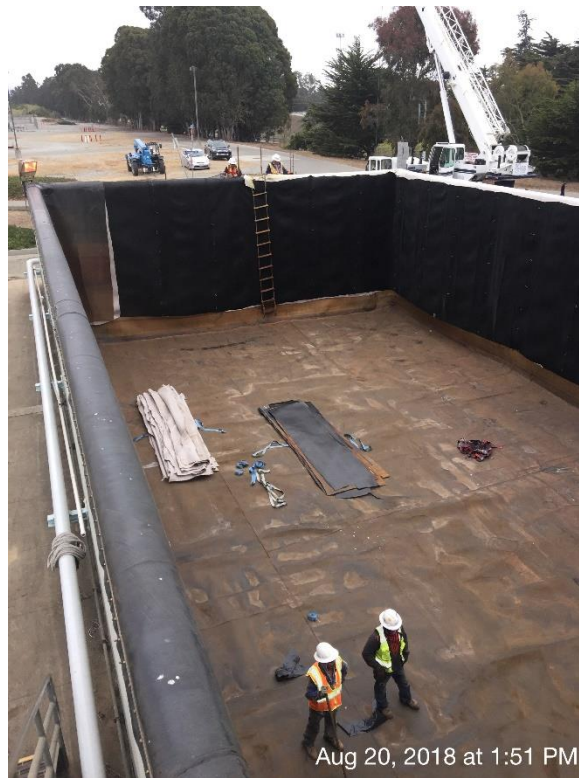
Major progress made so far today, the pieces/strips of geotextile and primary stacked in the middle of the impoundment
