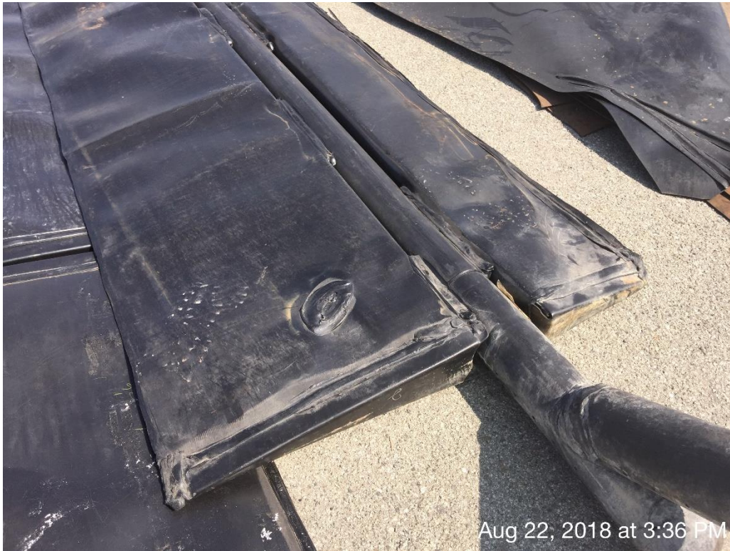
The pipe was sandwiched between 2 foam blocks to minimize the stress cracking of the liner surrounding the pipe
