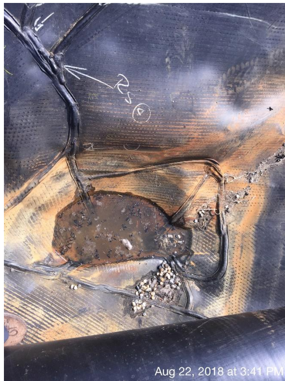
Detail of the sump area, minimal amount of water present to make the observations, a sacrificial piece of liner will be placed above it and a sump pump placed to evacuate the surface water that accumulate into the lined area
