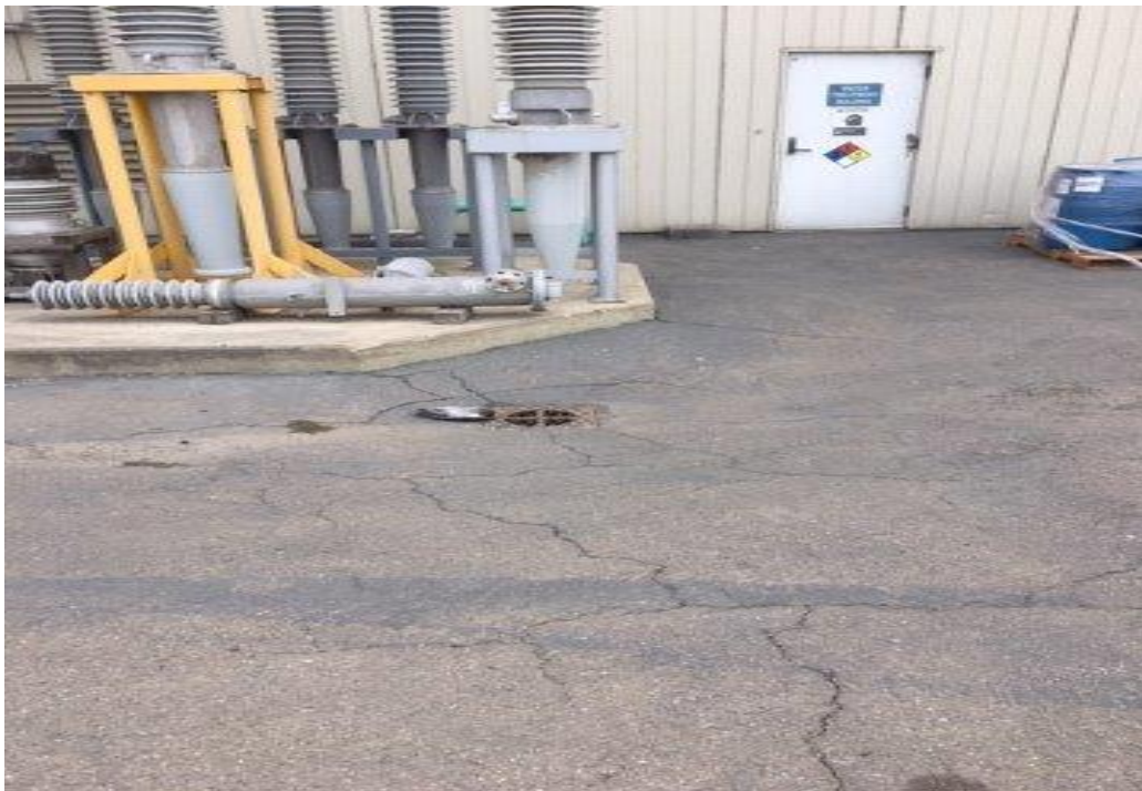
Photo 16. Dead pigeon carcass as observed by LEC personnel on north side of STIG water treatment building. November 13, 2018.
