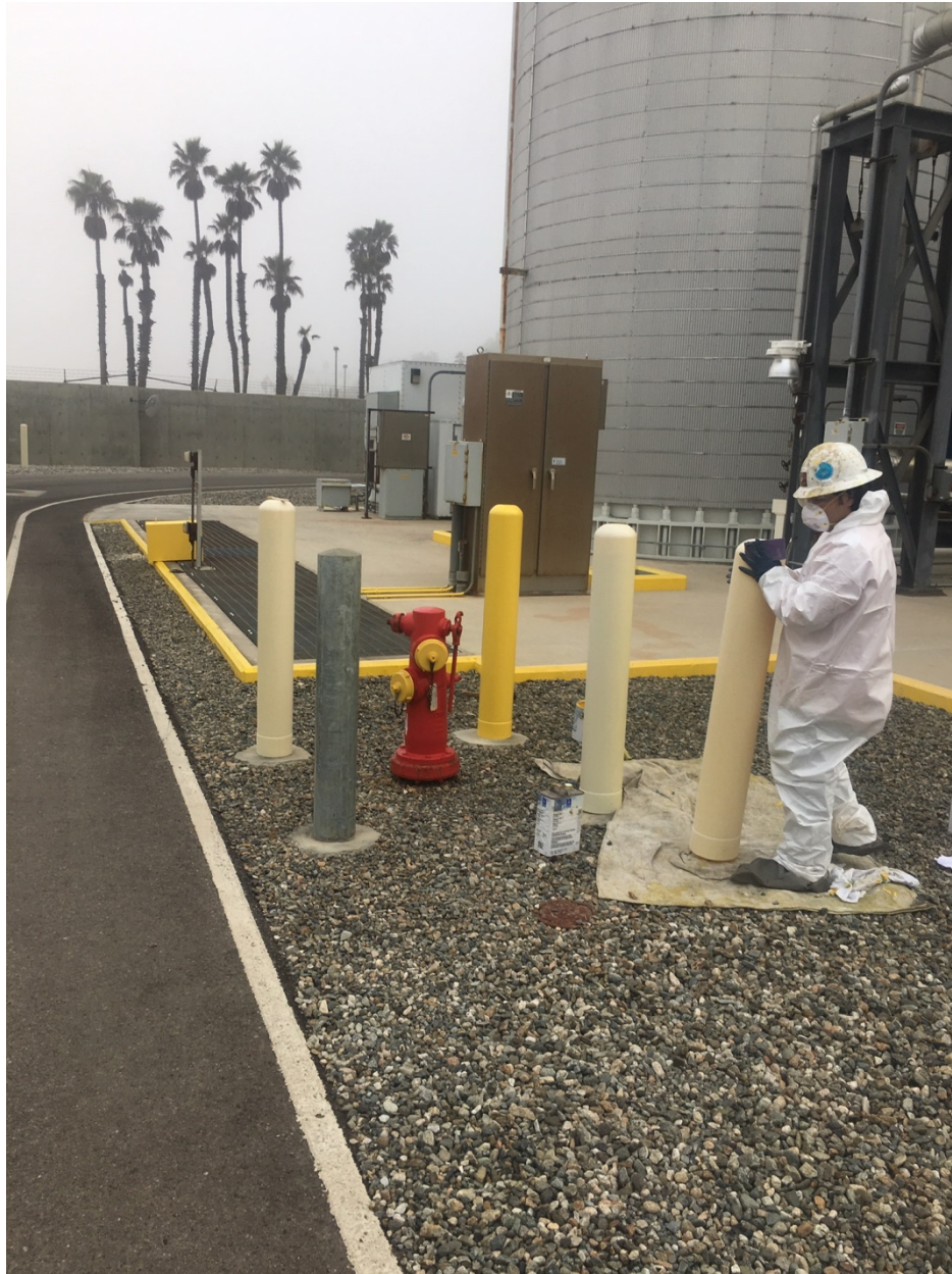
Bollards reconditioned and repainted
