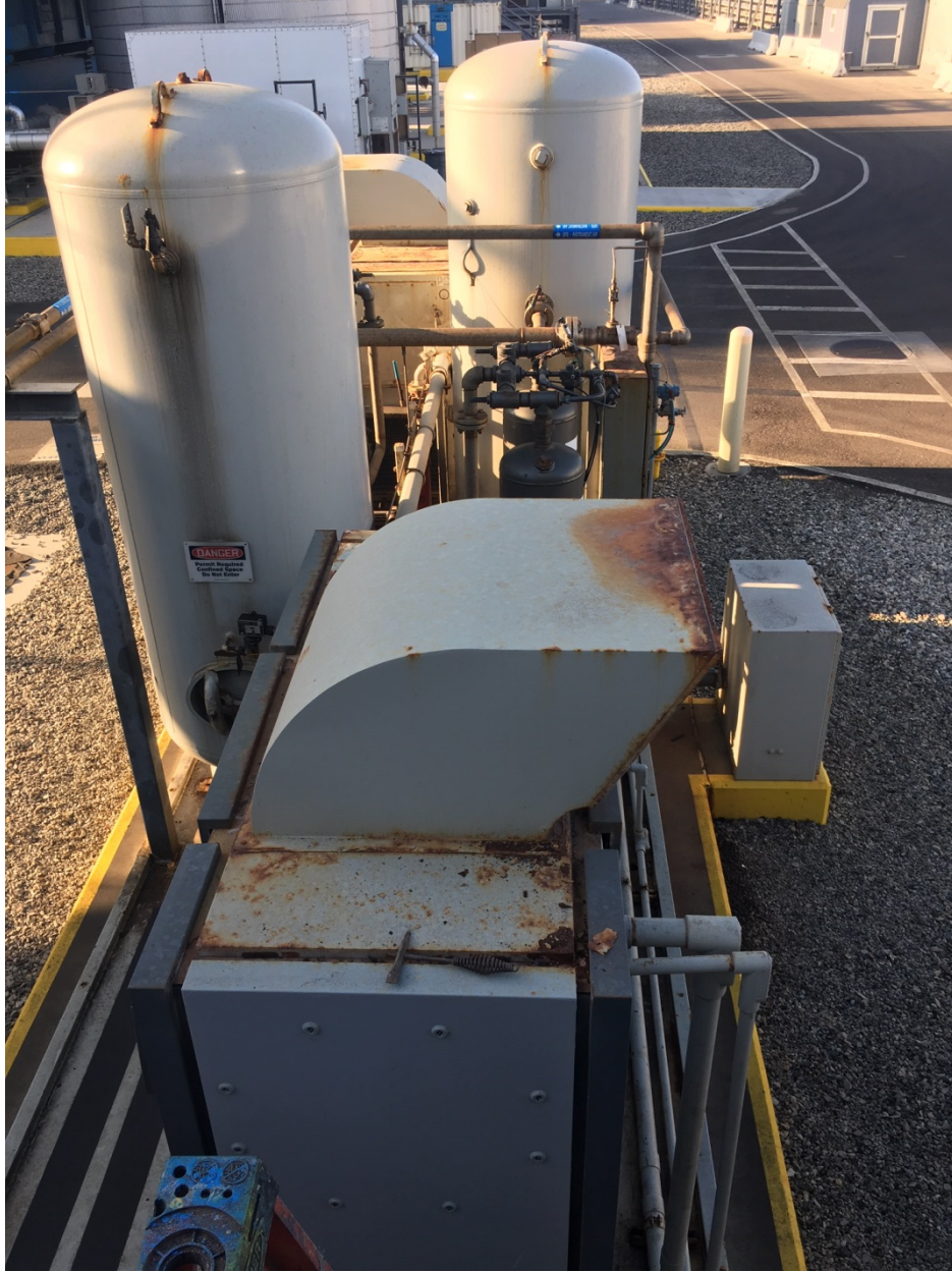
Air Compressor System prior to repainting
