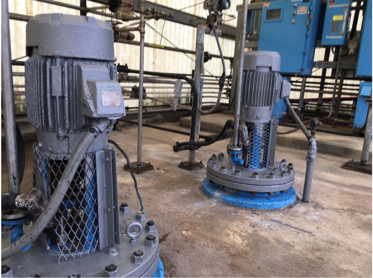
Ammonia Forwarding Pumps prior to repainting
