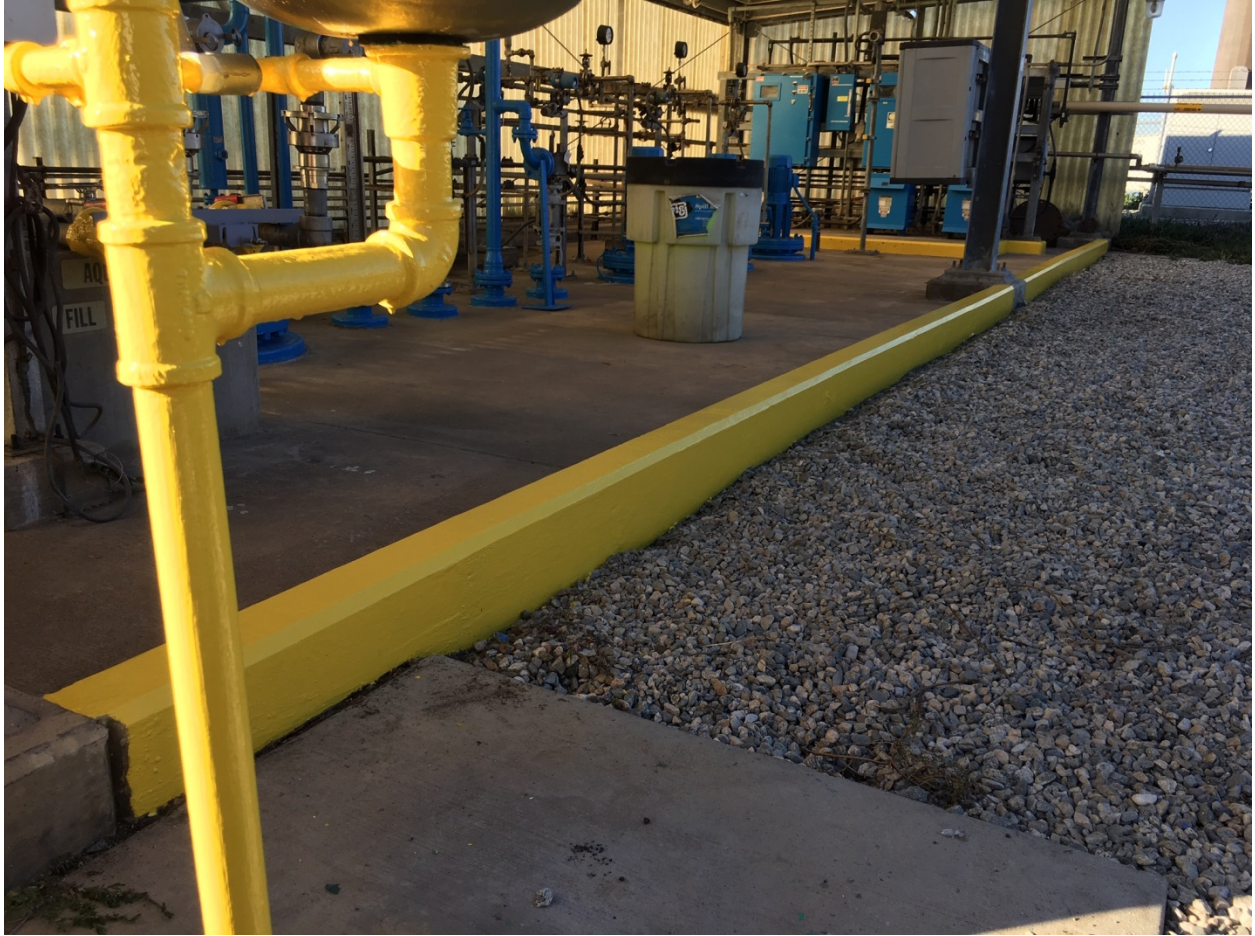
Curbing for Ammonia Tank System repainted
