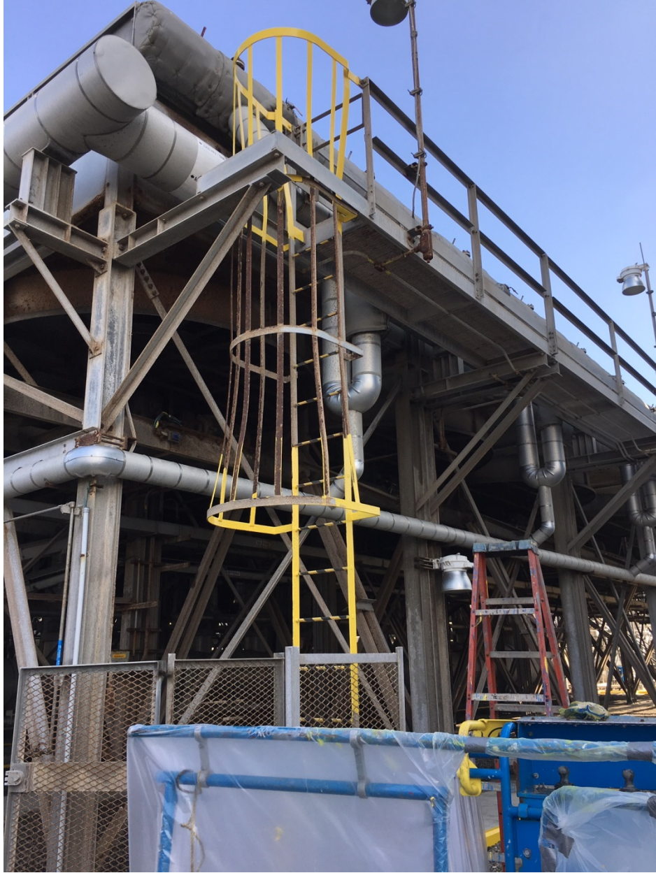
Ladder(s) sanded and repainted
