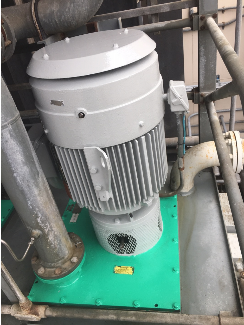
Forwarding Pump repainted
