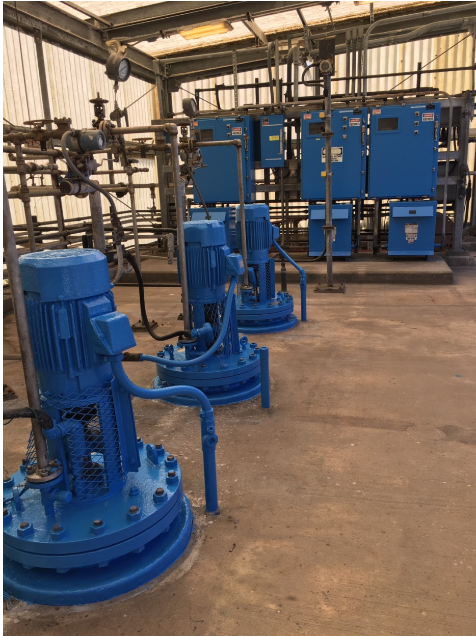
Ammonia Forwarding Pumps repainted
