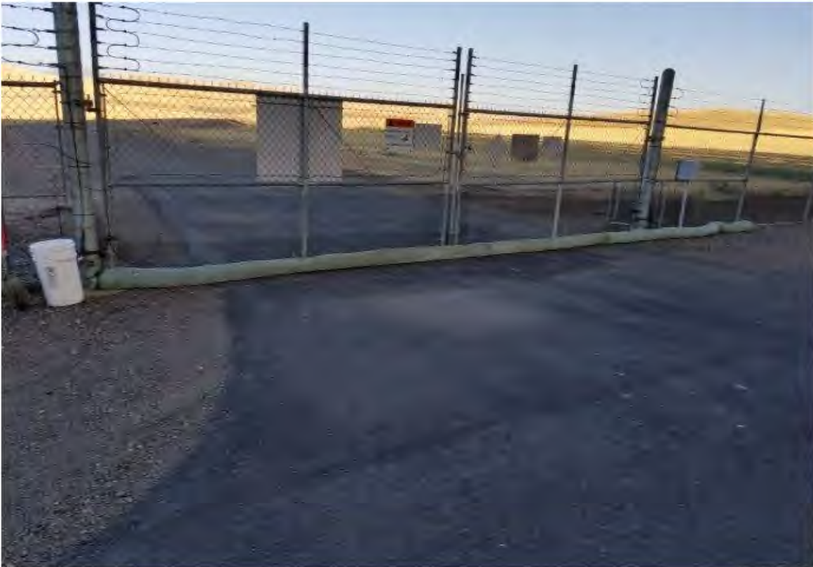
Photo 36, of fiber core roll placed at bottom of back gate to help keep snakes out, 6/14/18.
