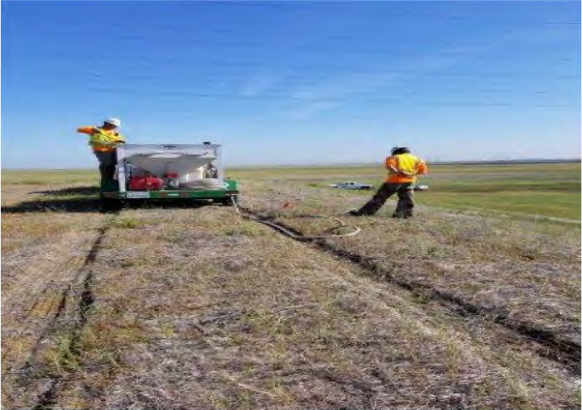
Photo 13, of Sierra Weed Control backfilling erosion area with sand slurry, 5/3/18.
