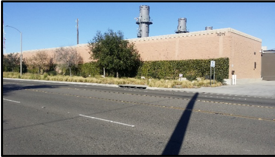
Miraloma Avenue, south wall
