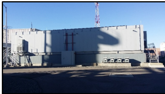
Main Electrical Enclosure Building (1/24/19)
