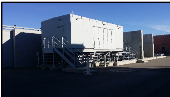
Balance of Plant Building (1/24/19)
