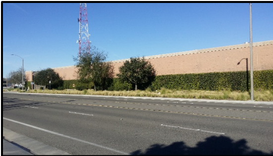
Miraloma Avenue, south wall
