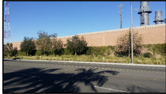
Miraloma Avenue, south wall
