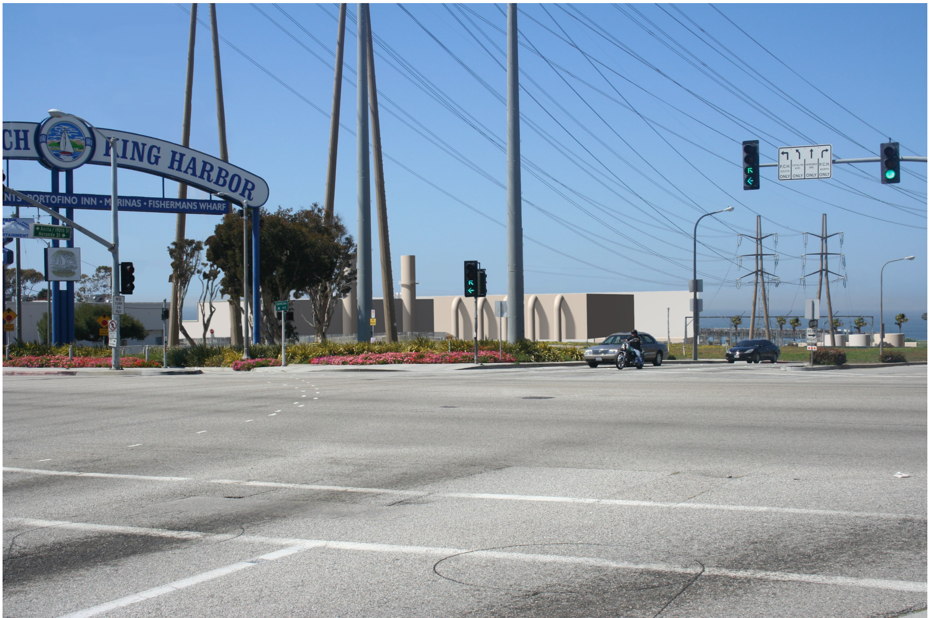
B. View from KOP 4 with the RBEP constructed and RBGS removed. The new Air-Cooled Condenser would be the most prominently visible RBEP feature.
