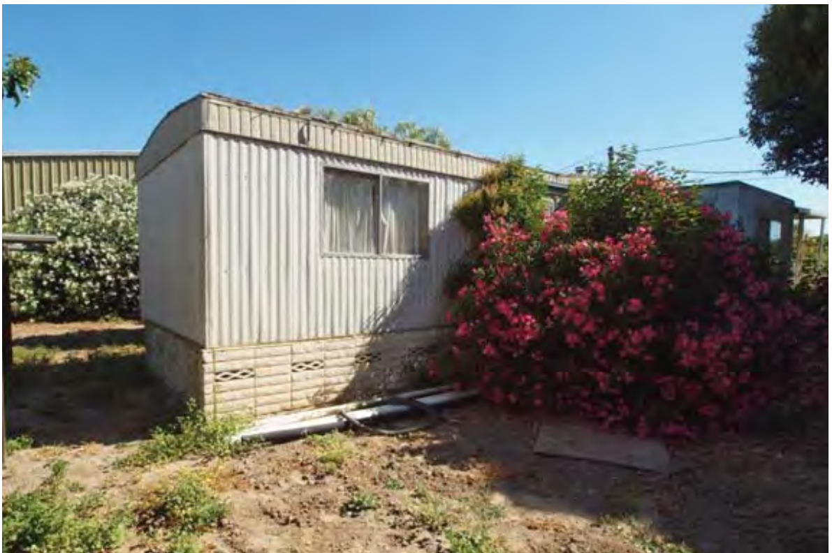
PHOTO 6: View of the prefabricated house within the farm complex, looking west from the main house.
