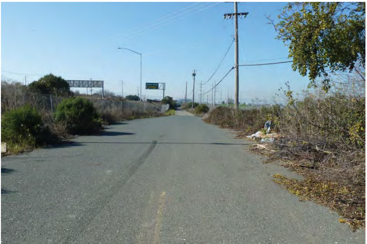
PHOTO 10: Alviso – Milpitas Road, looking west along the southern boundary of the site. SR 237 is located on the left side of the photo.
