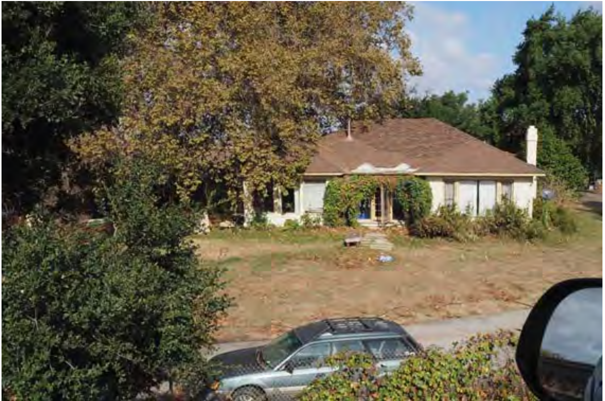
PHOTO 3: View of existing Edgar A. Jackson house in the southeastern corner of the site, looking north from Alviso-Milpitas Road.
