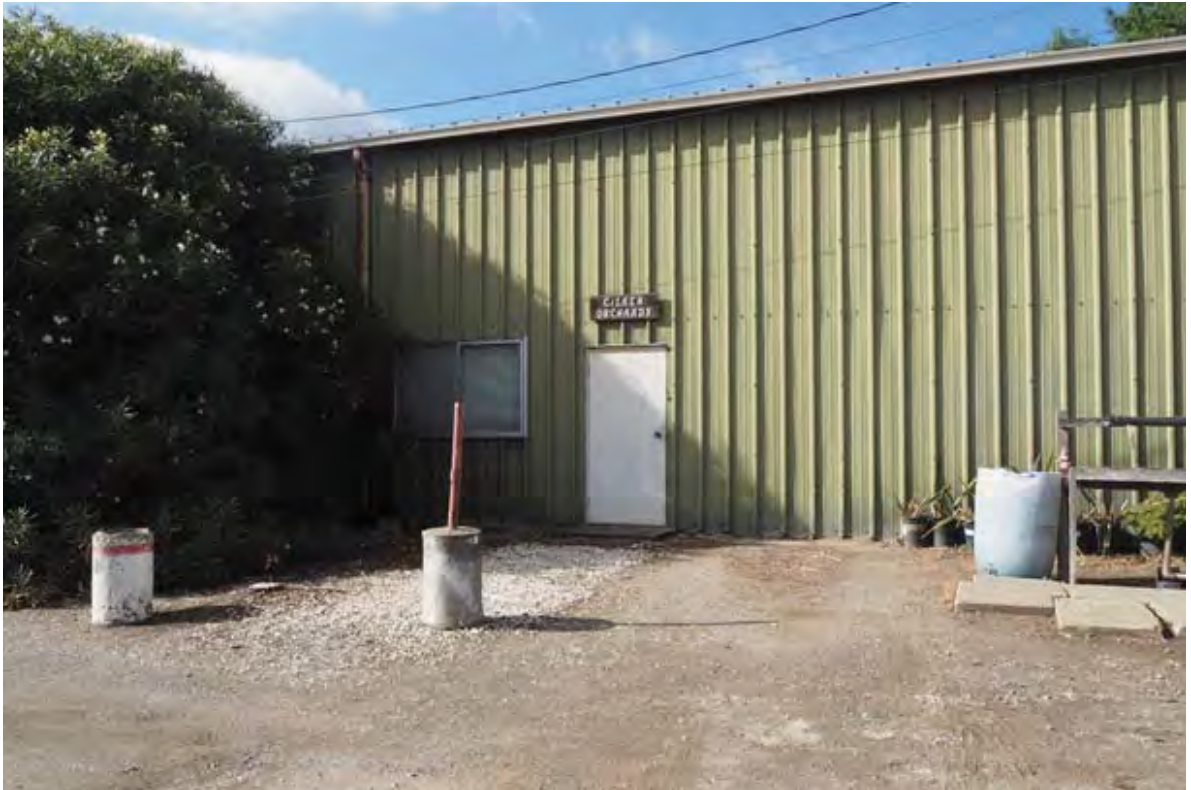
PHOTO 7: View of an accessory structure looking west, from the paved pathway.
