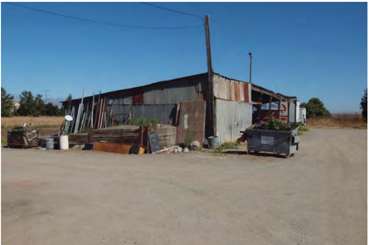
PHOTO 8: View of farm complex structure on the project site, looking northwest from the paved pathway.
