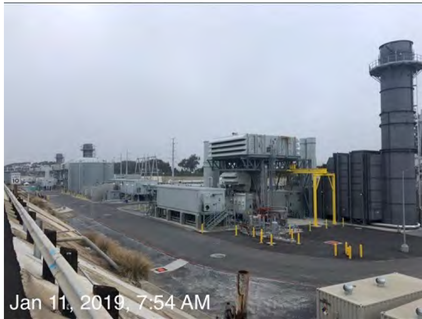
Photo 1: NRG construction is in the final stages of completion. Photo taken 1/11/19, facing northeast.
