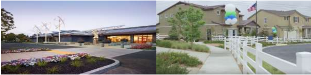
Figure 25. The Zero Net Energy Training Center (left) and the Zero Net Energy Meritage Homes (right)
