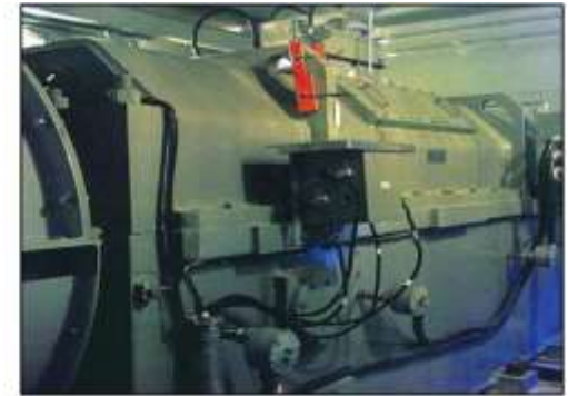
130 MW rated Encased Clutch installed in LMS100.
