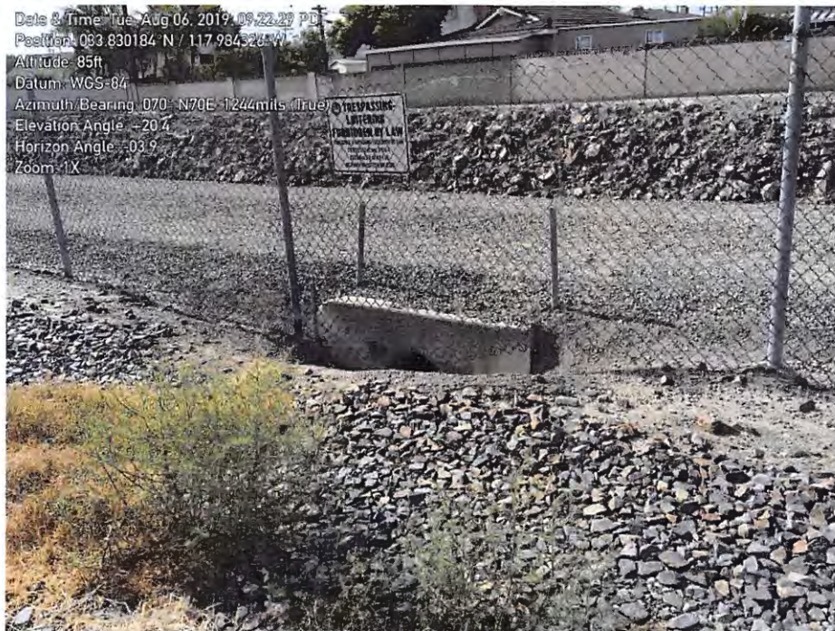
Photo 4. View southwest from the south-central portion of the proposed Carbon Creek Laydown Yard at a drain leading from the parcel into Carbon Creek.
