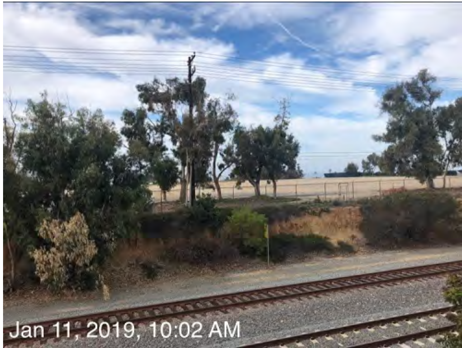
Photo 9. Construction has been completed in the West Laydown Area. Photo taken 1/11/19, facing west.
