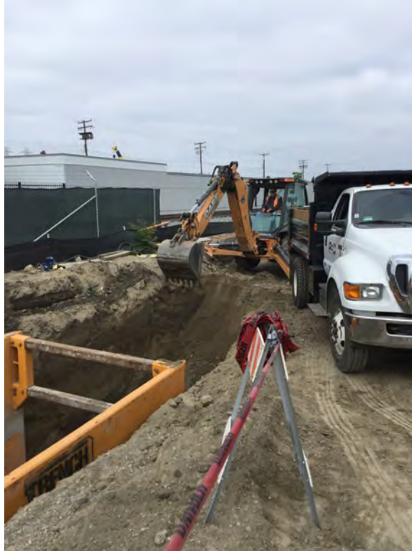
Excavation in parcel 1 66kv Duct bank
