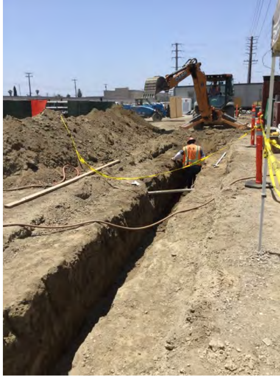
Fire protection line running west, close to ARB trailers
