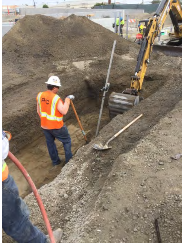
Excavation of a duct bank lateral off of the 66kv, going north
