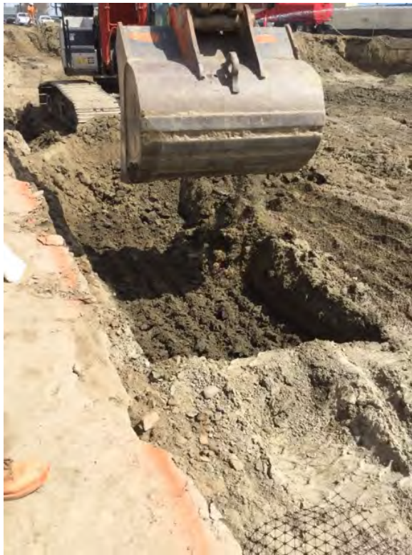
Ortiz taking the entire grade down another foot into the sandy clay unit
