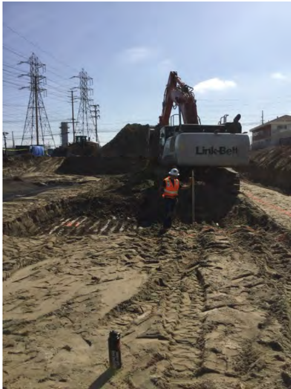
Excavation for 480V Auxiliary transformer depth ~EL61'
