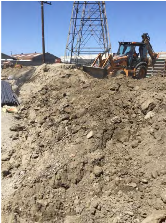
ARB excavating a mound in parcel 2 down to grade
