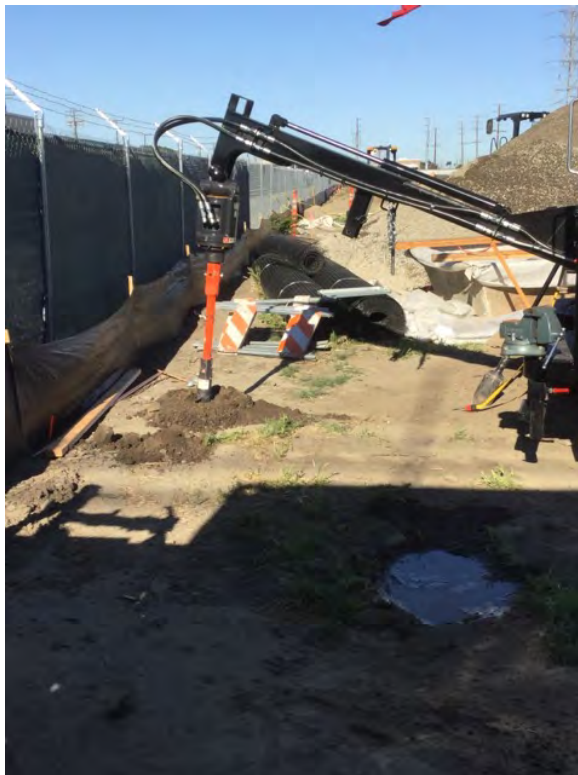
Auger used to drill 4' depth for temp pole installation
