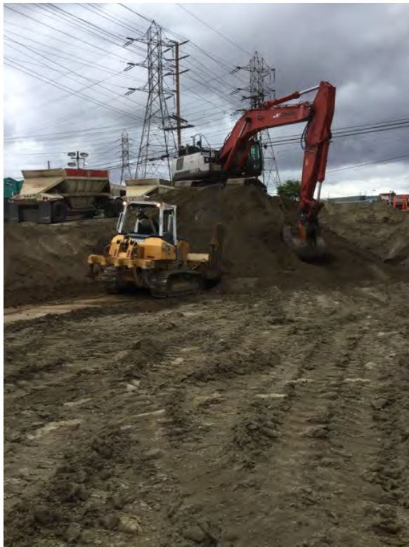
Excavator and dozer used for mass excavation
