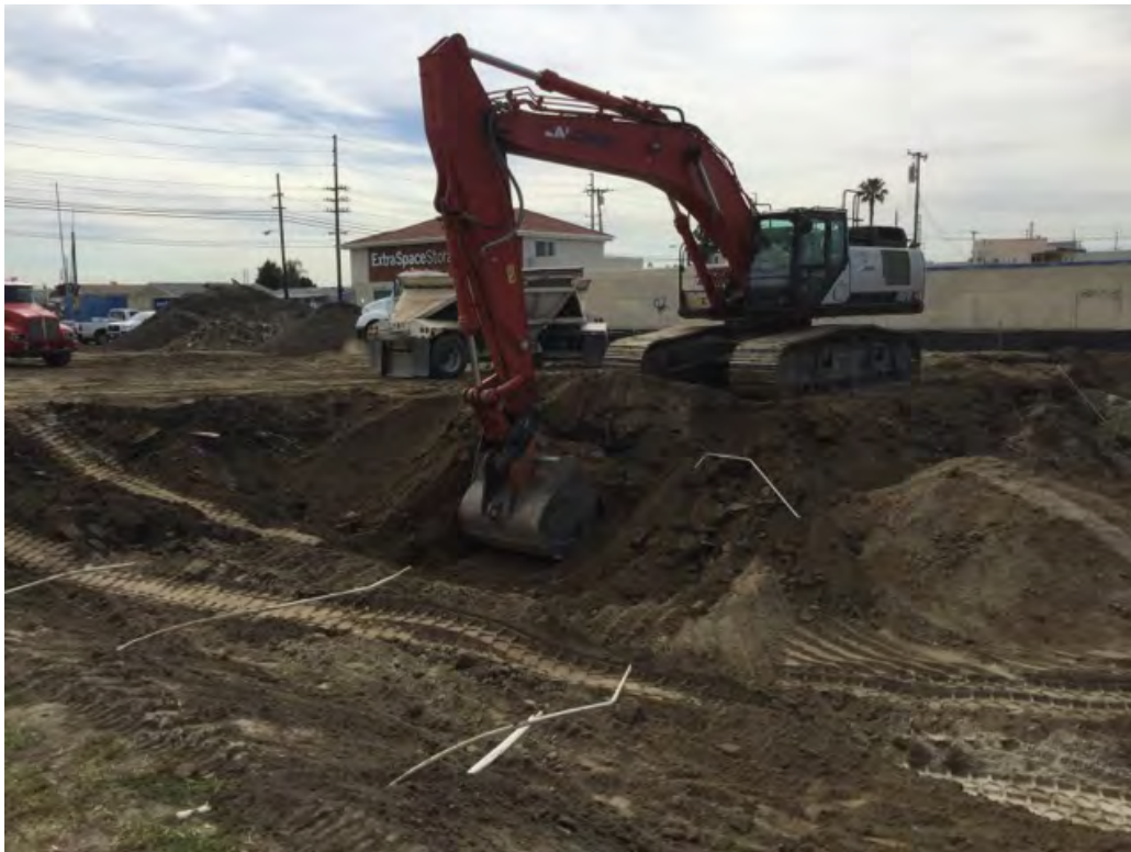
Excavator used during overex of parcel 1
