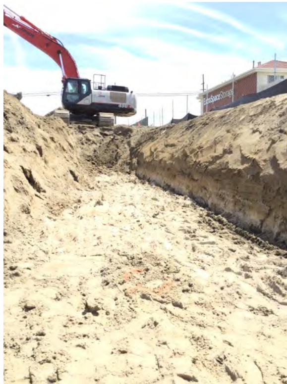
Excavator lowering the cut further down to EL~63, close to the south east corner of parcel 1
