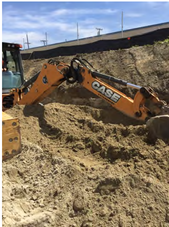
ARB churning up sediment for conduit trench in order for it to dry out.
