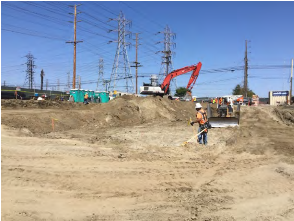
Excavator and dozer used for mass excavation
