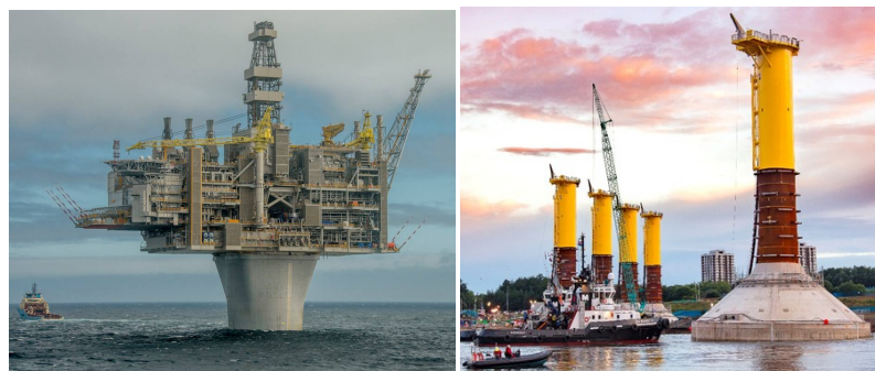
Figure 2. Concrete's durability offshore has been demonstrated in numerous oil and gas applications (left) and wind turbine gravity-base foundations (right).
